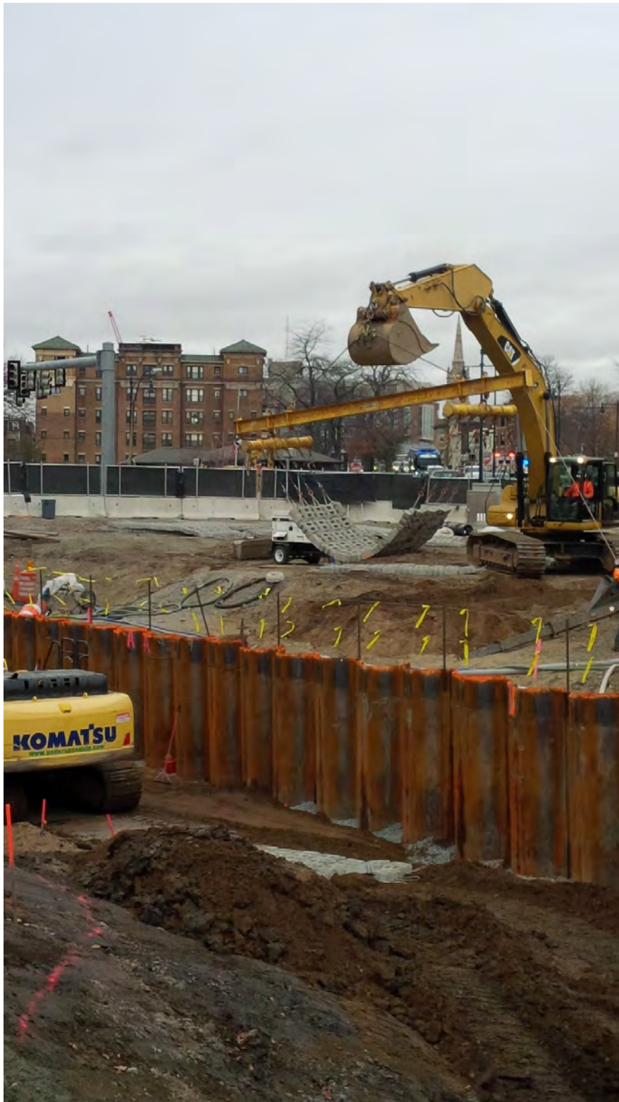
Equipment lowering sections of Articulated Concrete Blocks (ACBs) in place for scour protection downstream of the new Riverway Culvert – mid November 2015.
