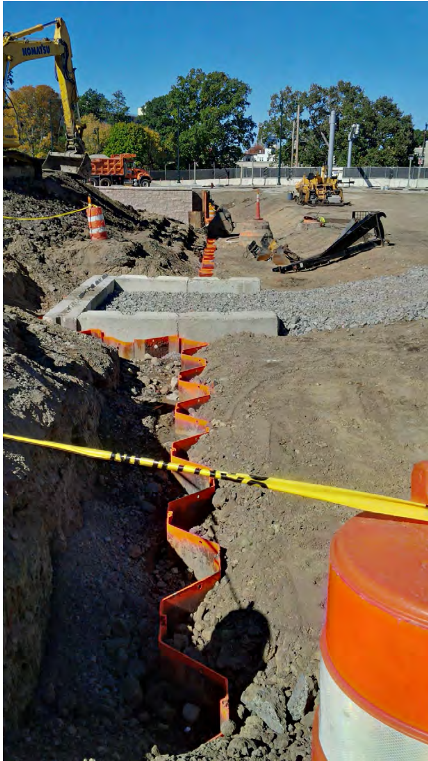
Steel sheeting installed for the river diversion in the pre-excavated trench in the former Sears Parking Lot – note the box-out for the existing storm drainage system – mid October 2015.
