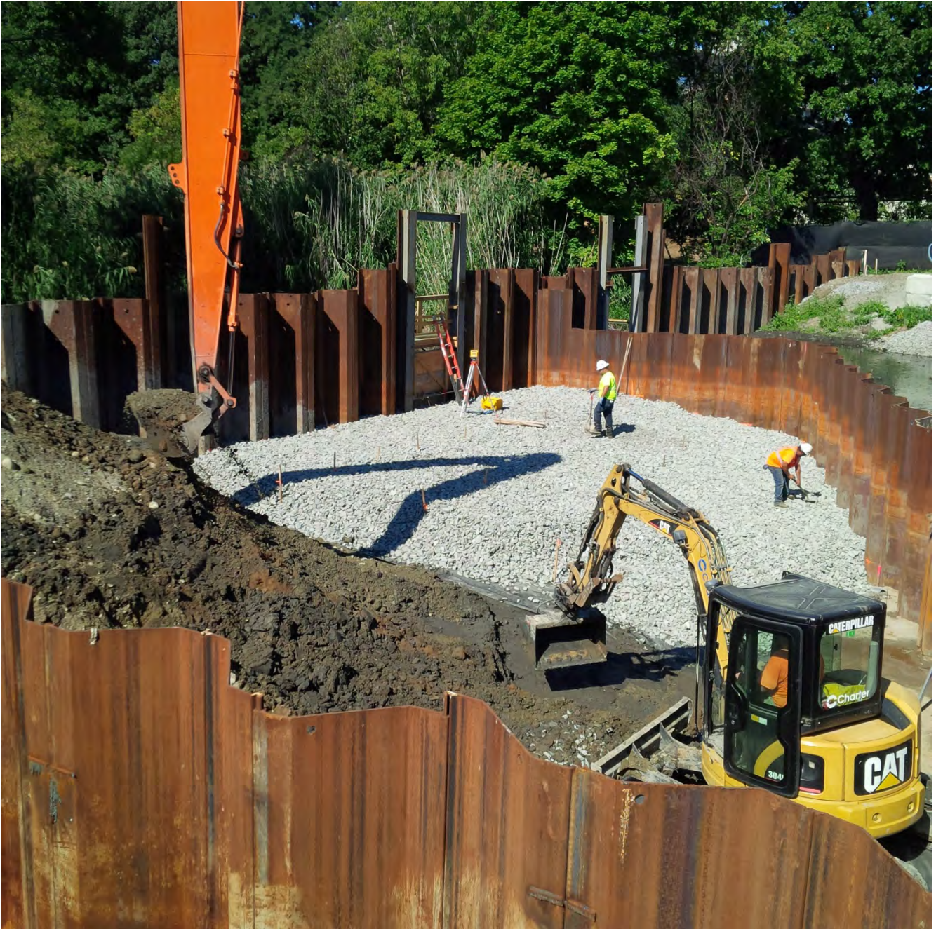
Grading and excavating of the flood risk management (FRM) channel on the southside downstream of the FRCS – mid September 2015.
