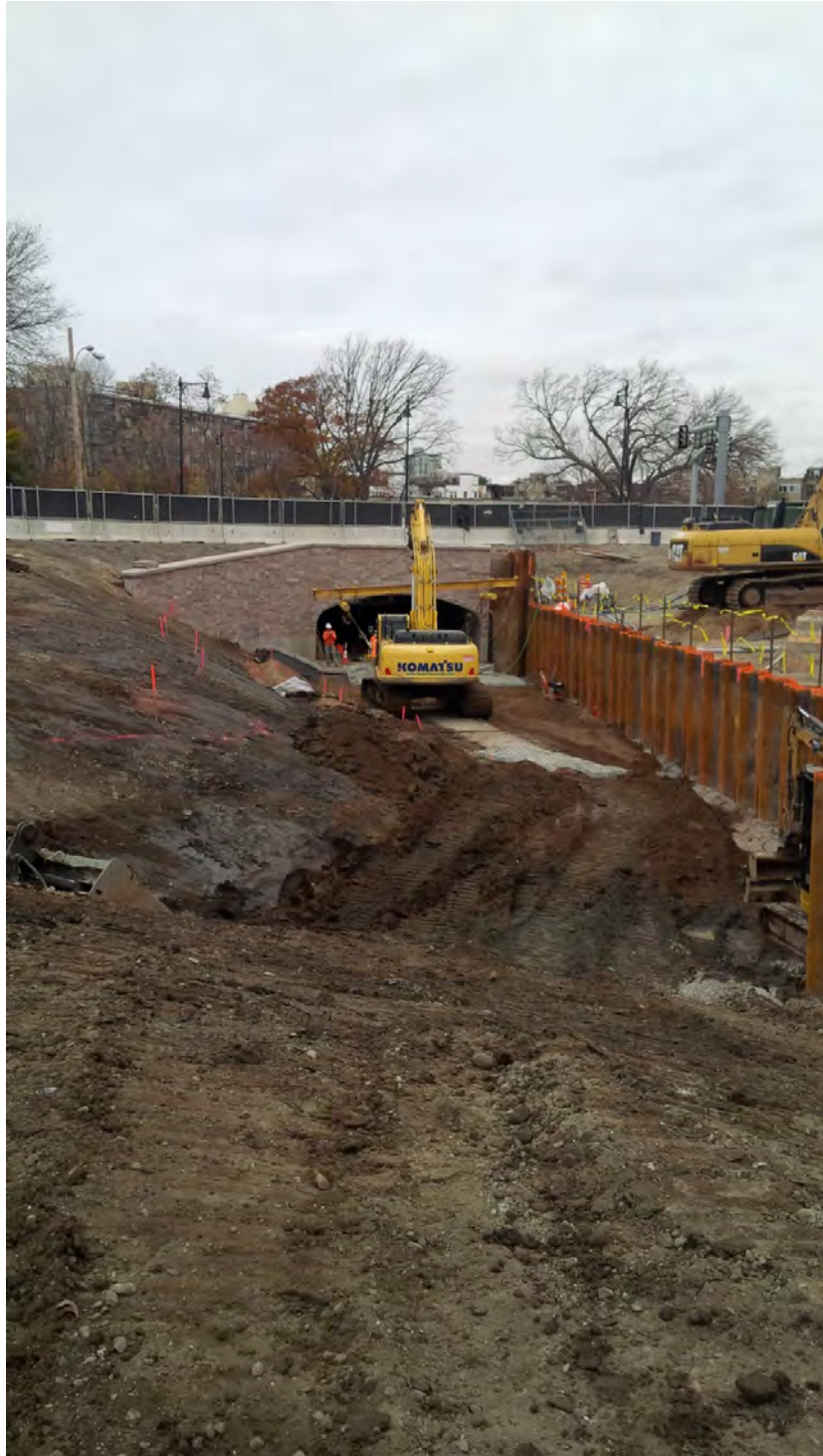
Excavation and shaping of the right (looking downstream) bank of the new river channel downstream of the new Riverway Culvert – mid November 2015.
