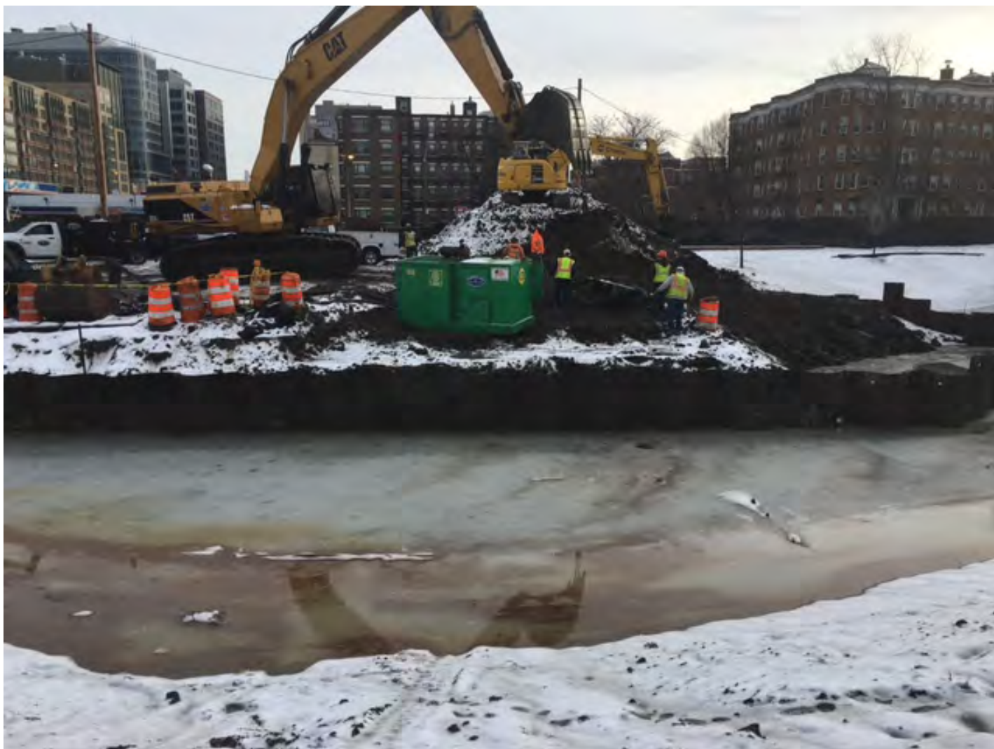
Former Jug Handle area – note the river flowing on the nearside in the new FRM channel; while excavation takes place on the far side – February 16, 2016.
