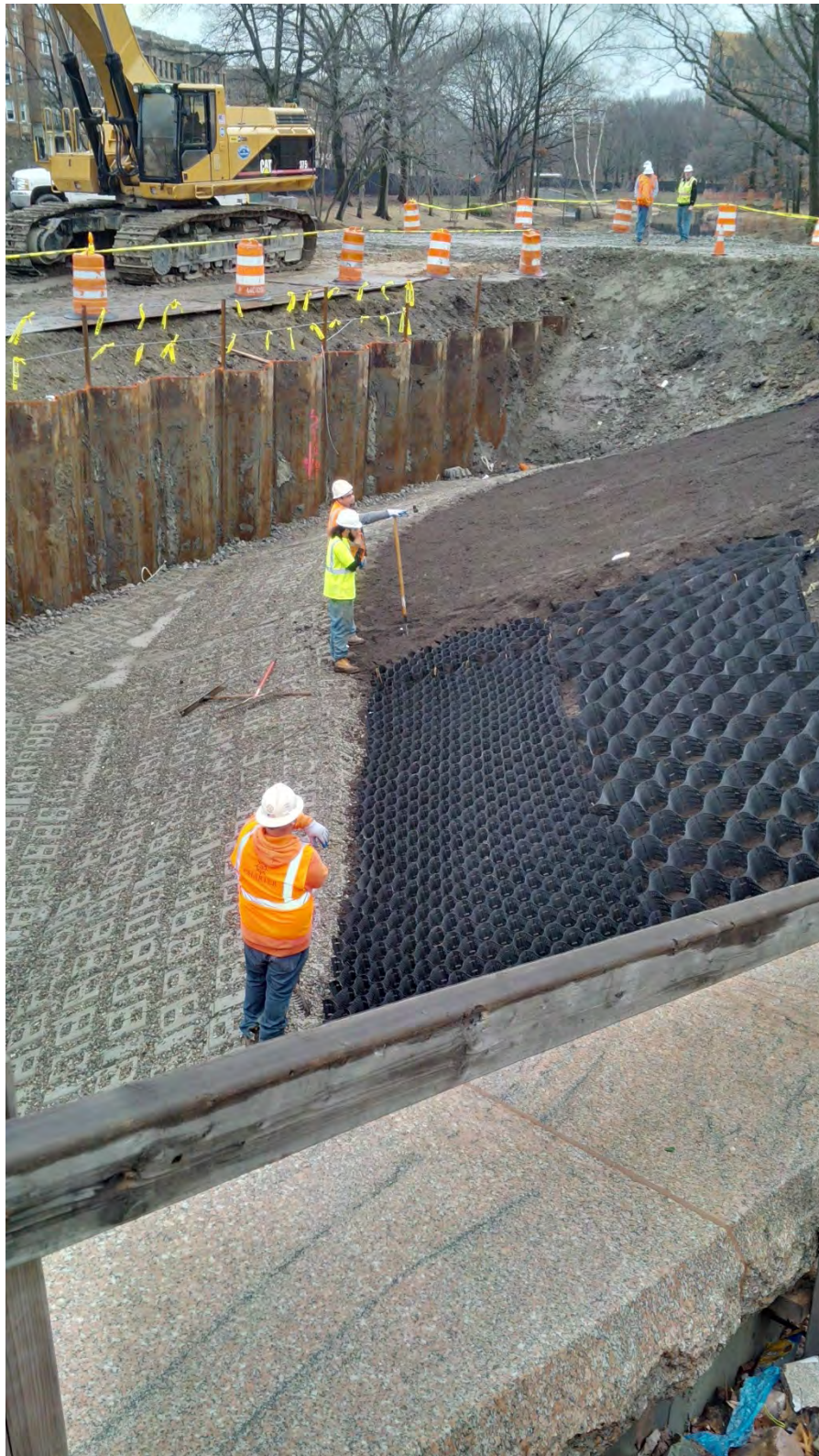
Installation of geocells and loam for bank restoration – downstream of the new Brookline Avenue culvert – early February 2016.
