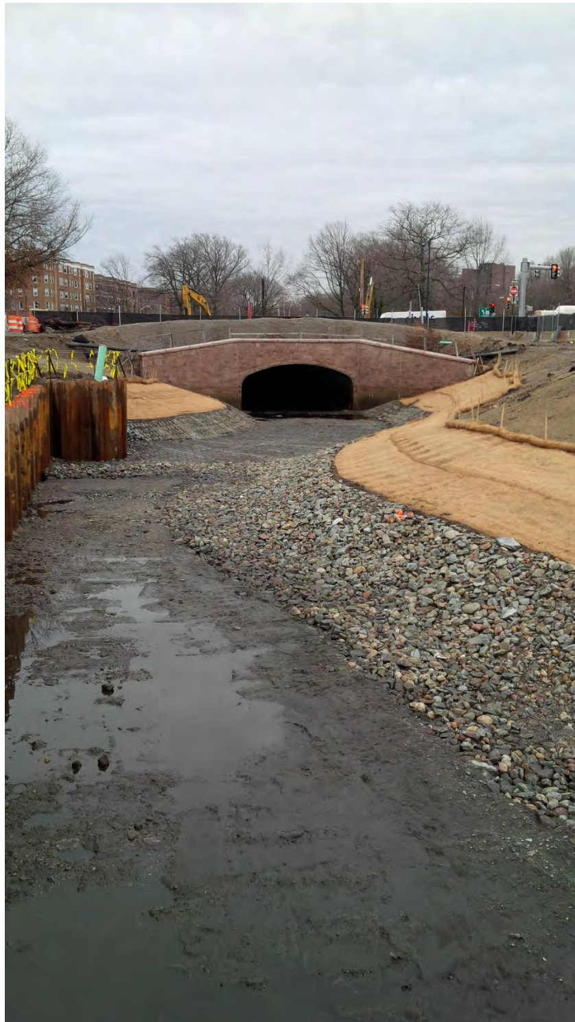
Southside of the flood risk management completed, to include ACB's for channel scour protection, and stone protection, geocells, and turf reinforcement mattress for bank protection – looking at the upstream Brookline Avenue culvert – early February 2016.
