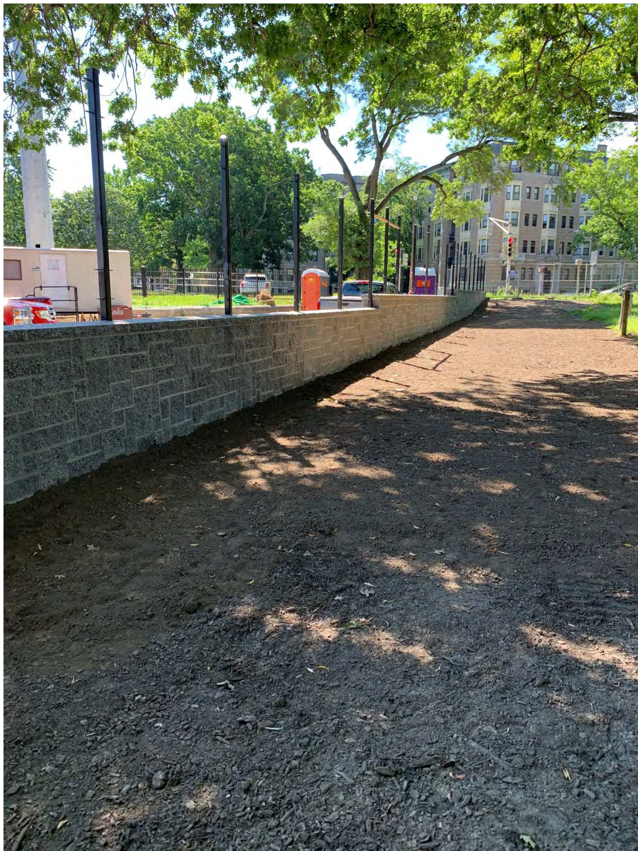
Work Area #13 – Boston Fire Department Building in the vicinity of the Fenway and Agassiz Road – granite veneer and capstone installed. Site backfilled at the south section of the constructed floodwall. Note the security fence post installed on top of the floodwall.
