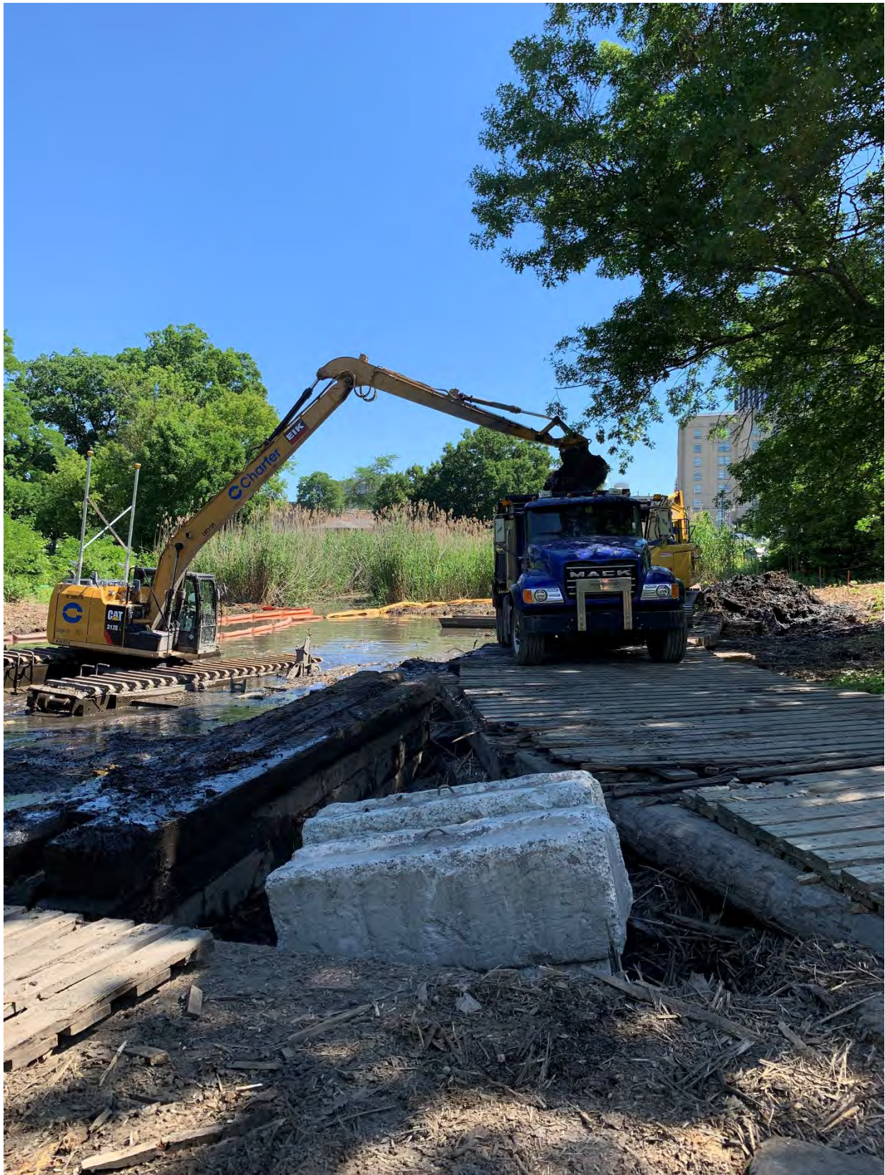
Work Area #6 – section of river by Short Street Bridge to Back Bay Yard – near the intersection of Park Drive and Riverway – upstream area outside of MWRA easement. Dredging of the flood risk management ongoing into July.
