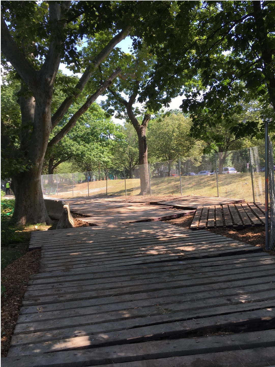
Root protection (8" wood chips and timber matting) and trunk protection (jersey barriers) for protection of existing trees along the construction access roads.
