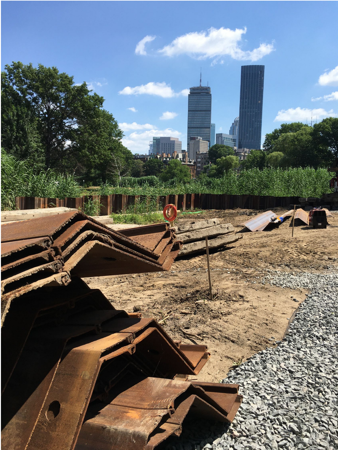
Construction of the Central Processing Area at Work Area #11 (Agassiz Road) with steel sheeting. Central Processing Area will be the primary point of sediment handling prior to disposal.
