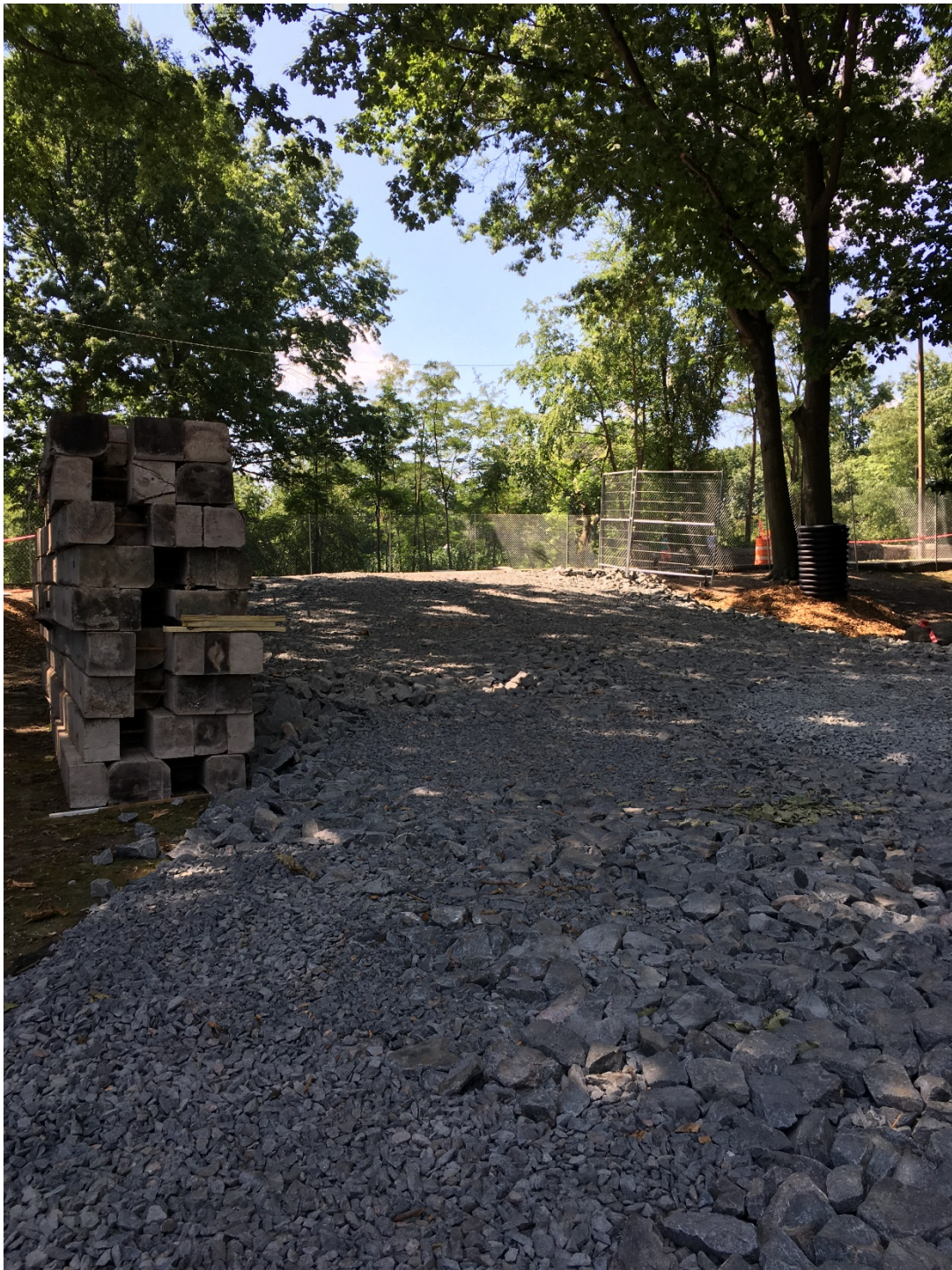
Construction access road at Work Area #11 (Agassiz Road) – constructed on top of 8" wood chips and timber matting for existing tree protection. Note also the corrugated plastic wrap around the tree trunk.
