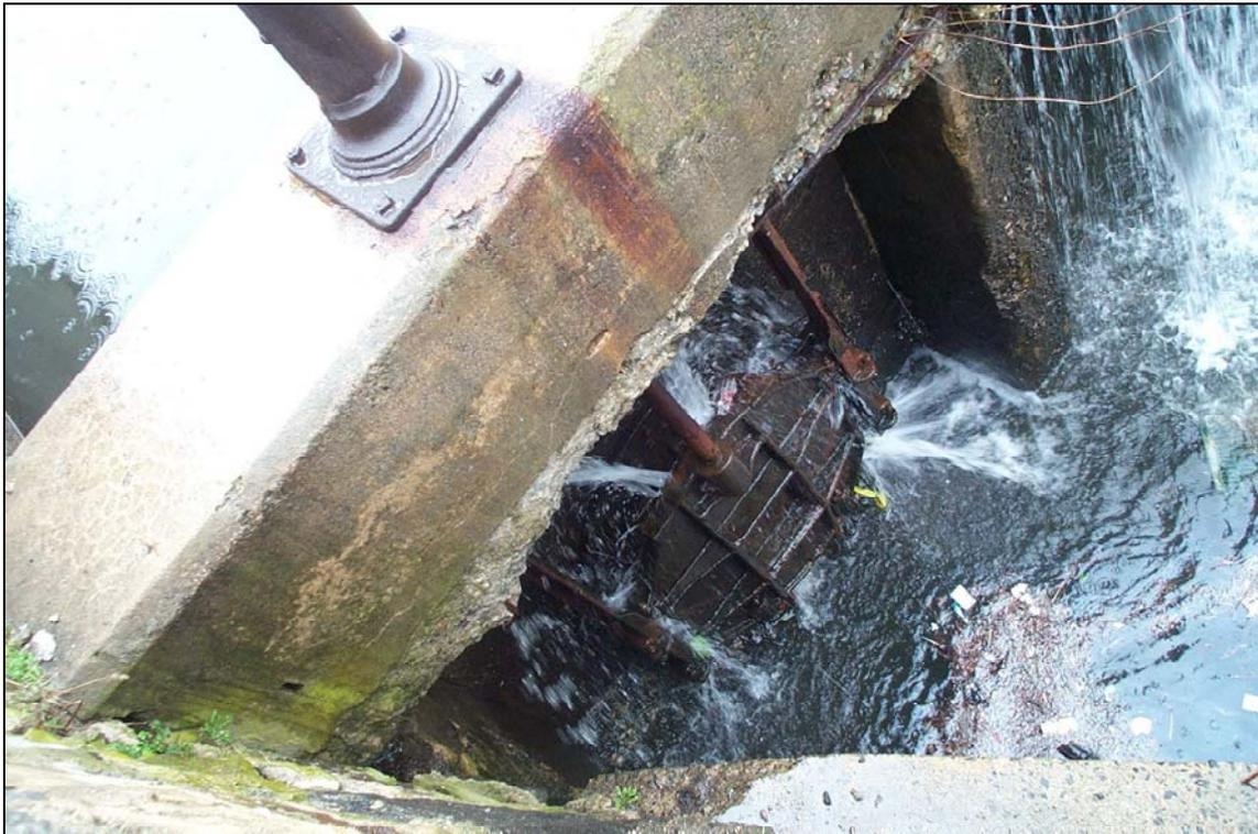
**Plate 3. Failing sluice gate of the Main Street dam**
