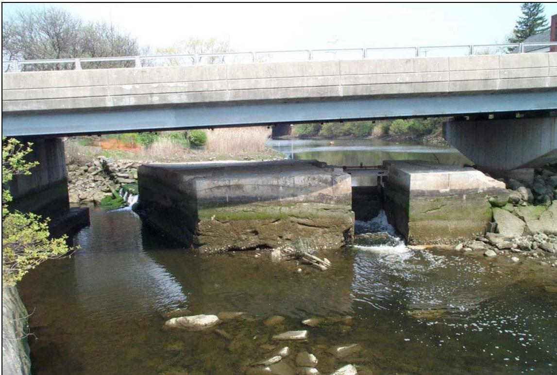
**Plate 8. Concrete obstruction under Pulaski Street Bridge on the Mill River in Stamford, CT. This abandoned structure blocks fish passage during mid and low tides.**
