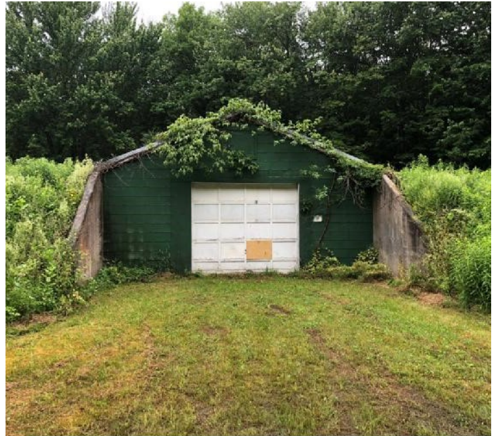
Former Bunker area, June 2018.
