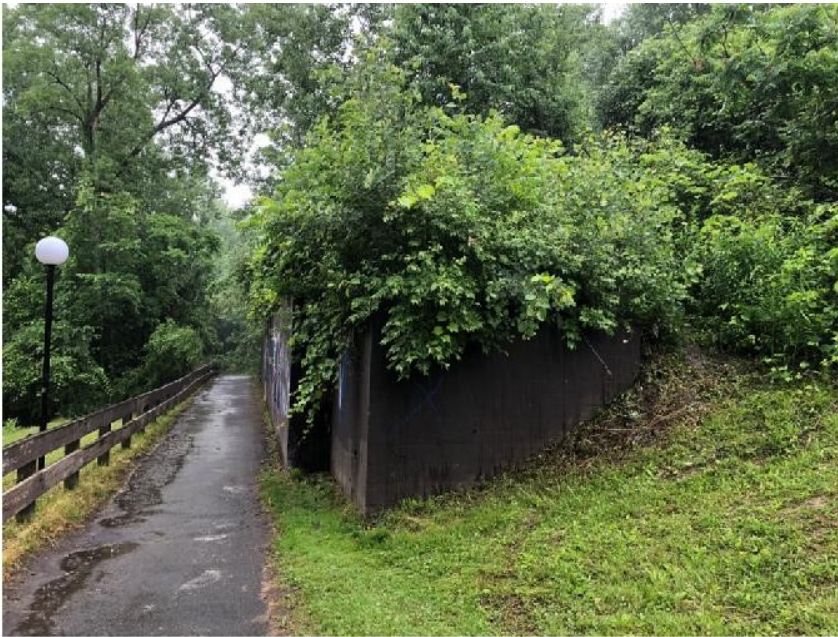
Former Ammonium Picrate area, June 2018.
