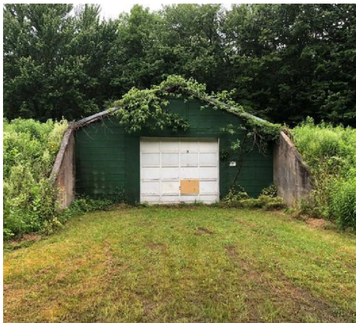
Former Bunker area, June 2018.
