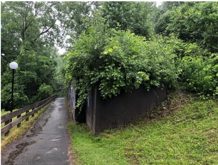
Former Ammonium Picrate area, June 2018.
