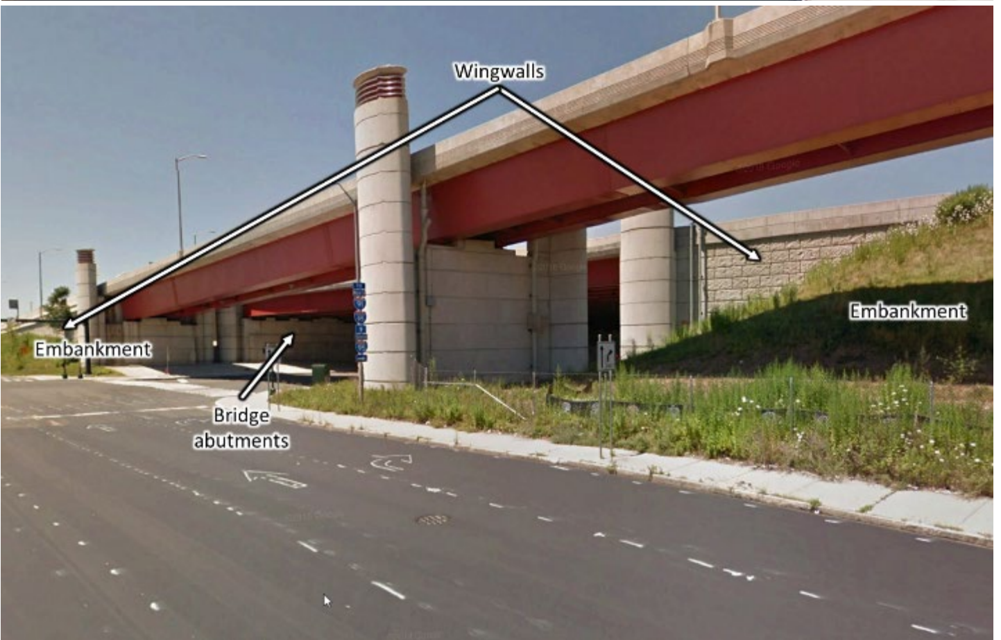
Figure 29: Canal Dock Road Bridge under I-95
