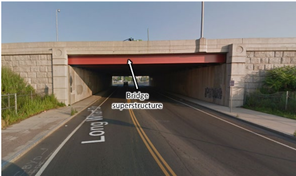
Figure 13: Photo showing typical bridge superstructure
