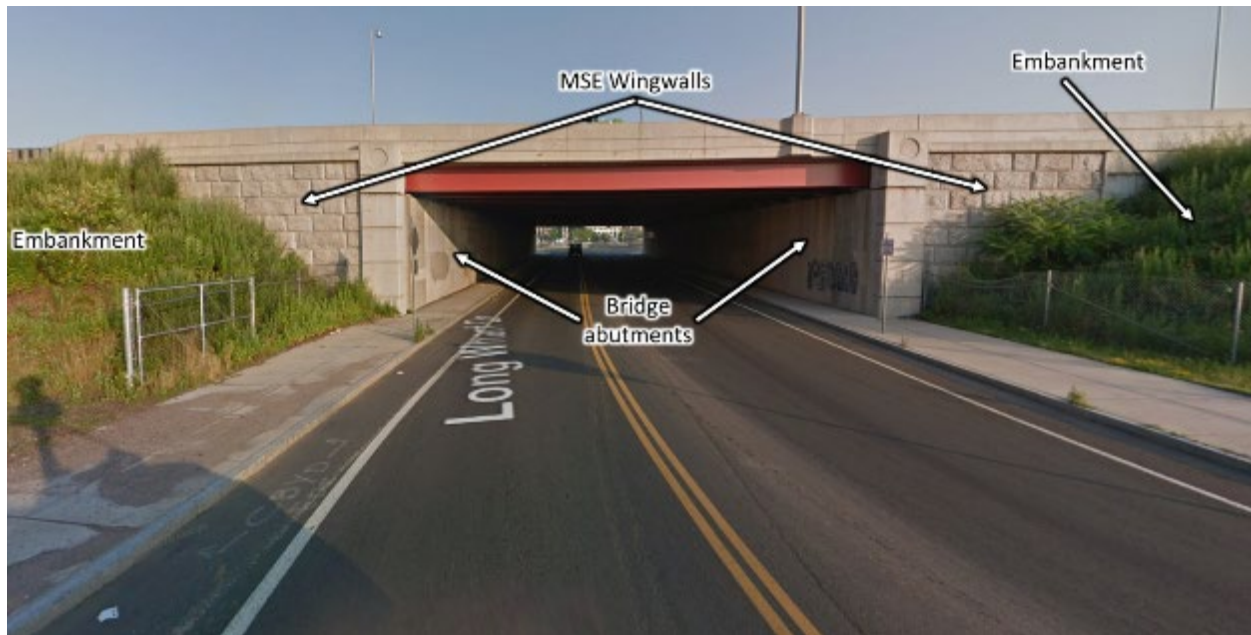
Figure 14: Photo showing location of MSE wingwalls
