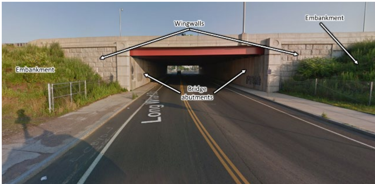
Figure 11: Bridge overpass at Long Wharf Drive viewed from ocean side.
