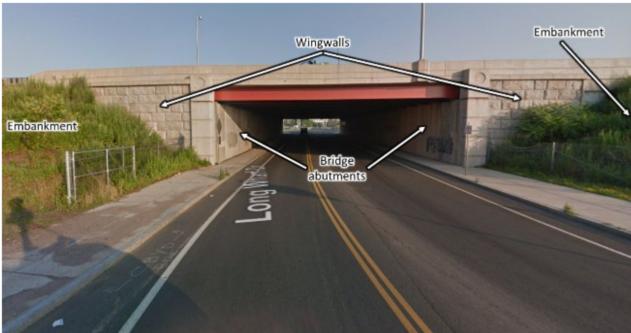
Figure 19: Long Wharf Drive Bridge Overpass, I-95 embankment
