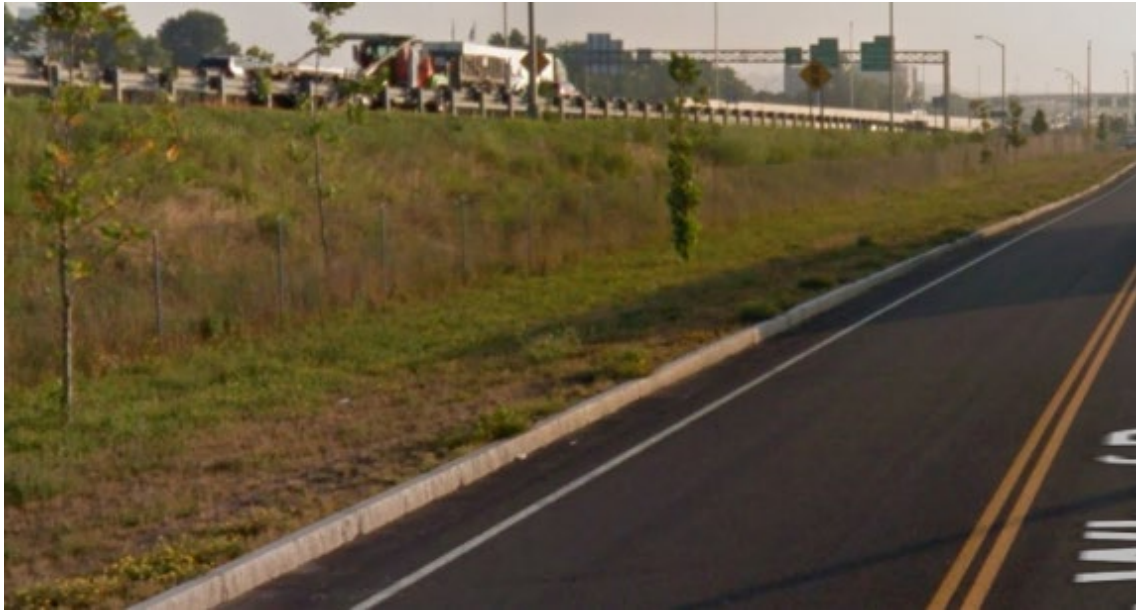
Figure 4: View of ocean side of I-95 embankment from Long Wharf Drive overpass looking northeast.
