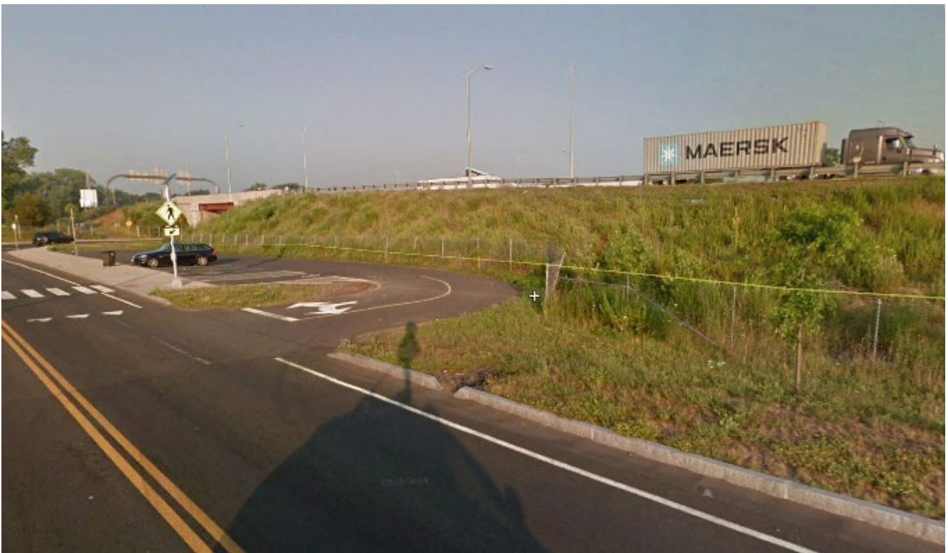
Figure 24: Typical condition of I-95 embankment
