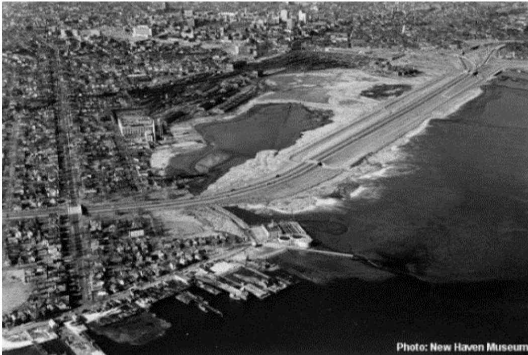
Figure 9: Construction of the I-95 embankment circa 1950s
