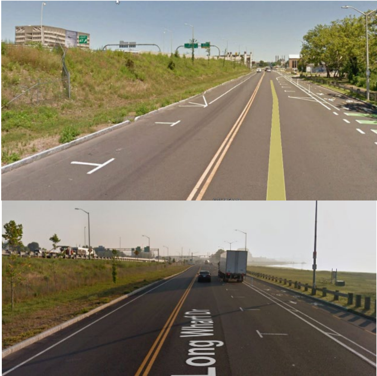
Figure 16: Typical condition of seaward face of I-95 embankment
