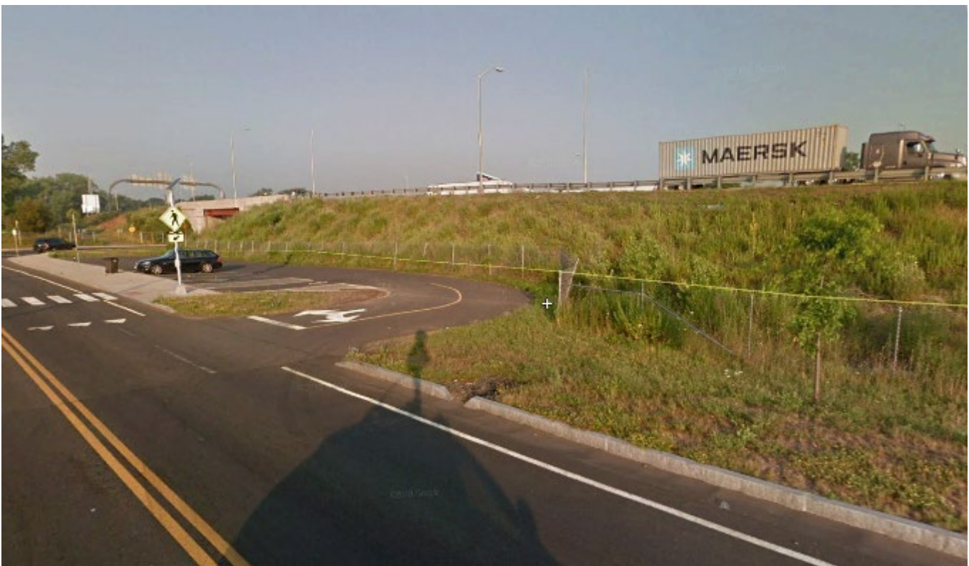
Figure 25: Typical condition of I-95 embankment
