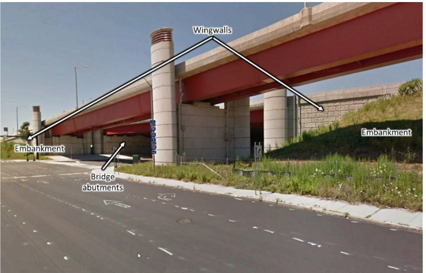
Figure 21: Canal Dock Road Bridge under I-95
