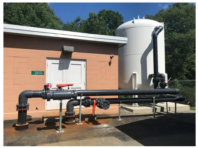
Devens installed a single GAC filter in June 2019. Has been treating ~ 600K GPD since activation on 8-5-19.
