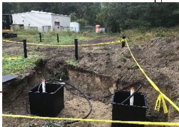
Construction of injection wells
