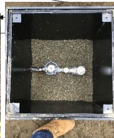
Completed injection well
