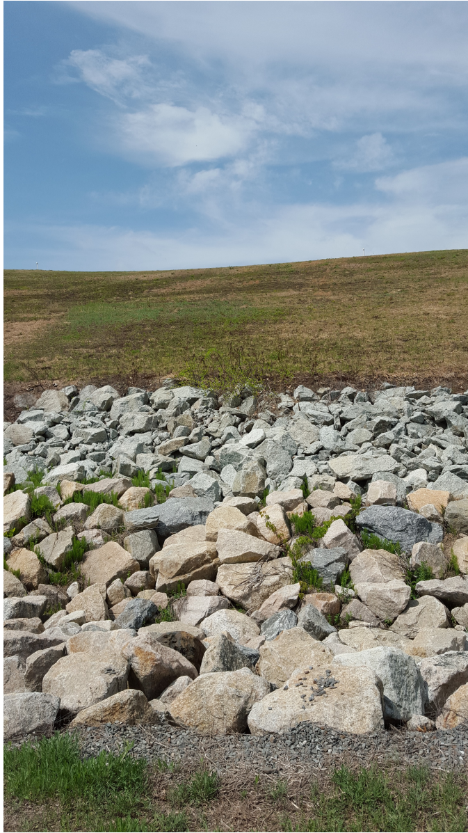
DCL slope, cap in good condition, riprap at toe
