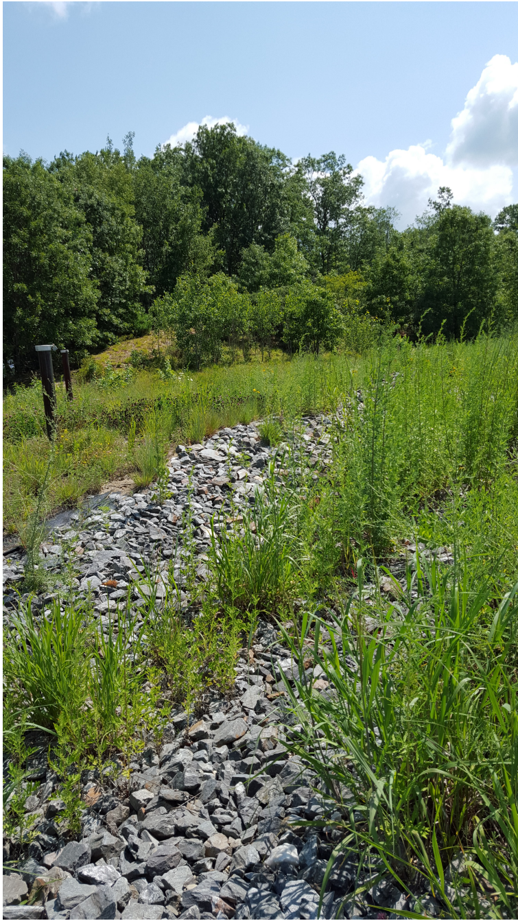
Riprap at barrier wall
