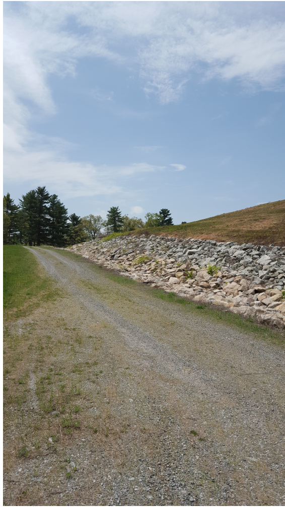
Toe of DCL, roadway and riprap
