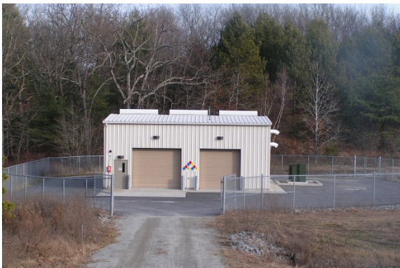
Shepley's Hill Landfill Arsenic Treatment Plant
