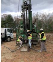
Rig pushes drill rods into the ground to remove soil/rock
