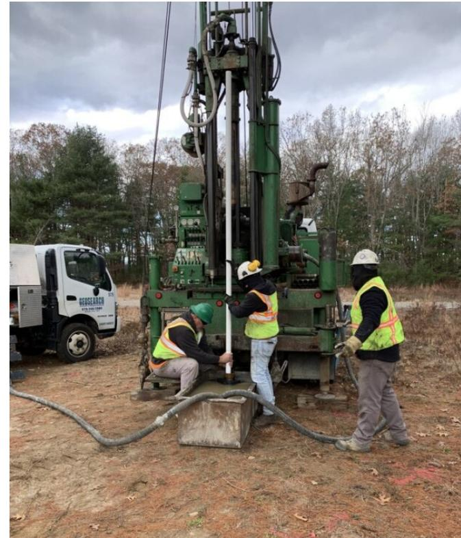
PVC pipe is installed to create the well
