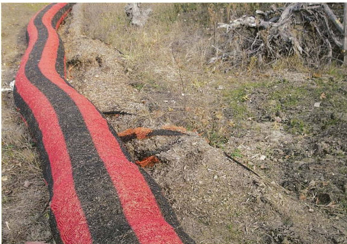
AOC 57 Area 2: Close-up of the newly installed erosion control tube (red & black stripes) to replace the degraded erosion control tube (orange & black stripes) (November 1, 2005).
