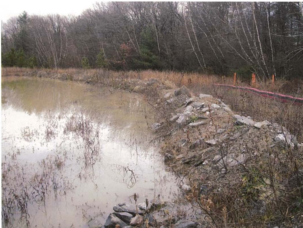
AOC 57 Area 2: Pool of storm water in front of berm installed in 2006 parallel to erosion control tube (top right corner) to well beyond the eastern edge of Area 2 (November 14, 2006).
