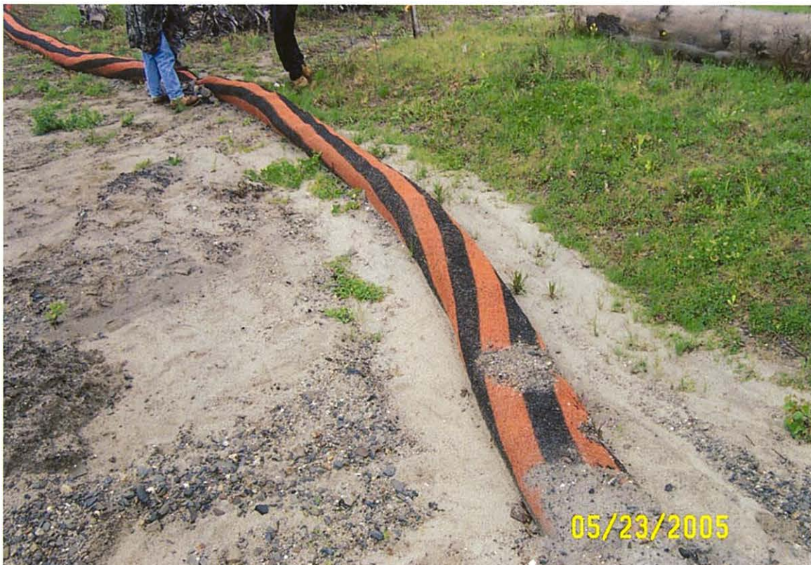
AOC 57 Area 2: Close-up showing the failed section of the erosion control tube and sedimentation from upgradient soil stockpiles (May 23, 2005).
