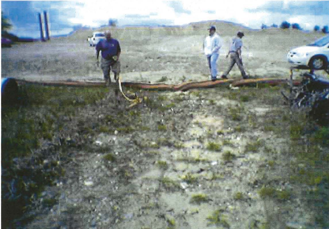
AOC 57 Area 2: Erosion of upgradient stockpiled soils onto the restored upland as a result of the failed erosion control tube as observed by the Groundwater LTM Team (May 19, 2005).
