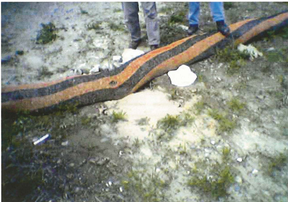
AOC 57 Area 2: Immediate corrective action taken by the Groundwater LTM Team to block the undermining by filling with nearby rock (May 19, 2005).
