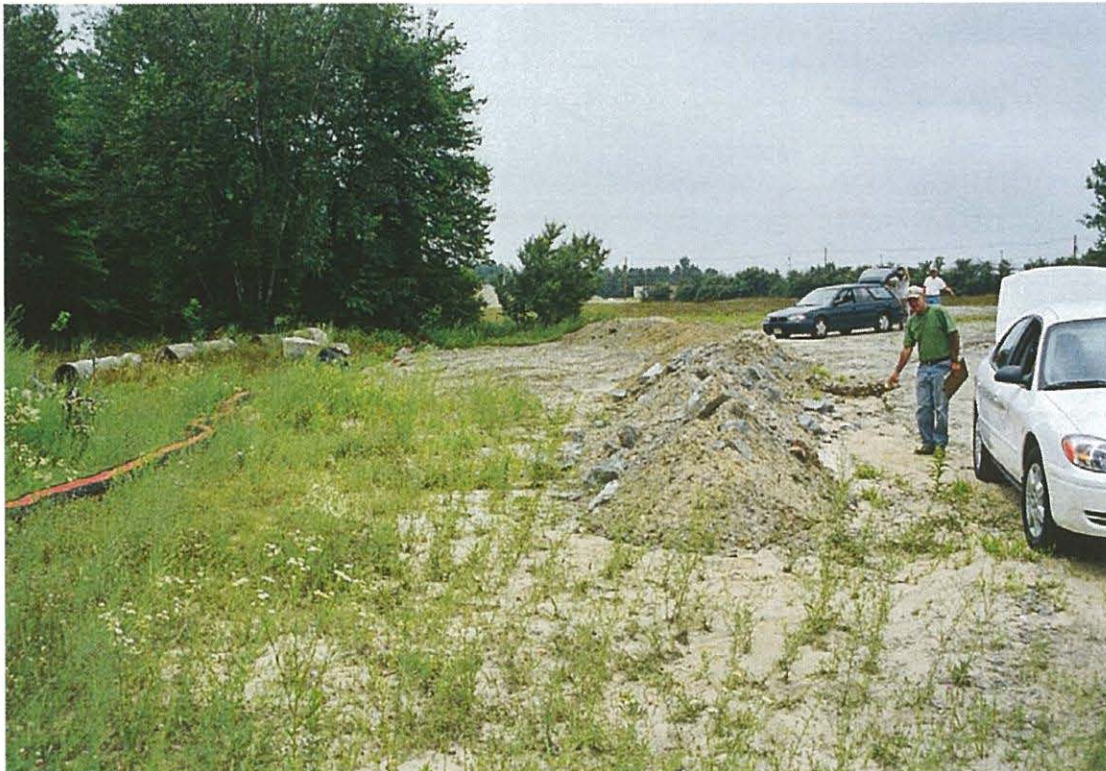
AOC 57 Area 2: Close-up of newly constructed unvegetated berm installed parallel to the erosion control tube that only extended to the eastern edge of the site (July 14, 2005).
