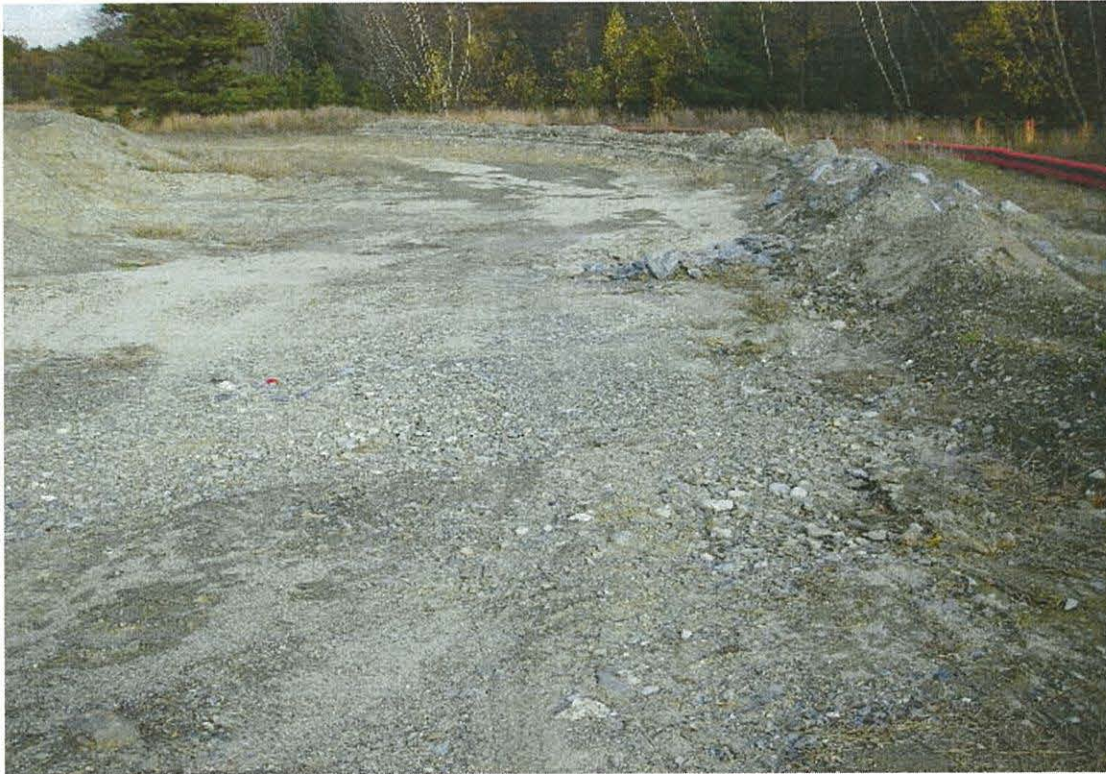
AOC 57 Area 2: Extension of the unvegetated berm installed parallel to the erosion control tube to well beyond the eastern edge of the site (November 1, 2005).
