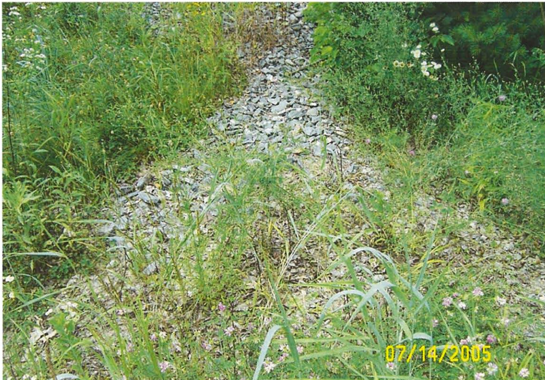
AOC 57 Area 2: Area immediately below the drainage channel established to protect the slope from erosion and armored with rip rap stone on the east side of the slope showing indications of erosion and sedimentation (July 14, 2005).
