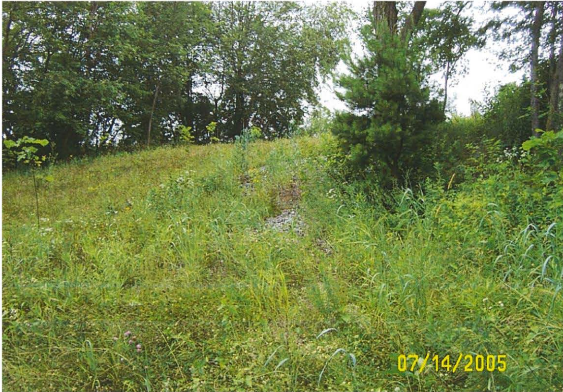
AOC 57 Area 2: Area immediately below the drainage channel established to protect the slope from erosion and armored with rip rap stone on the east side of the slope showing indications of erosion and sedimentation (July 14, 2005).
