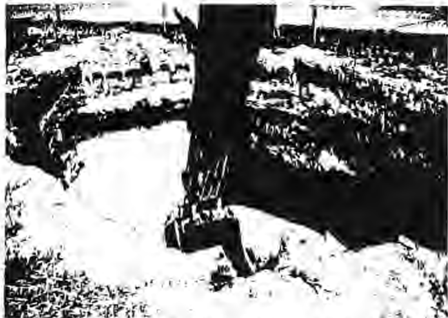
(6) Excavation of marked off area to 10 ft; first 20 ft hole being backfilled.
