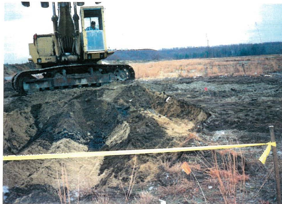
18. Stained soil encountered on south side - December 14
