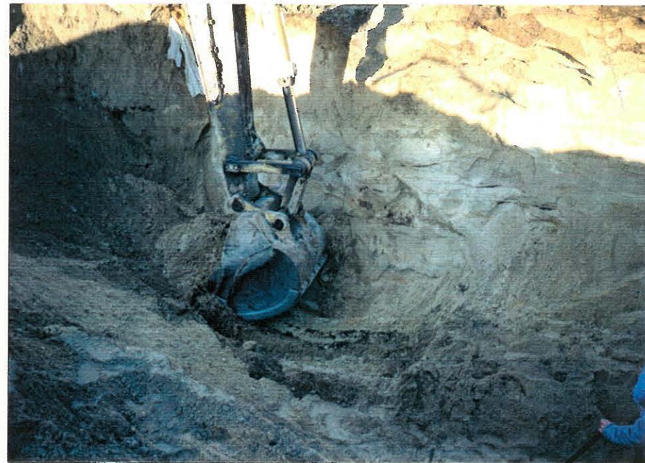
24. Removal of stained soil from bottom - December 16
