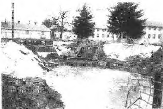
Backfilling of excavation
