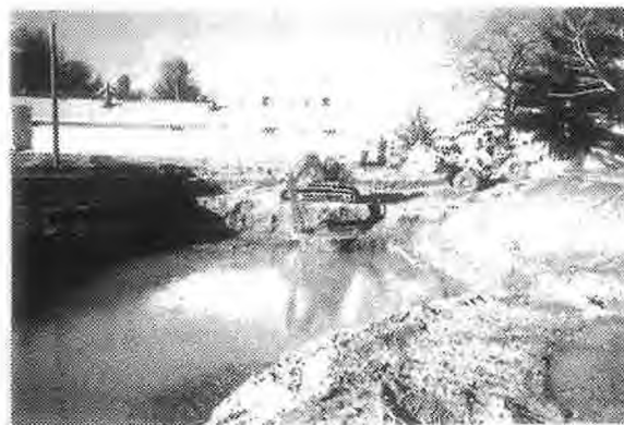
Removal of contaminated soil from excavation
