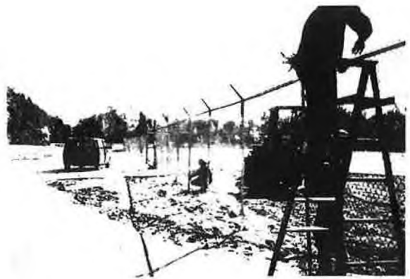
Re-installation of Existing Fence
