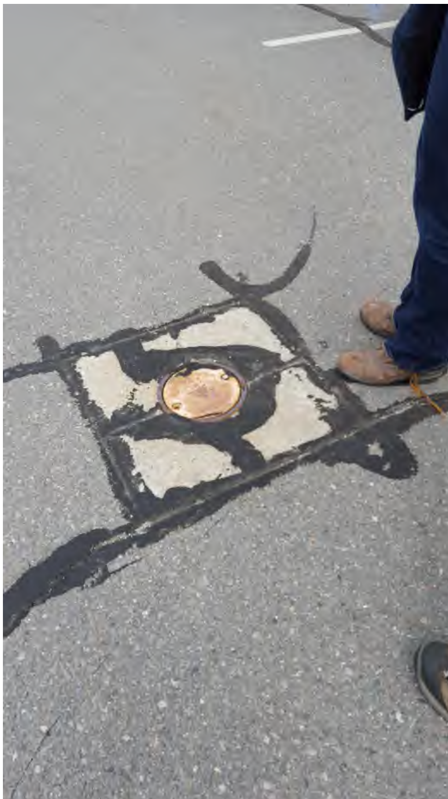
Excessive crack sealing around monitoring wells noted on site.
