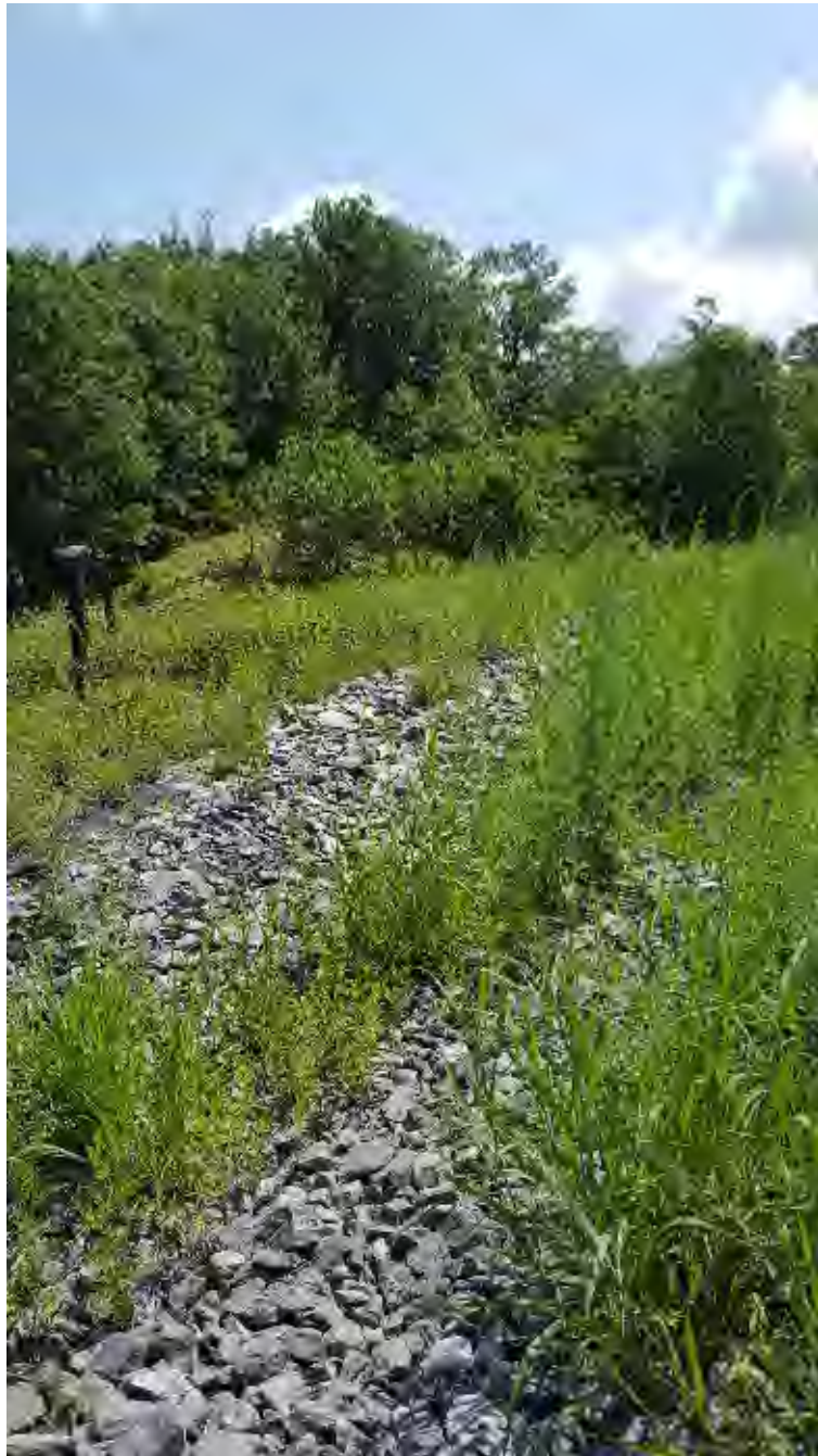
Riprap at barrier wall
