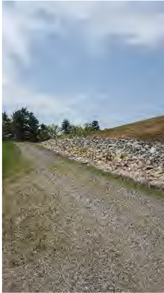
Toe of DCL, roadway and riprap
