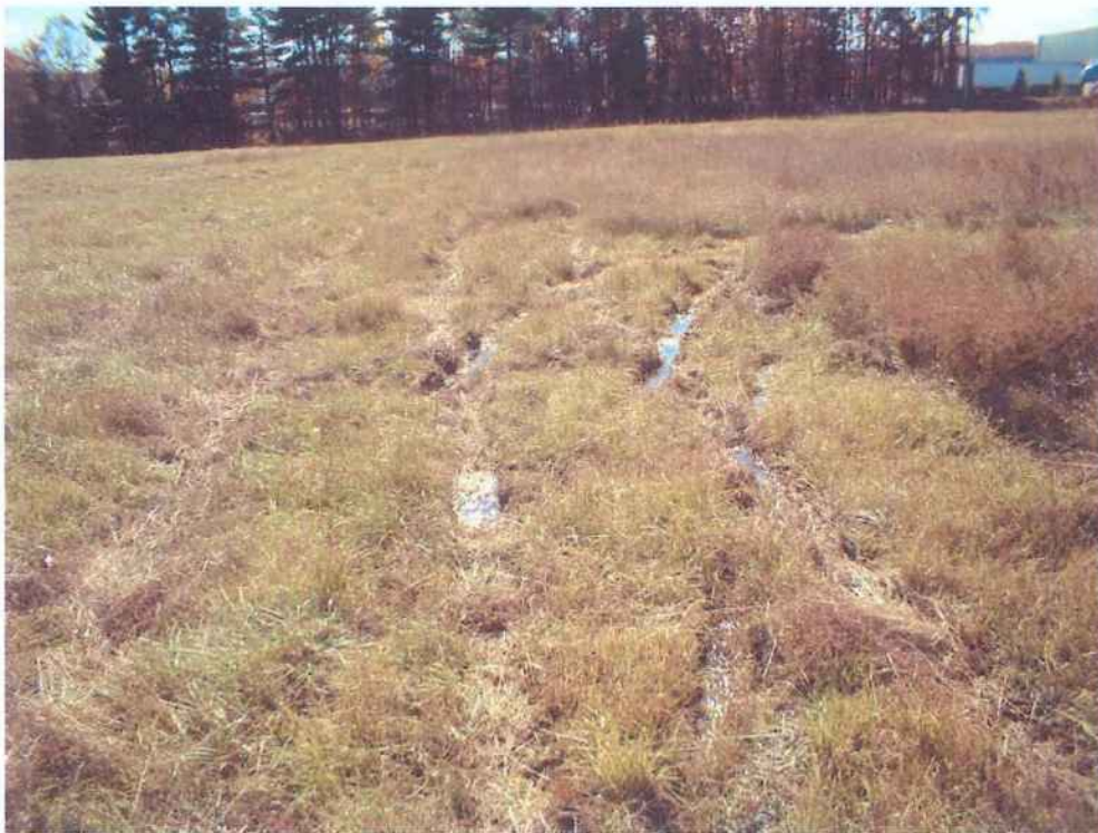
Photo 8 – Ruts in surface soils on south side of landfill from trespassing vehicles or mowing equipment.
