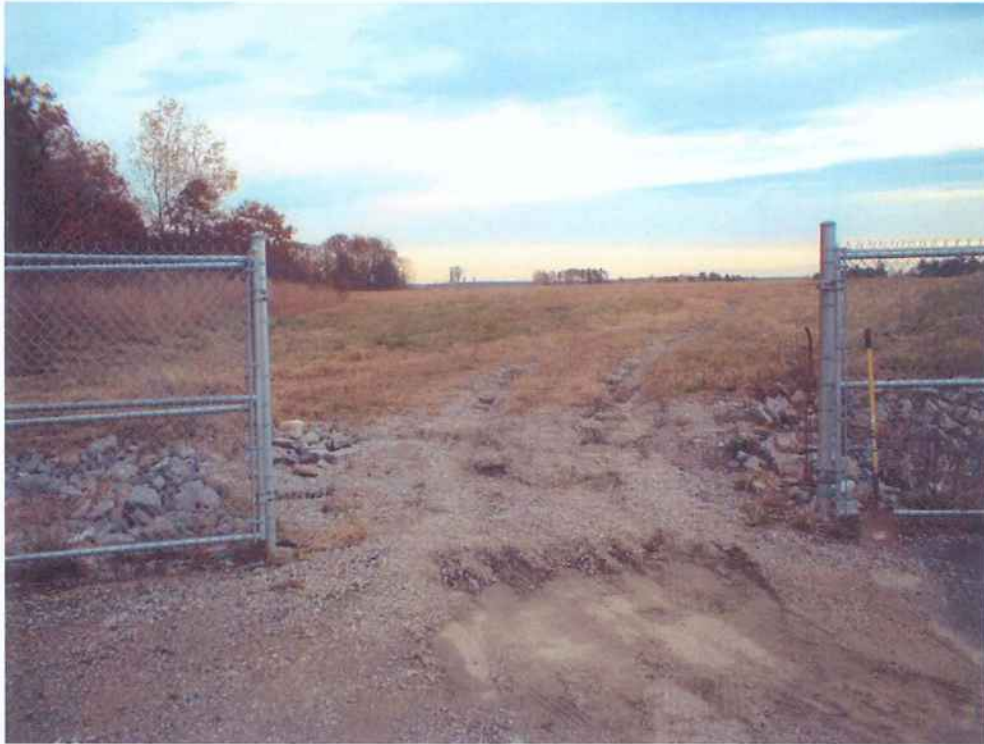
Photo 6 – View south of erosion/deposition of gravel from access road near northeast corner of landfill near gate for treatment plant.
