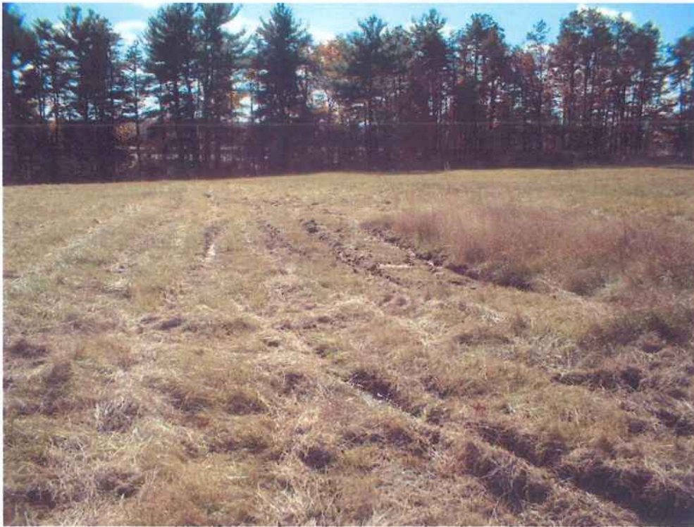
Photo 9 - Ruts in surface soils on south side of landfill from trespassing vehicles or mowing equipment.
