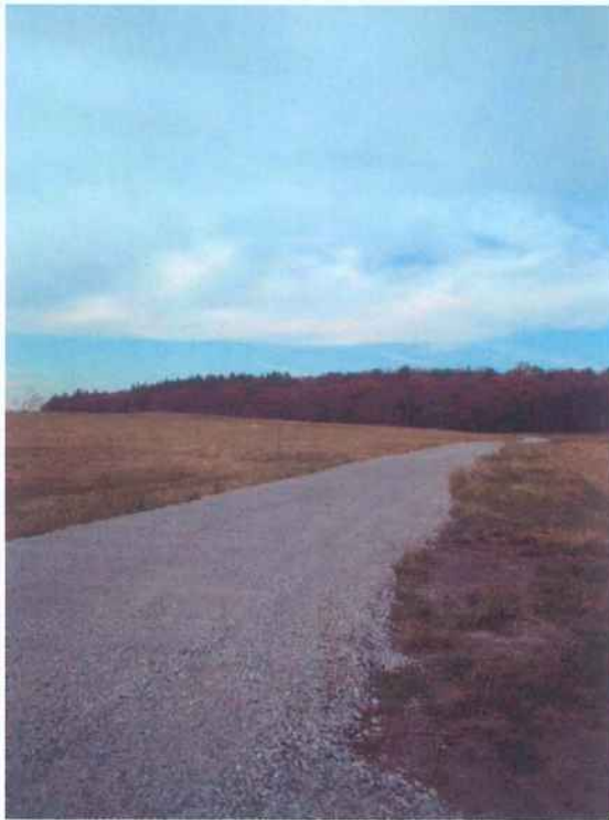
Photo 2 - New dense-grade road across landfill.
