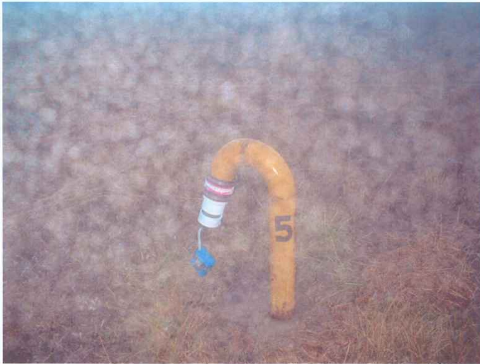
Photo 7 – Older vent with limited corrosion.
