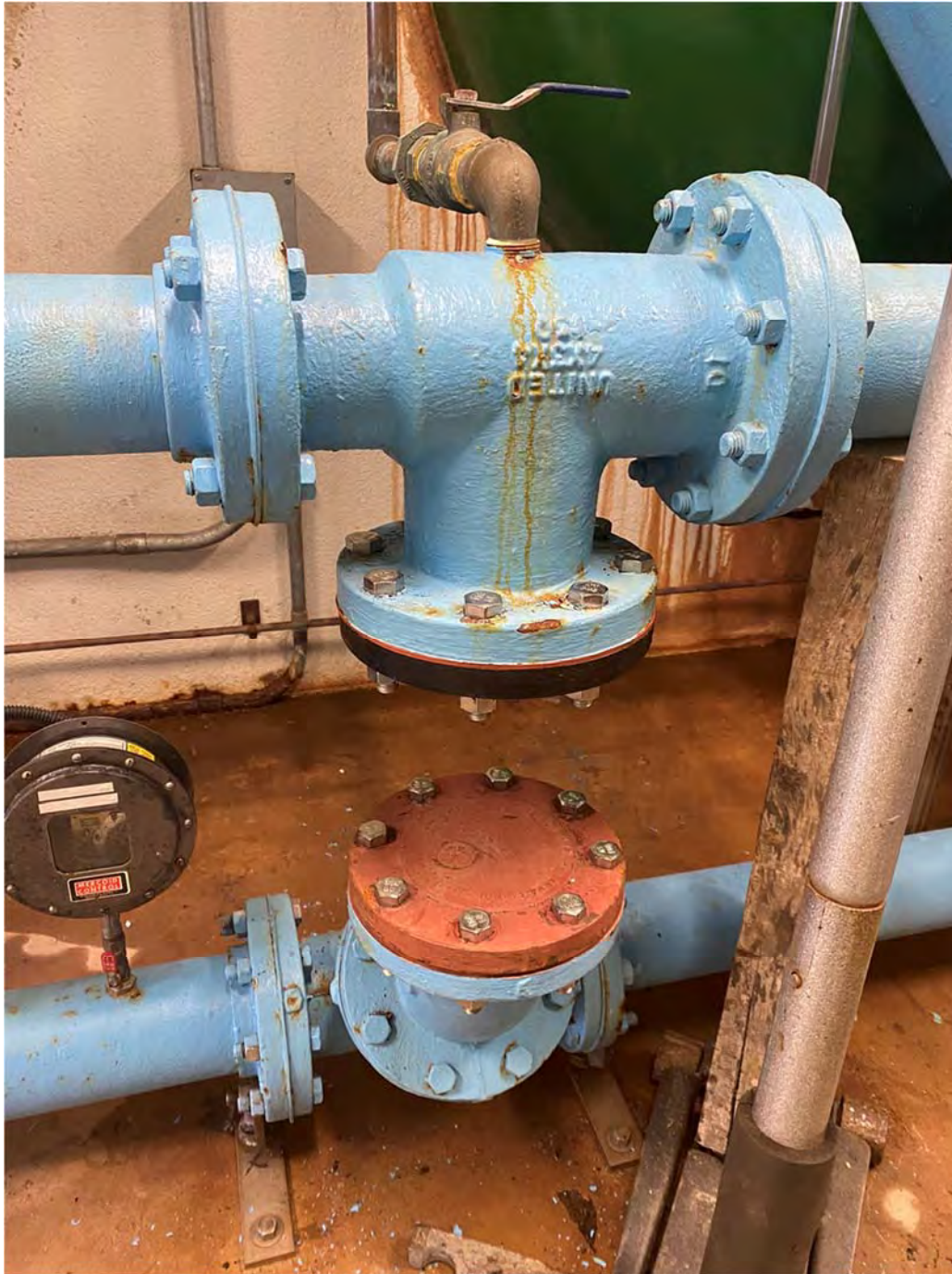
Picture 3: Booster station spool pipe removed, and blind flanges installed.
