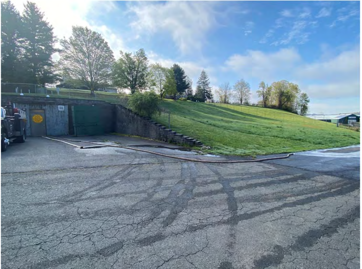
Picture 2: Water from the storage tanks at the Durham Booster Station being drained to the ground surface. View to the southeast.
