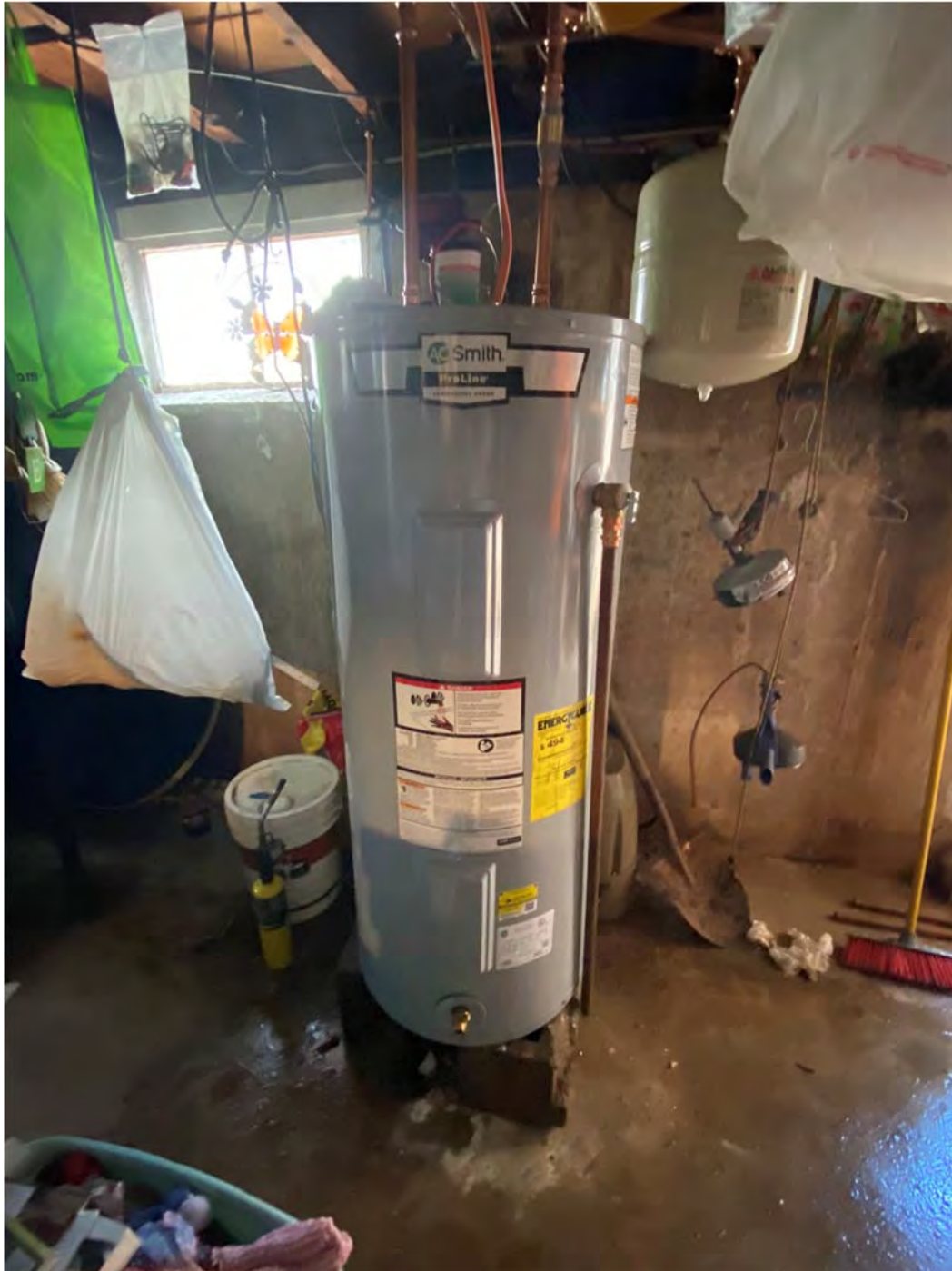
Picture 5: Fazzino Plumbing replaces the hot water heater at 187 Maple Avenue.
