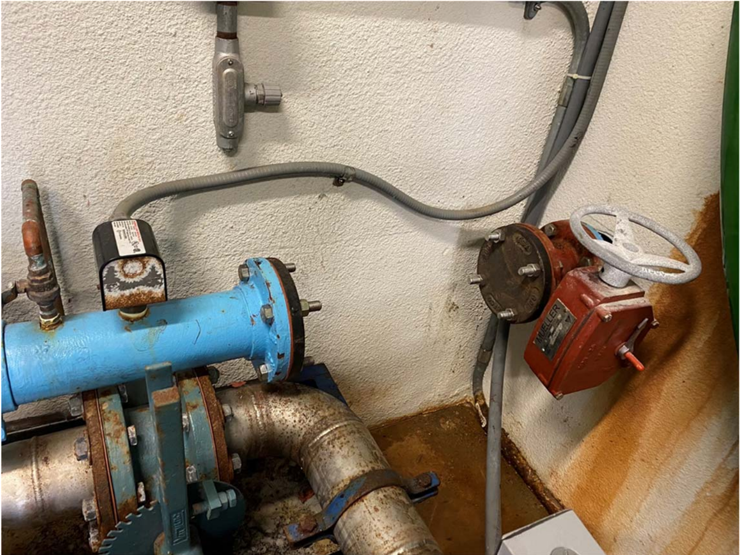
Picture 4: Ludlow removes the 3" well meter and caps both sides. View to the east.
