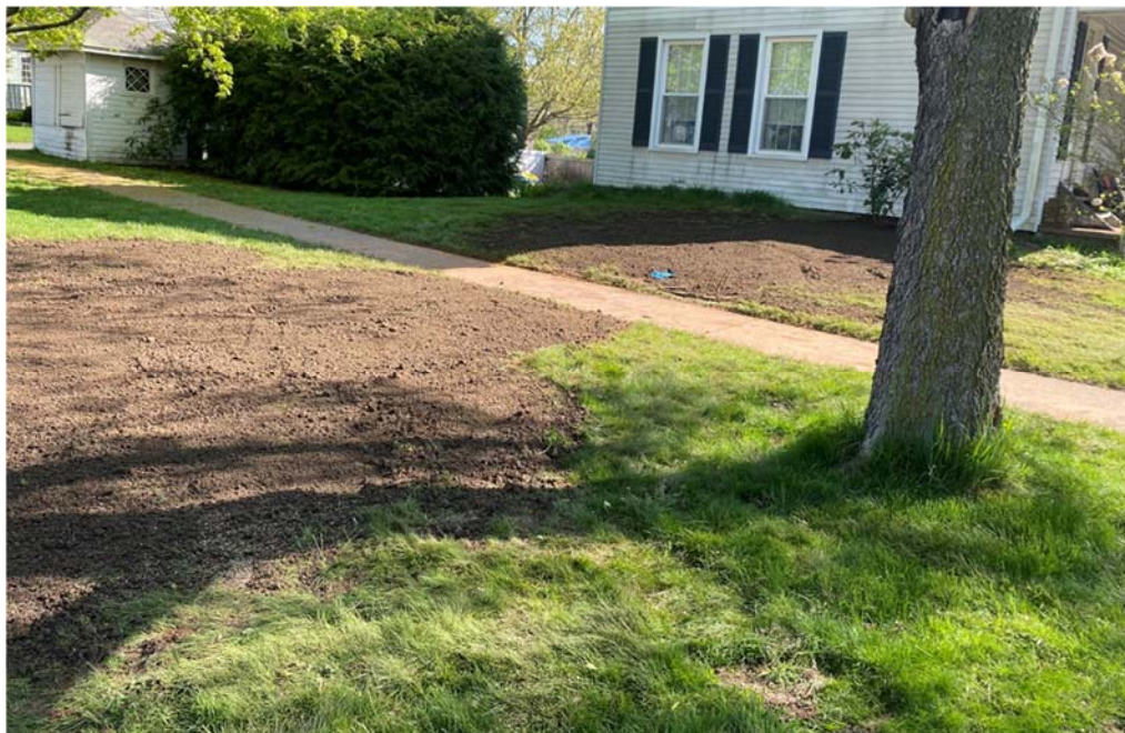
Picture 1: The water service trench has been backfilled, compacted, and grass seed was spread over the trench for the service connection to 55 Main Street. View to the east.
