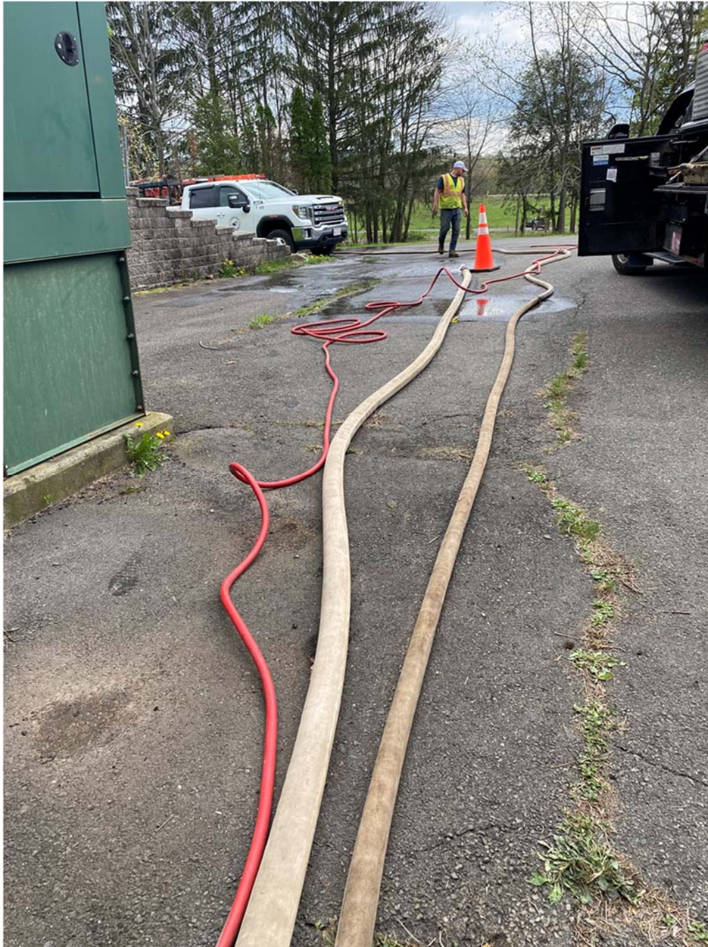
Picture 2: Ludlow connects to the 3 tanks in the booster station using a 1", 2" and 3" hose to empty the tanks of water out the pump station and down the hill. View to the west.
