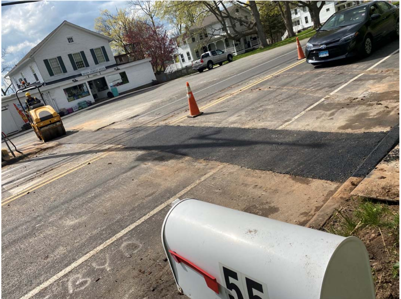
Picture 7: Ludlow completes paving on Main Street over the trench for the water service to 55 Main Street. View to the west.
