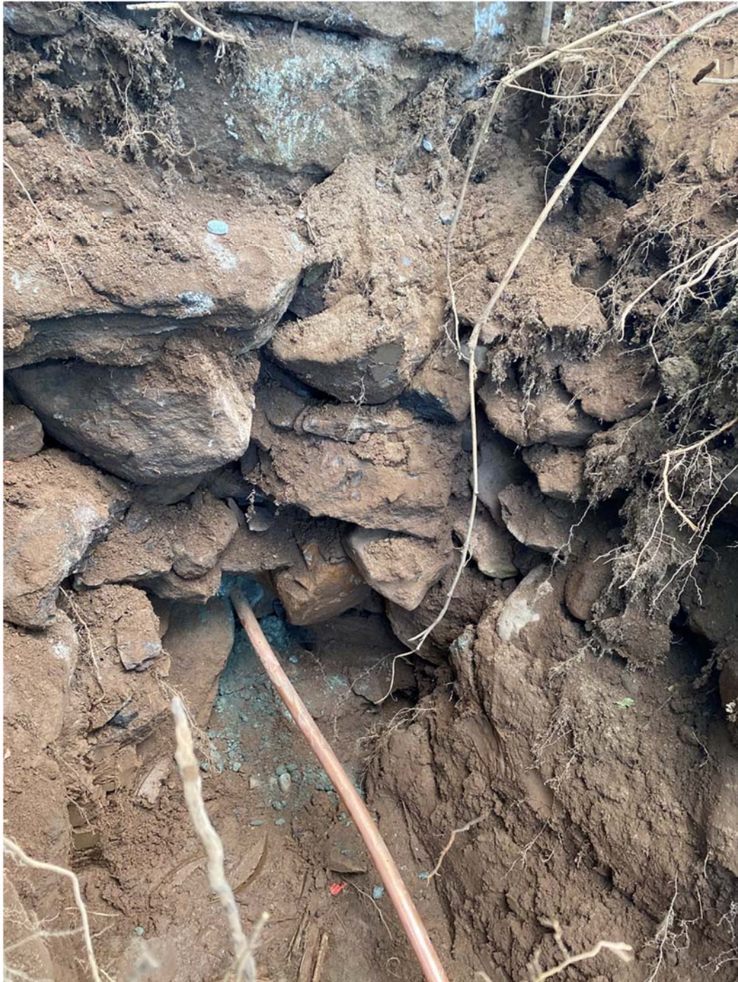
Picture 4: The 1" copper cubing has been inserted through the stone foundation for 55 Main Street.
