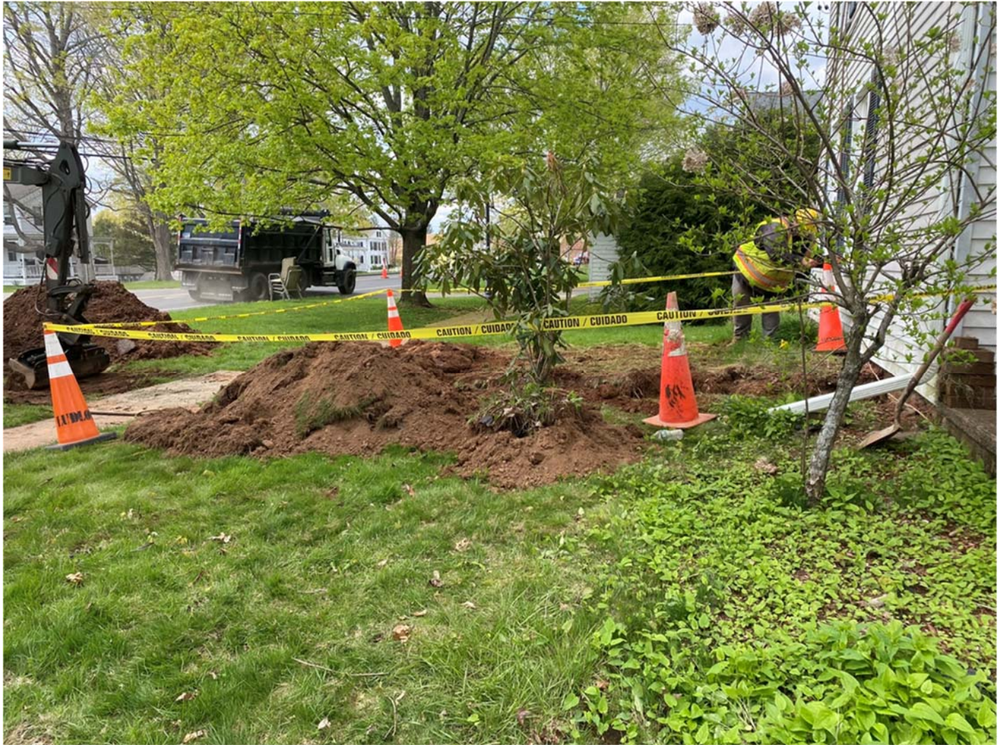
Picture 8: The partially open trench in the front yard of 55 Main Street is surrounded by safety cones and caution tape and left overnight. The backfill will be completed tomorrow morning. View to the north.
