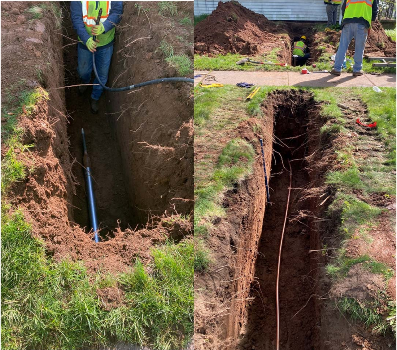
Picture 3: A mole is used to penetrate a small channel beneath the sidewalk which the 1" copper tubing can run through towards the house for the water service connection. View to the east.
