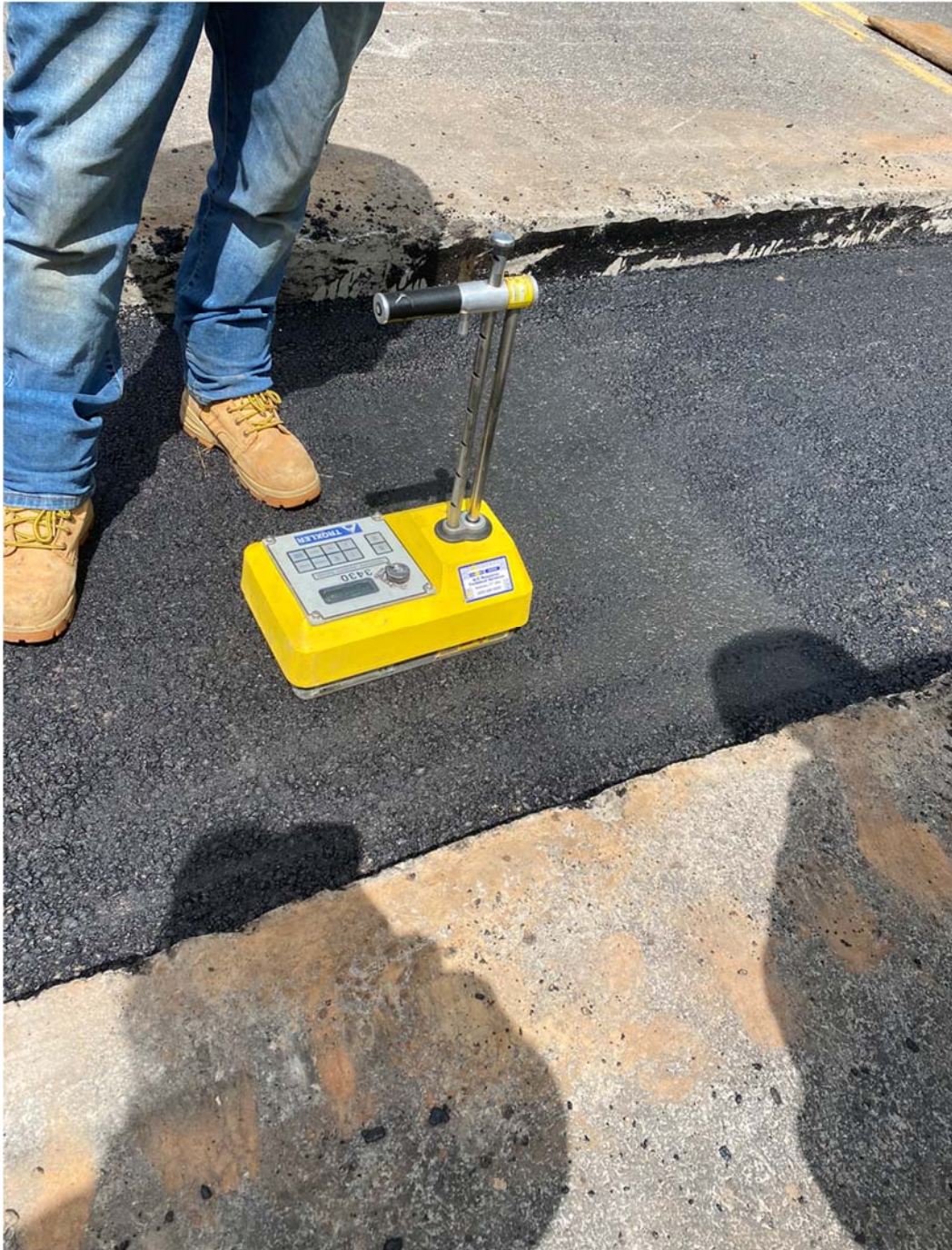
Picture 6: Ludlow places asphalt over the trench of the service to 55 Main Street. Compacted in 3" lifts. Asphalt is compaction tested after each lift by John Turner Testing.
