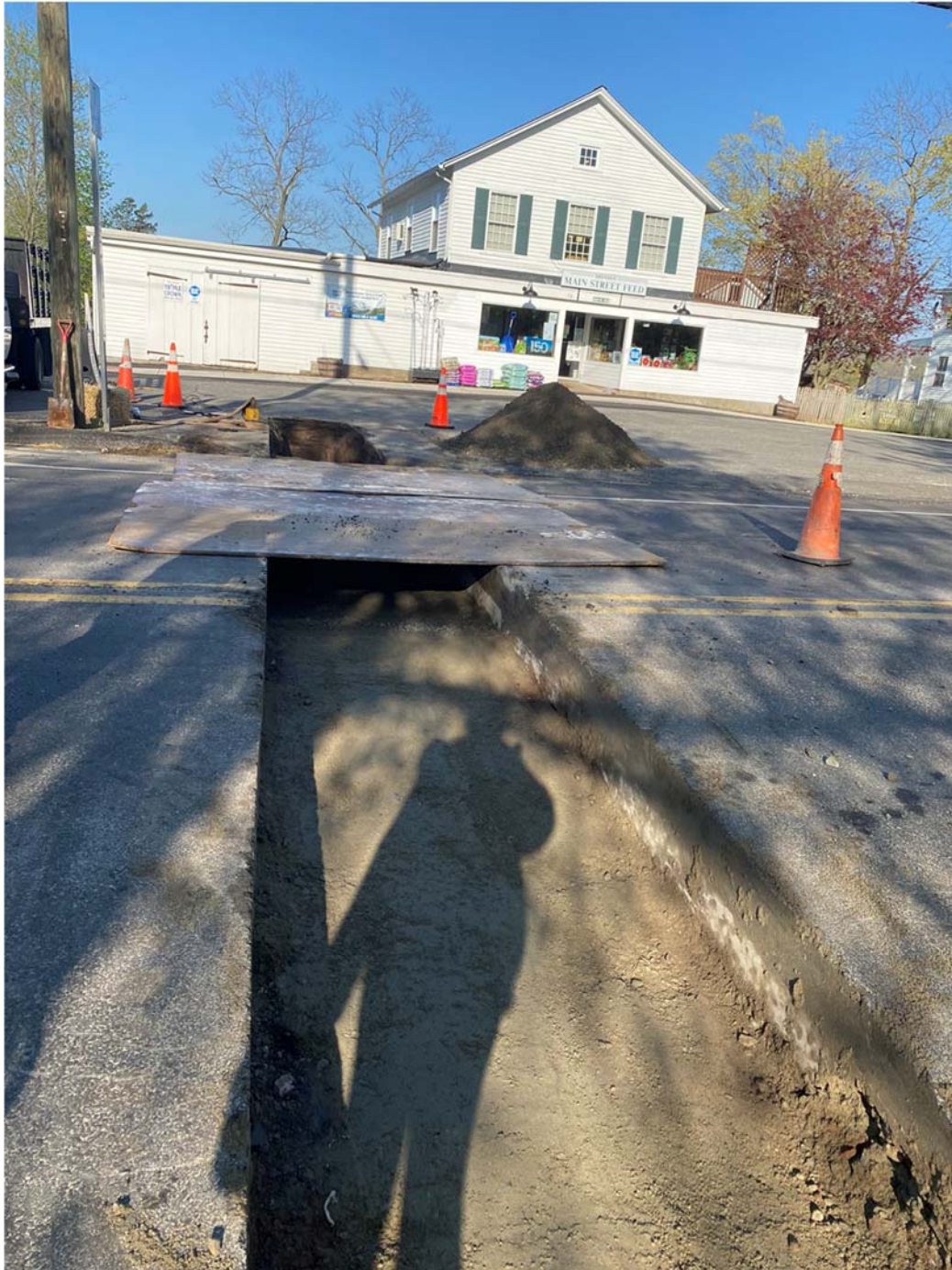
Picture 1: Ludlow removes the 4" temporary trench pavement which was placed Friday and excavates down to a depth of 14". View to the west.
