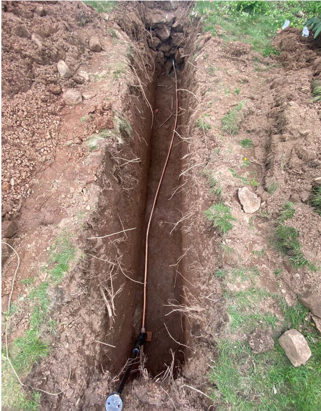
Picture 5: Ludlow has connected the water service from 55 Main Street to the new curb stop. View to the east.
