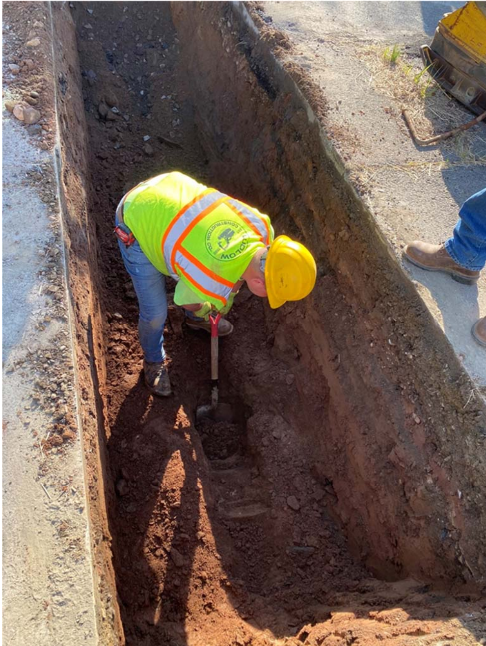
Picture 1: Ludlow excavates and hand digs to locate the PVC water main to connect water service to 55 Main Street, Durham.
