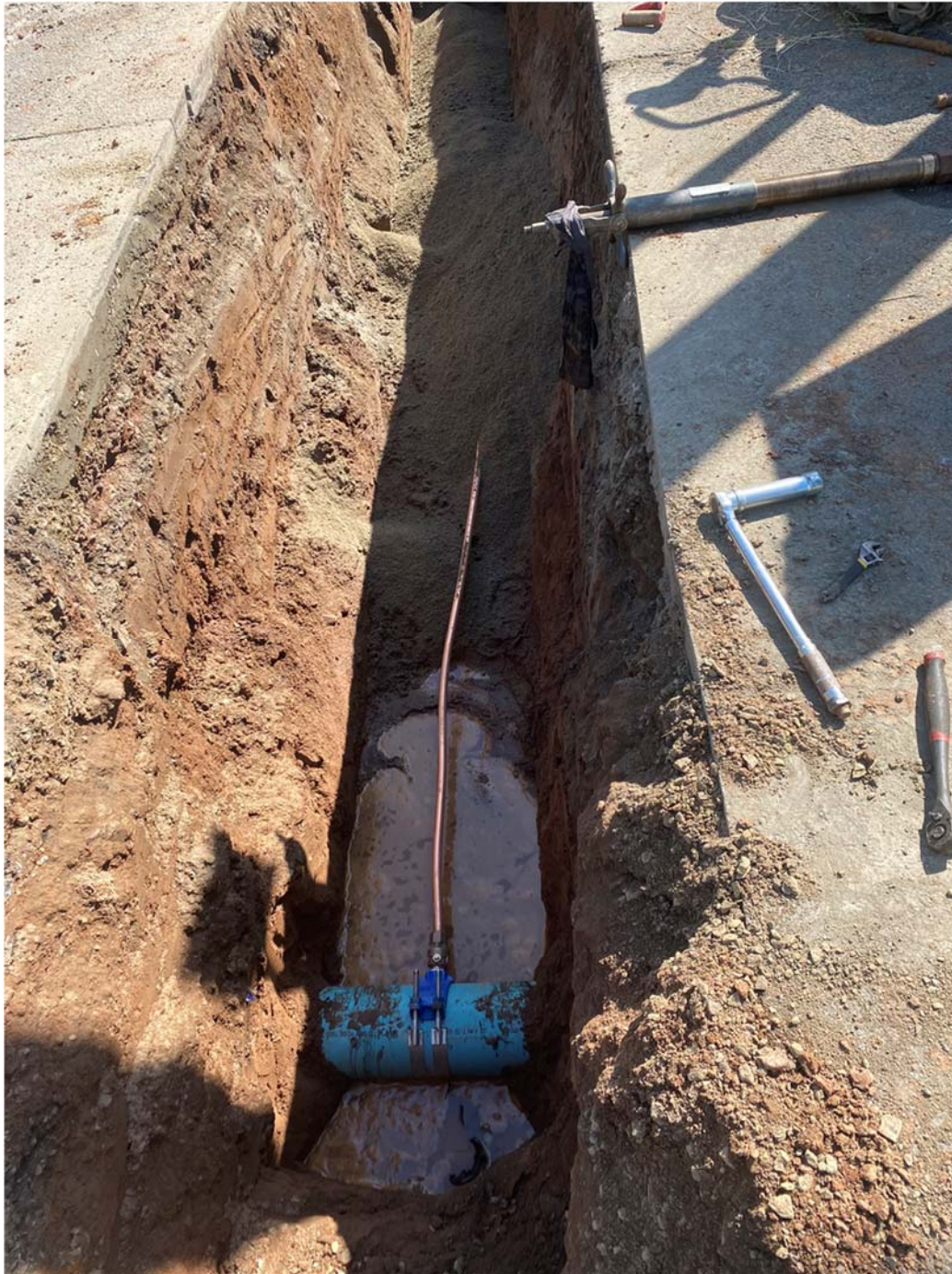
Picture 2: Ludlow taps the 8" diameter PVC water main and connects the 1" copper water service tubing. View to the east.
