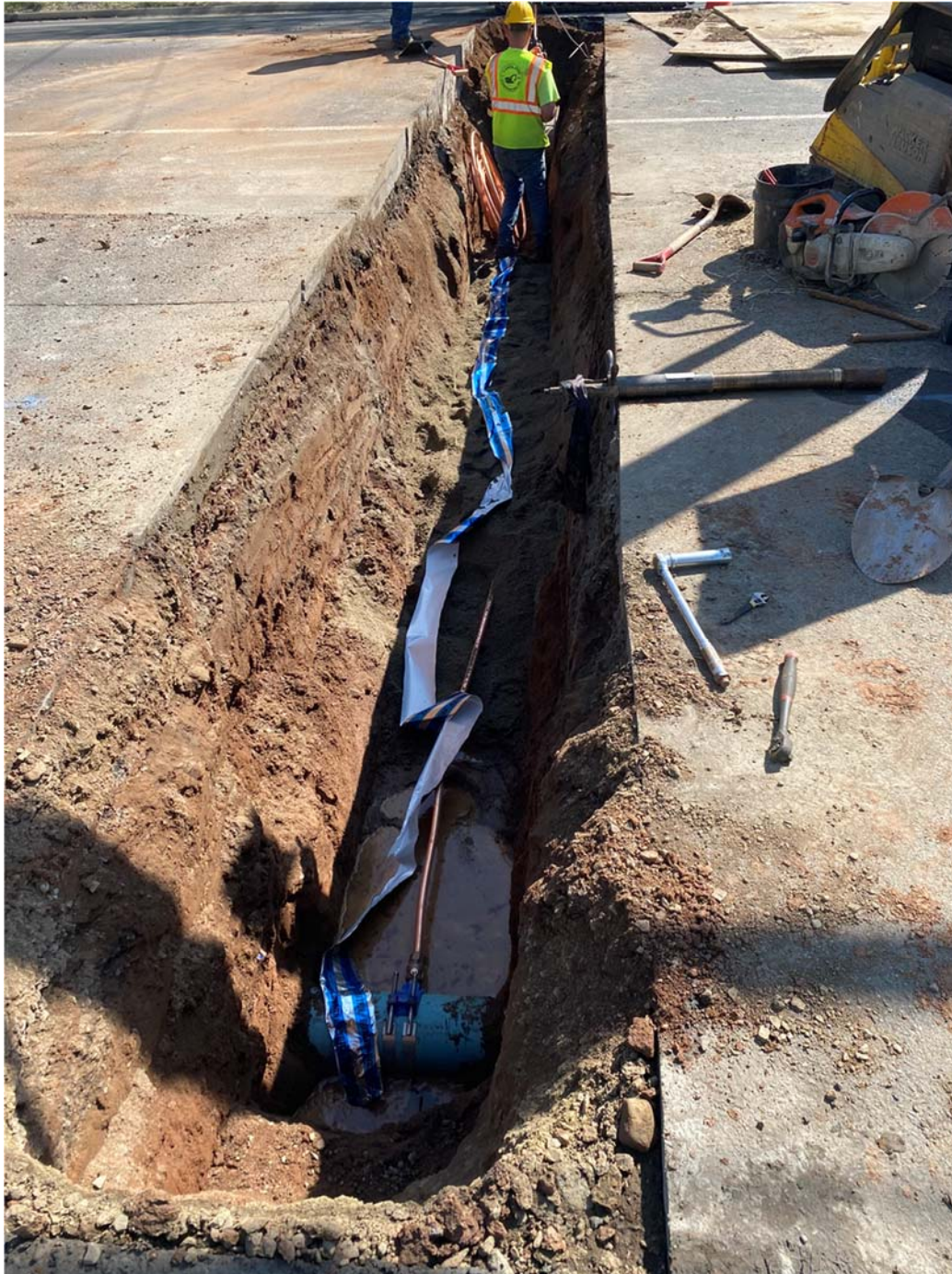
Picture 3: Blue utility warning tape is placed over the 2' of backfill over the service connection tubing for 55 Main Street
