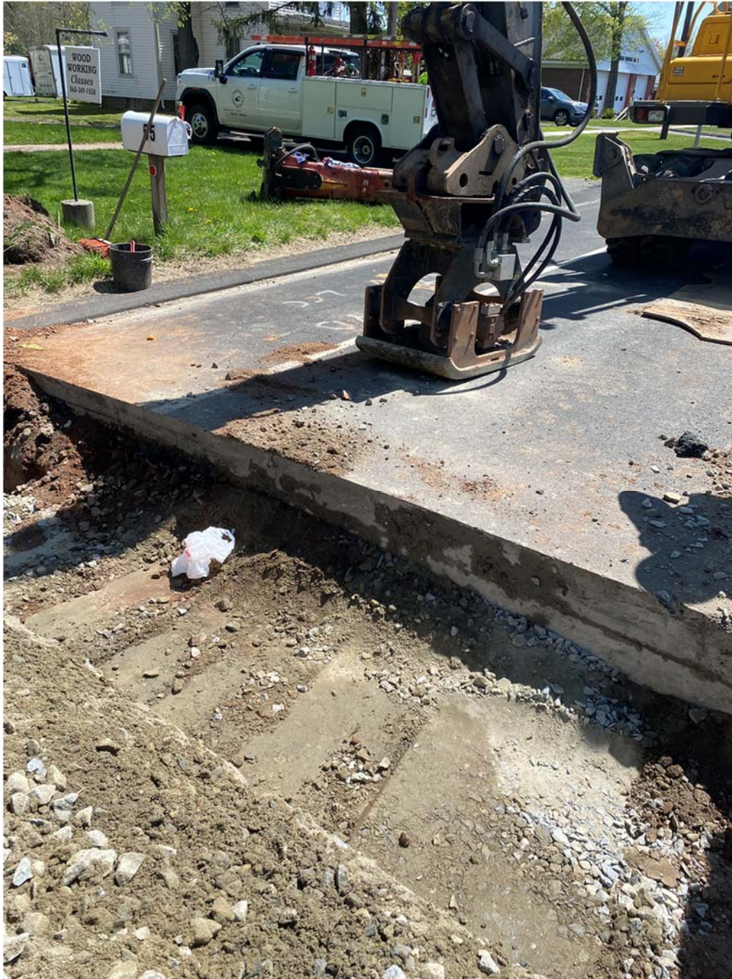
Picture 4: Ludlow uses the hoe ram to compact the processed stone backfill.
