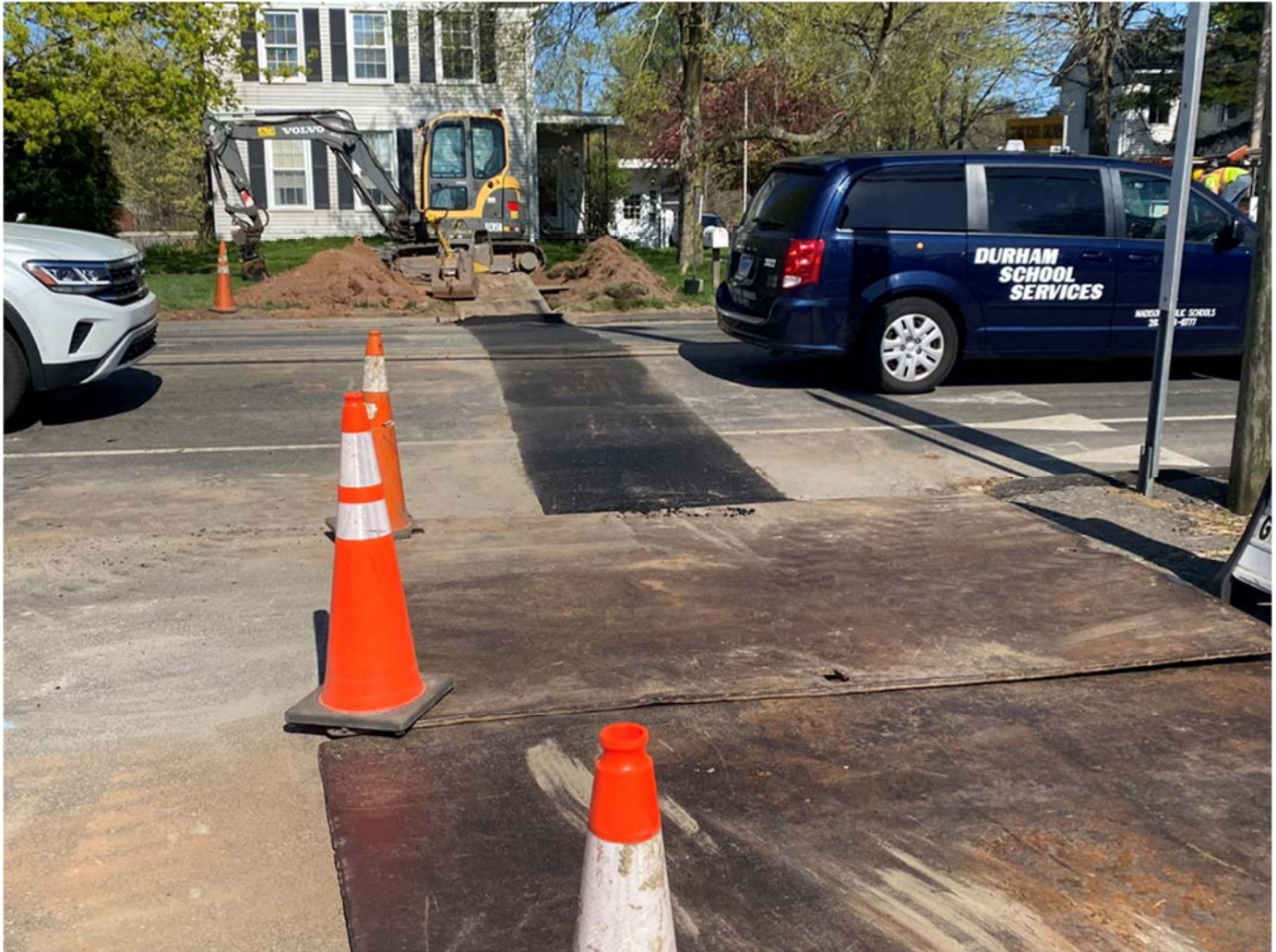
Picture 4: Road plates are placed over the open trenches, one just past the curb on the eastern side of the street over the trench in front of residence #55 Main Street, and the other plate is placed over the trench on the western side of the street just past the curb in front of 46 Main Street. Temporary asphalt is placed in 2 x 2" lifts between plates. View to the east.
