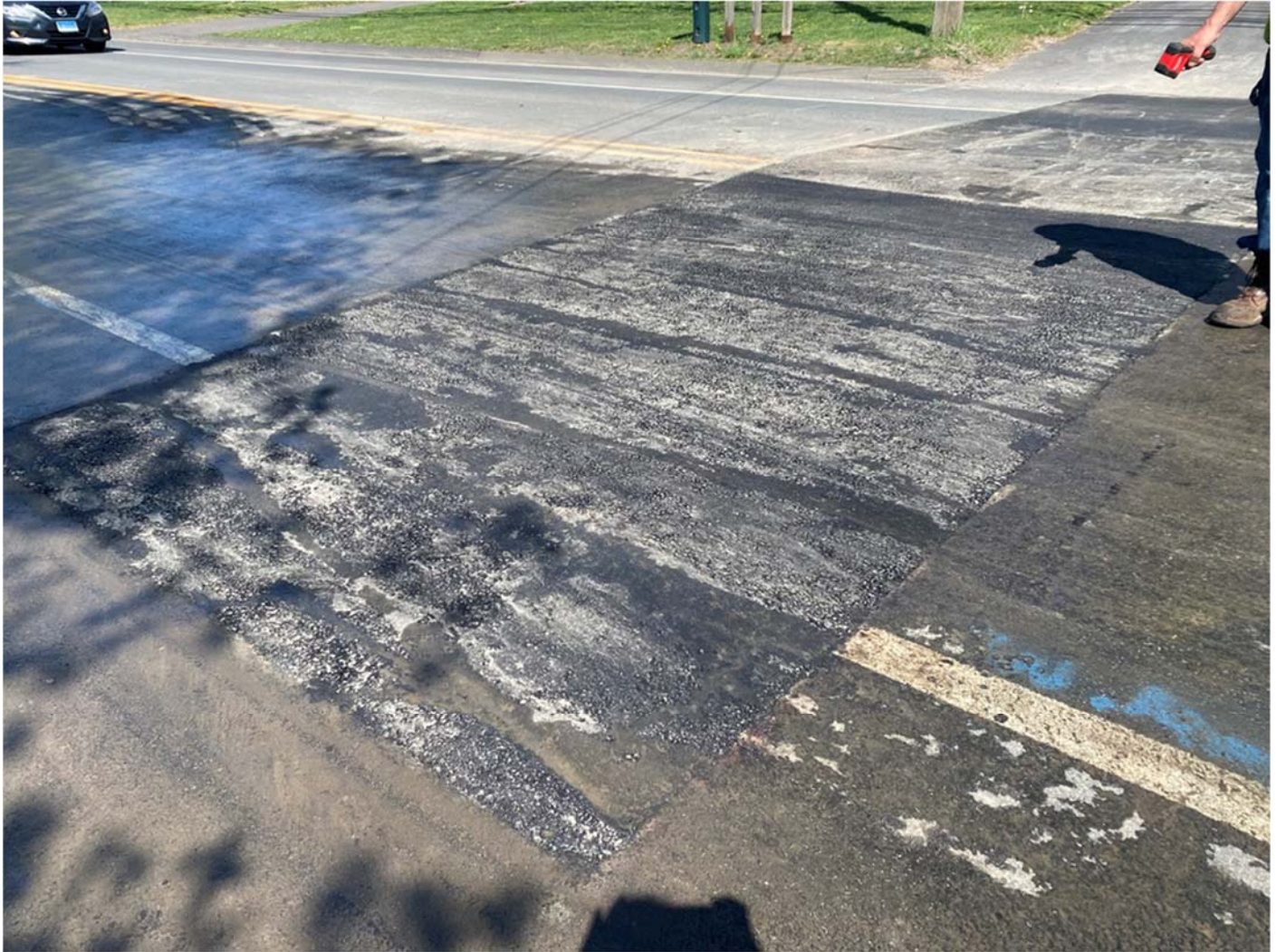
Picture 3: Asphalt is placed in 3 x 3" lifts
