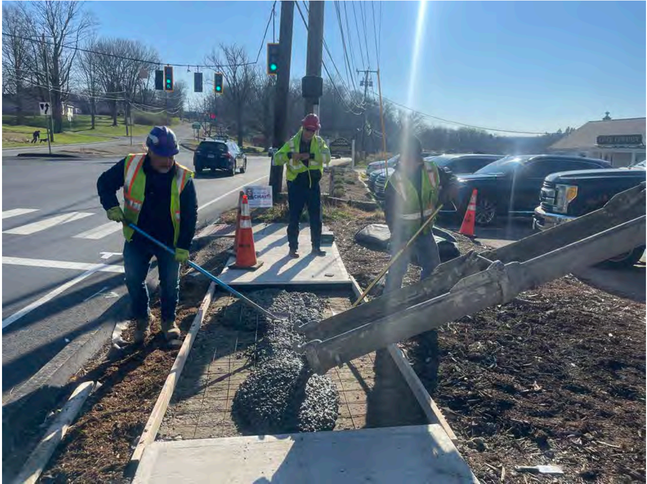
Picture 11: Ludlow assisting in the placement of the concrete being placed by Farmington Ready Mix in one of two forms they built to repair the sidewalk located on the east side of the 6 Main Street, Durham, property. View to the south.
