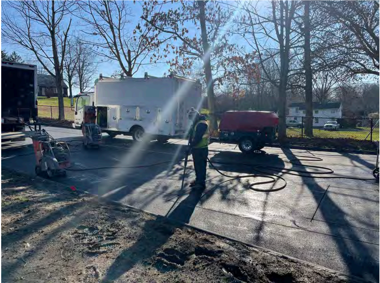
Picture 4: K.T.M using pressurized air to clean out the cuts they made in the pavement on Pickett Lane for the installation of traffic loops between Stations 10+00 and ~10+50. View to the southeast.
