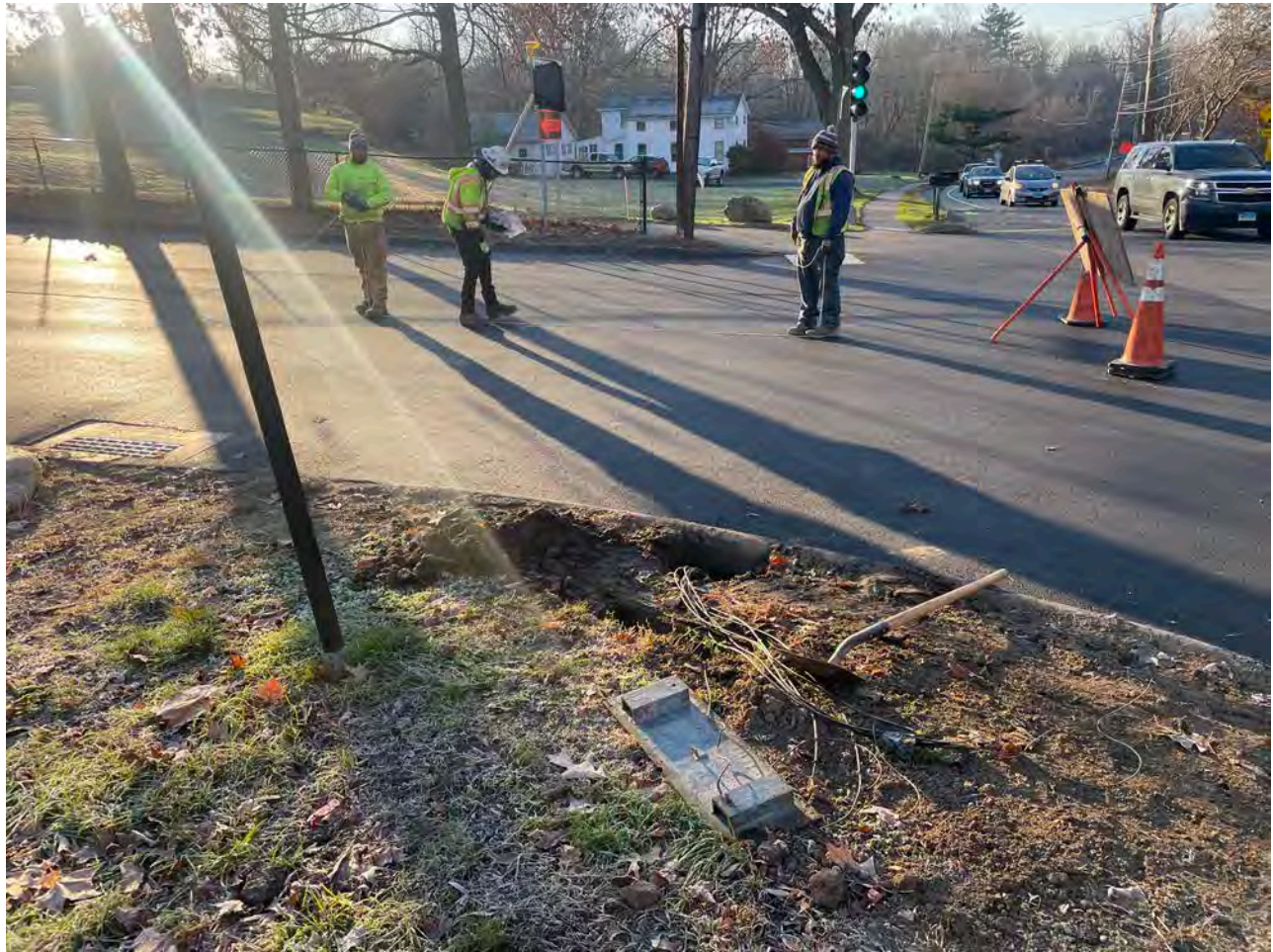
Picture 1: K.T.M laying out the locations of traffic loops on Pickett Lane between Stations 10+00 and ~10+50. View to the south.
