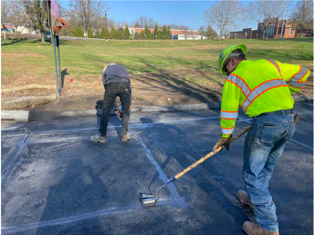
Picture 7: K.T.M leveling the sealant over the loop wire they placed in the cuts they made in the pavement on Pickett Lane for the installation of traffic loops between Stations 10+00 and ~10+50. View to the north.
