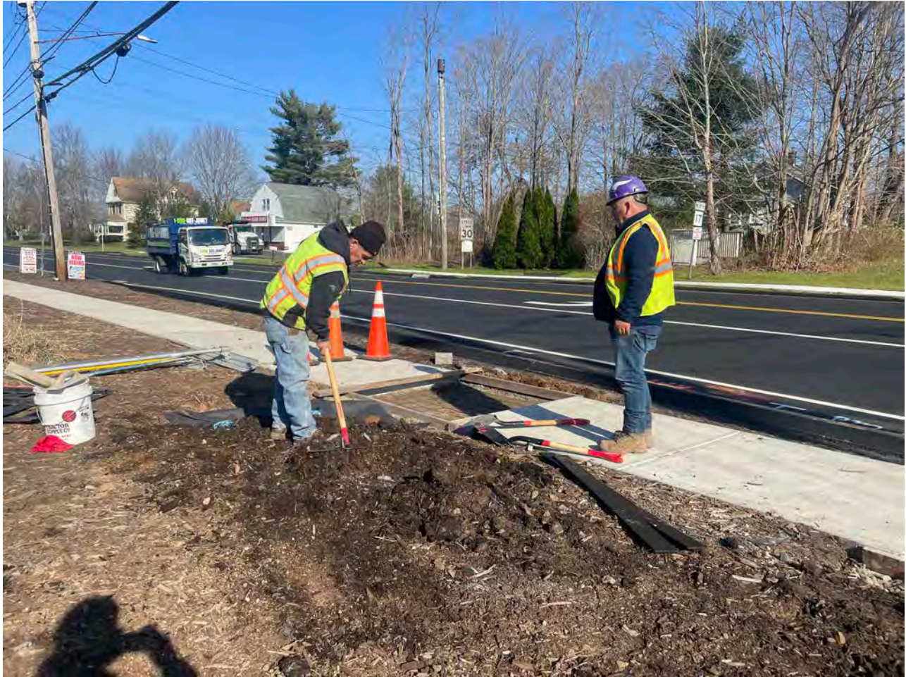
Picture 10: Ludlow restoring the mulch bed located on the west side of the sidewalk they are repairing on the east side of the 6 Main Street, Durham, property. View to the northeast.
