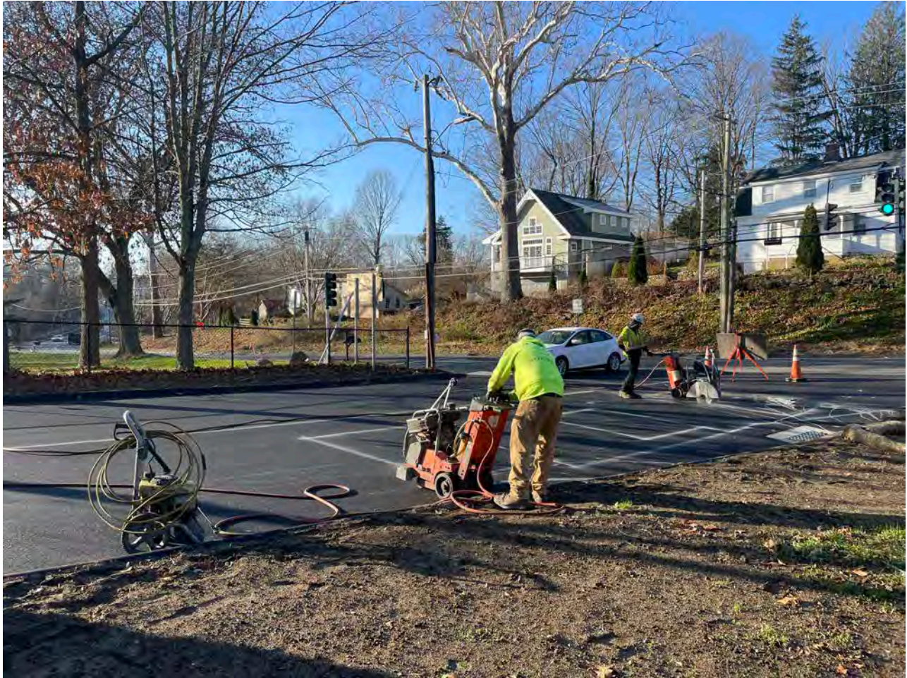
Picture 2: K.T.M saw-cutting pavement on the westbound lane of Pickett Lane for the installation of traffic loops between Stations 10+00 and ~10+50. View to the southwest.
