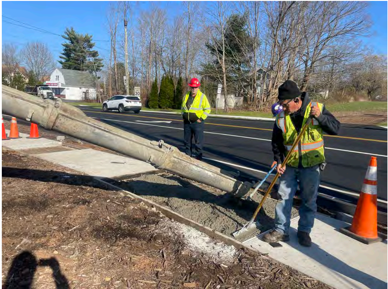
Picture 12: Ludlow assisting in the placement of the concrete being placed by Farmington Ready Mix in one of two forms they built to repair the sidewalk located on the east side of the 6 Main Street, Durham, property. View to the northeast.
