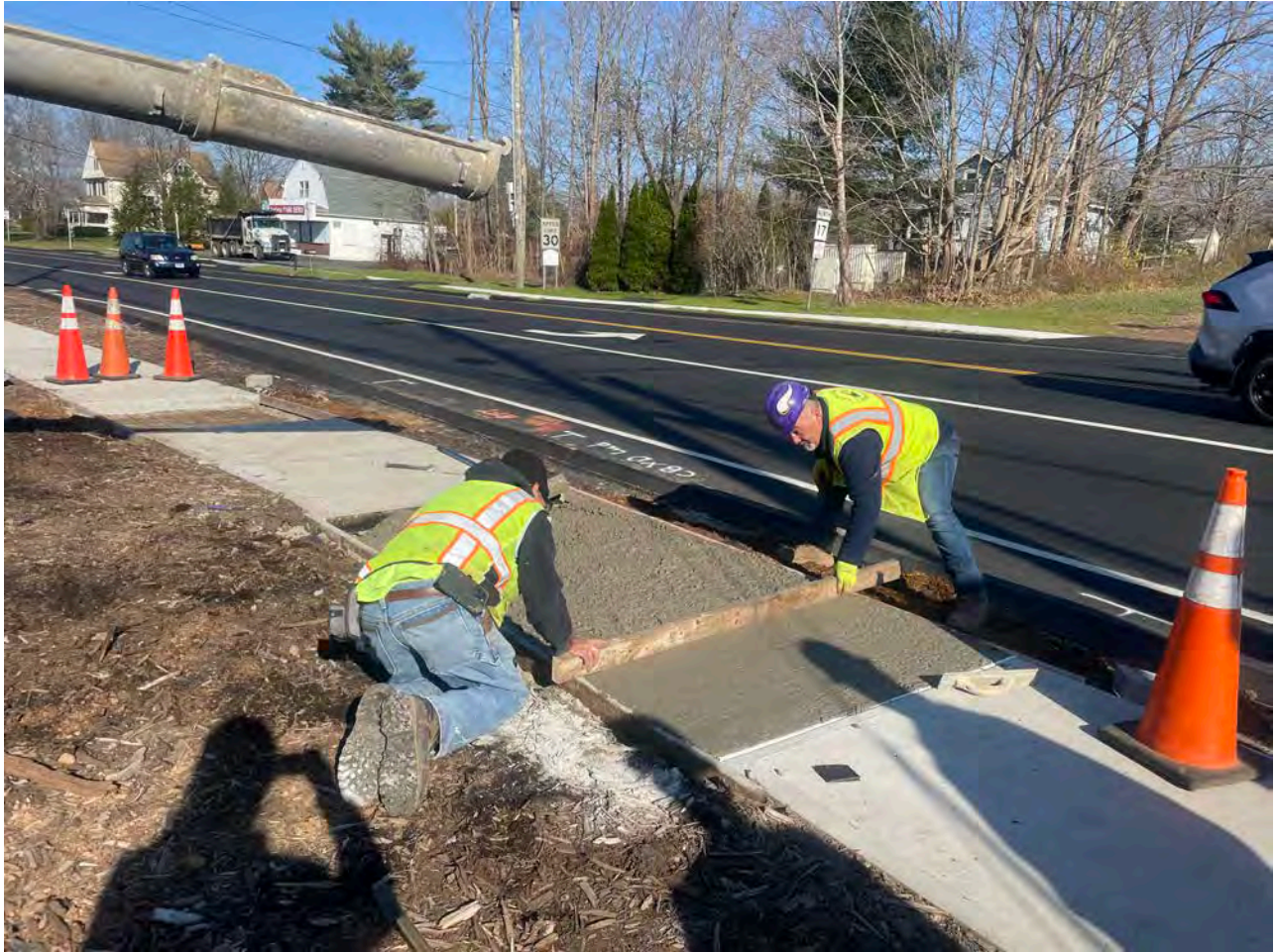
Picture 13: Ludlow leveling concrete being placed by Farmington Ready Mix in one of two forms they built to repair the sidewalk located on the east side of the 6 Main Street, Durham, property. View to the northeast.
