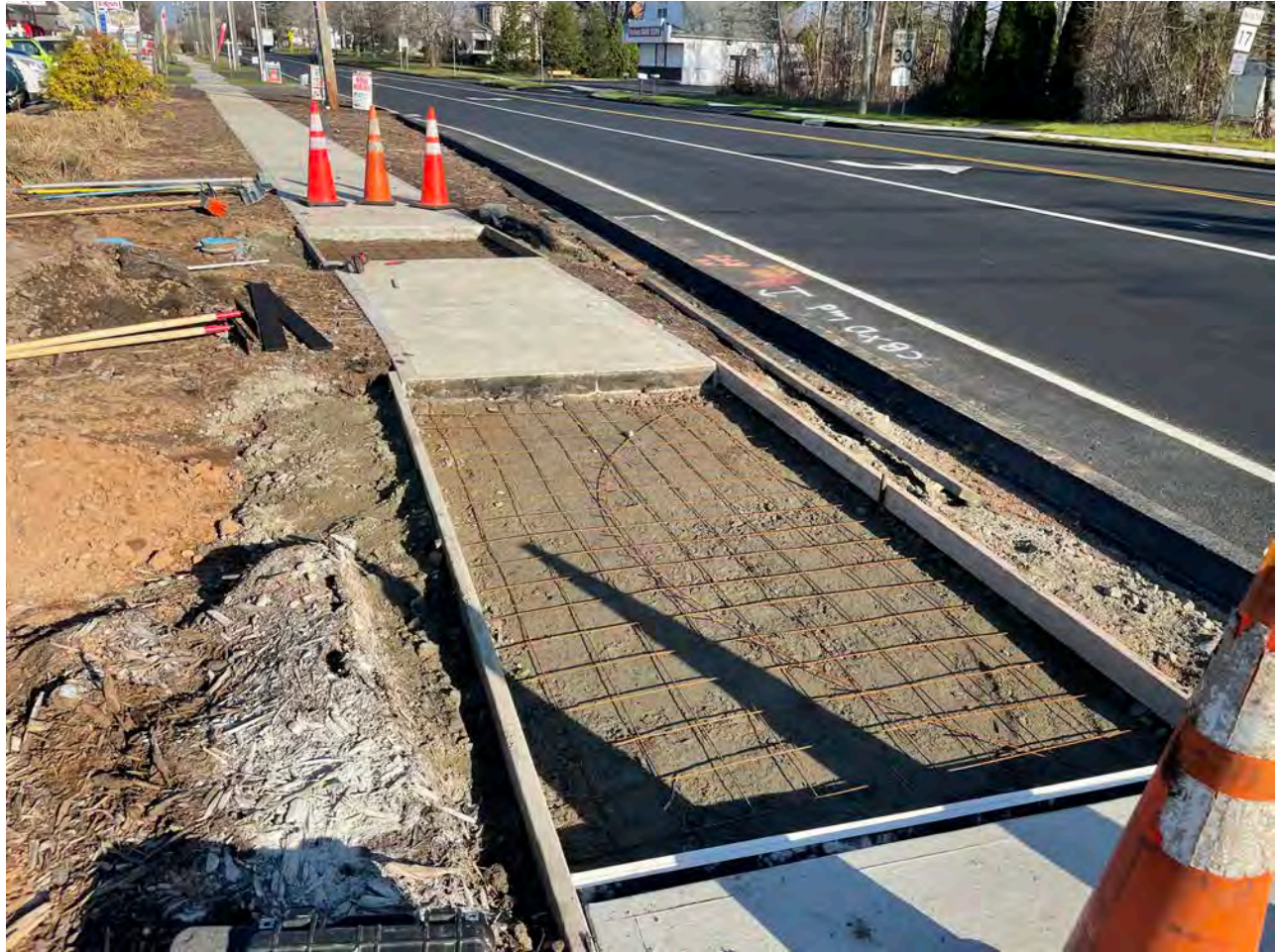
Picture 8: Section of sidewalk that Ludlow has framed up to receive a pour of 4000 PSI concrete as part of repair activities on the east side of the 6 Main Street, Durham, property. View to the northeast.
