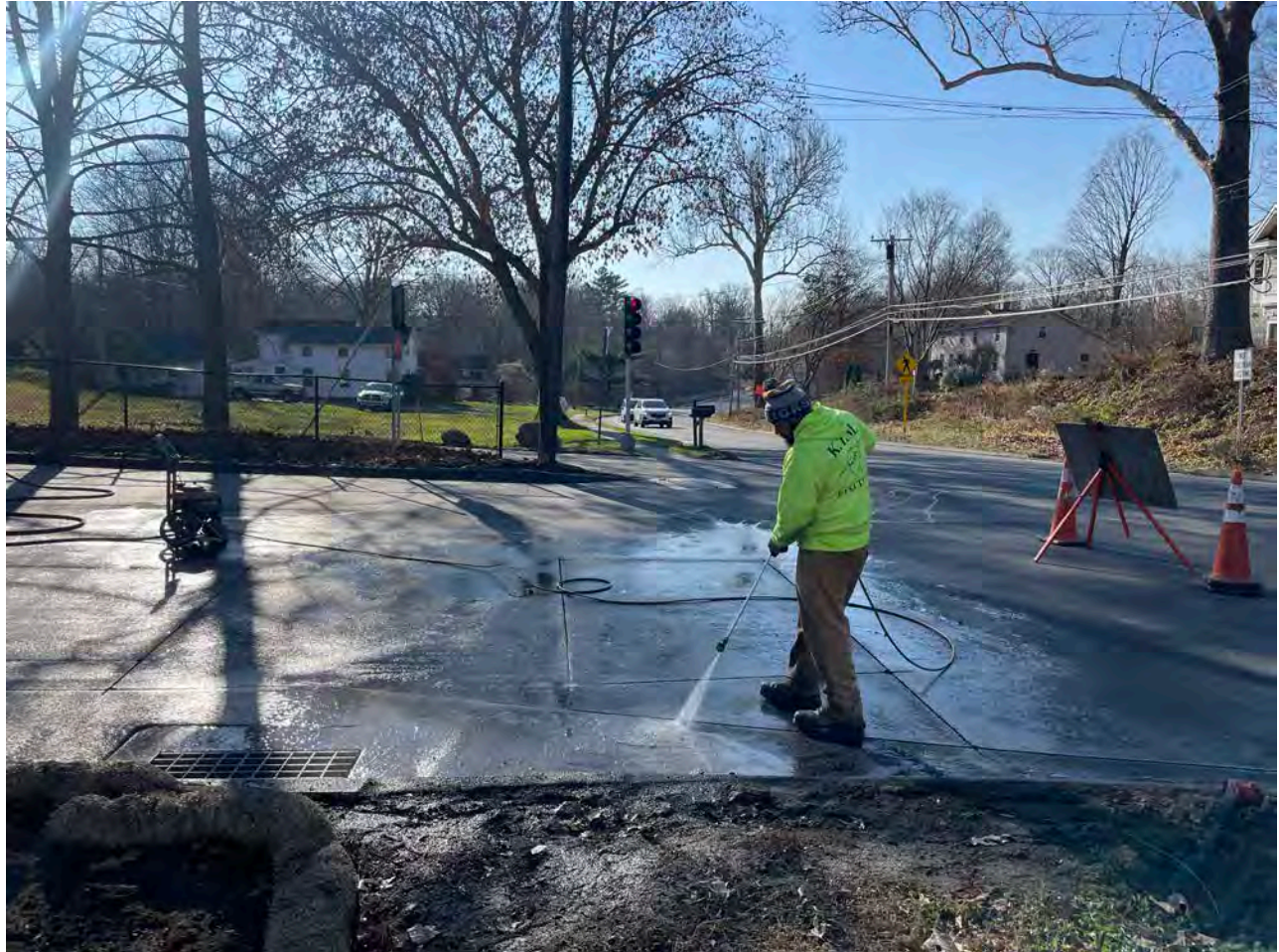
Picture 3: K.T.M using pressurized water to clean out the cuts they made in the pavement on Pickett Lane for the installation of traffic loops between Stations 10+00 and ~10+50. View to the south.
