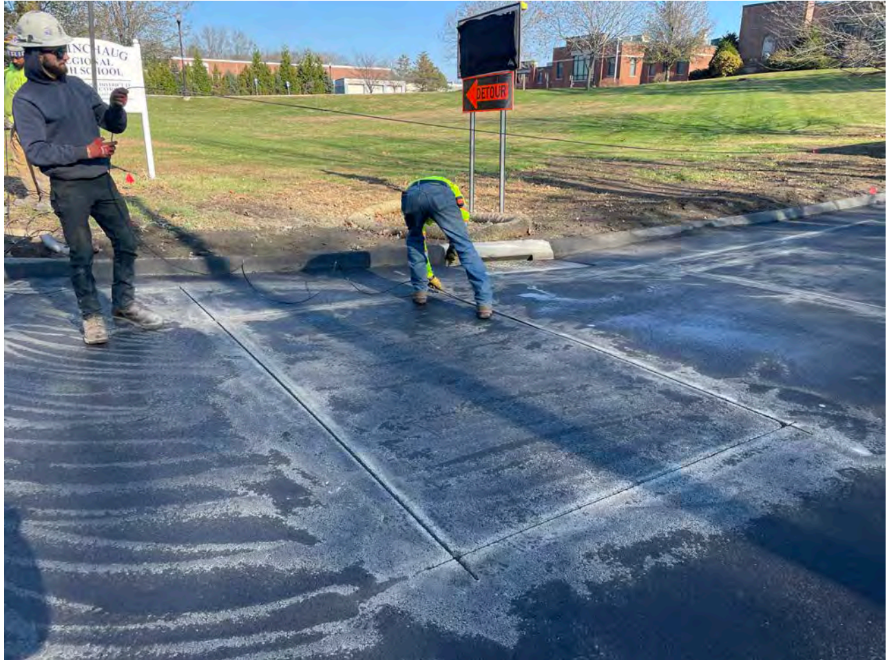
Picture 5: K.T.M installing loop wire in the cuts they made in the pavement on Pickett Lane for the installation of traffic loops between Stations 10+00 and ~10+50. View to the northeast.
