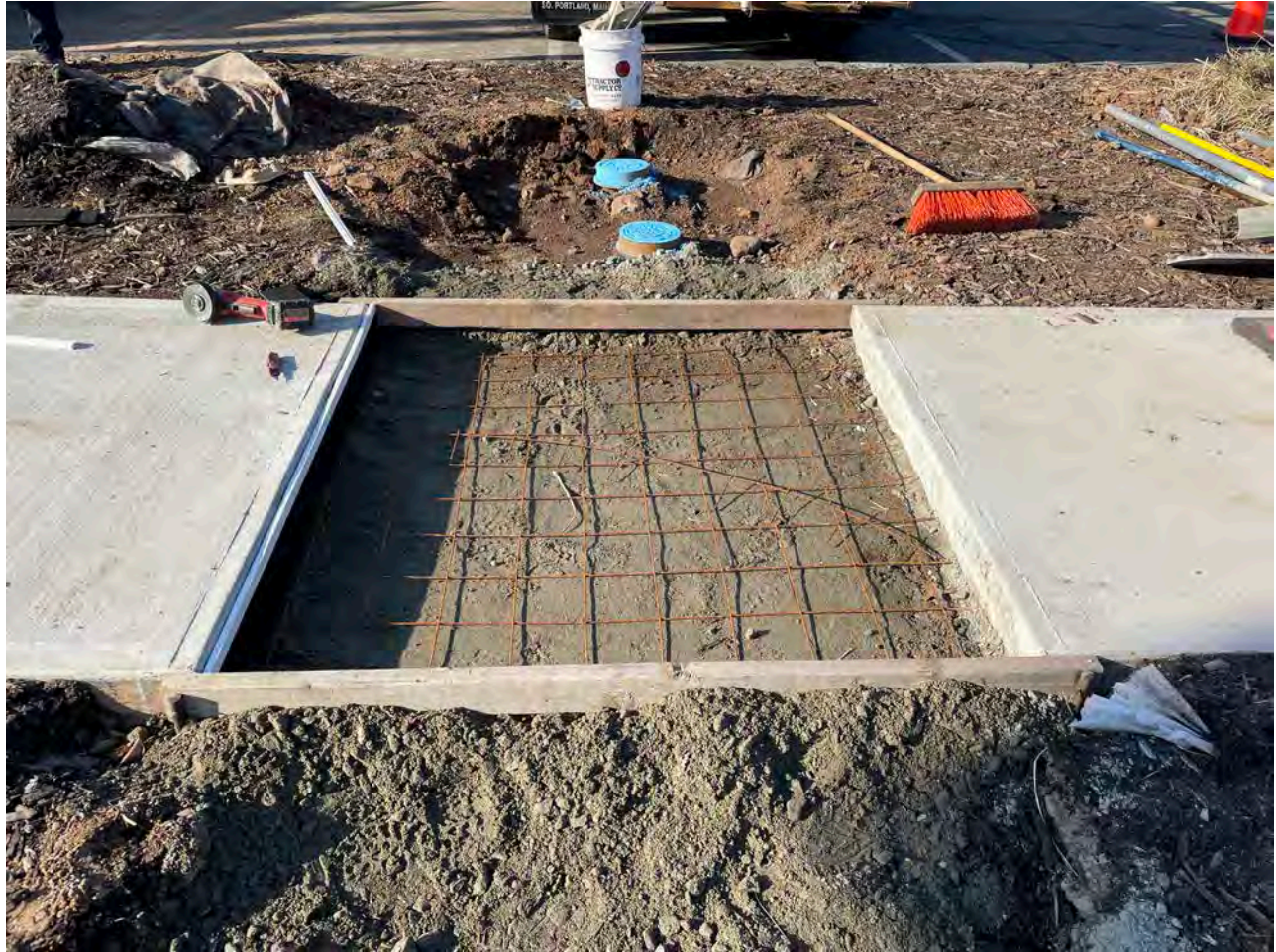
Picture 9: Section of sidewalk that Ludlow has framed and has placed a sheet of steel 4" x4" screen before filling with 4000 PSI concrete on the east side of the 6 Main Street, Durham, property. View to the west.
