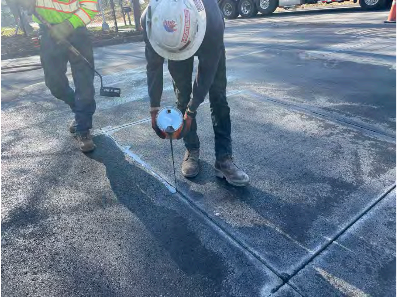
Picture 6: K.T.M placing sealant over the loop wire they placed in the cuts they made in the pavement on Pickett Lane for the installation of traffic loops between Stations 10+00 and ~10+50. View to the southwest.
