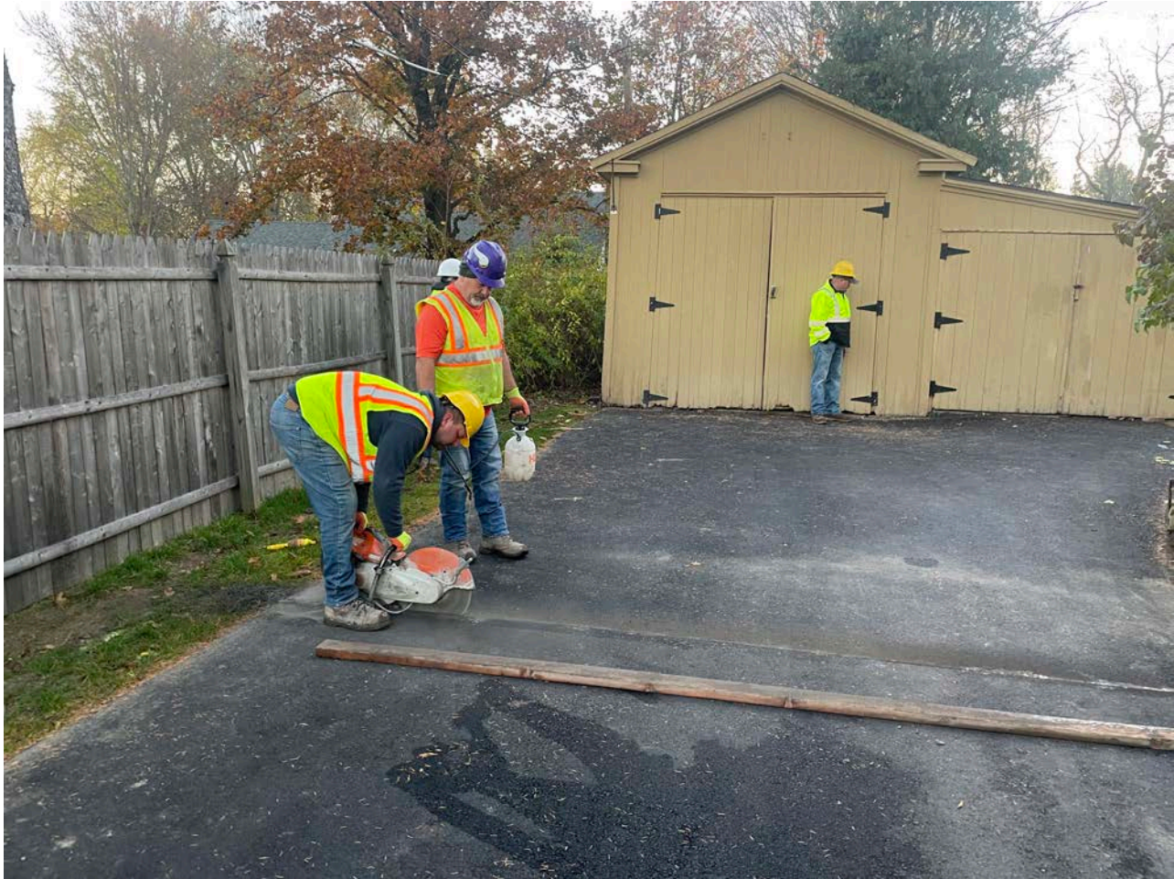
Picture 1: Ludlow saw-cutting across the driveway at the 257 Main Street, Durham, property as they prepare to replace a section of the pavement. View to the east.
