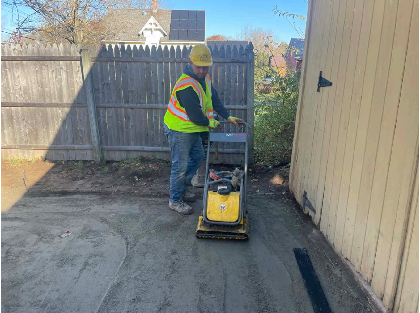
Picture 5: Ludlow compacting 1.25" processed gravel on the east side of the driveway located at the 257 Main Street, Durham, property with a plate compactor. View to the north.
