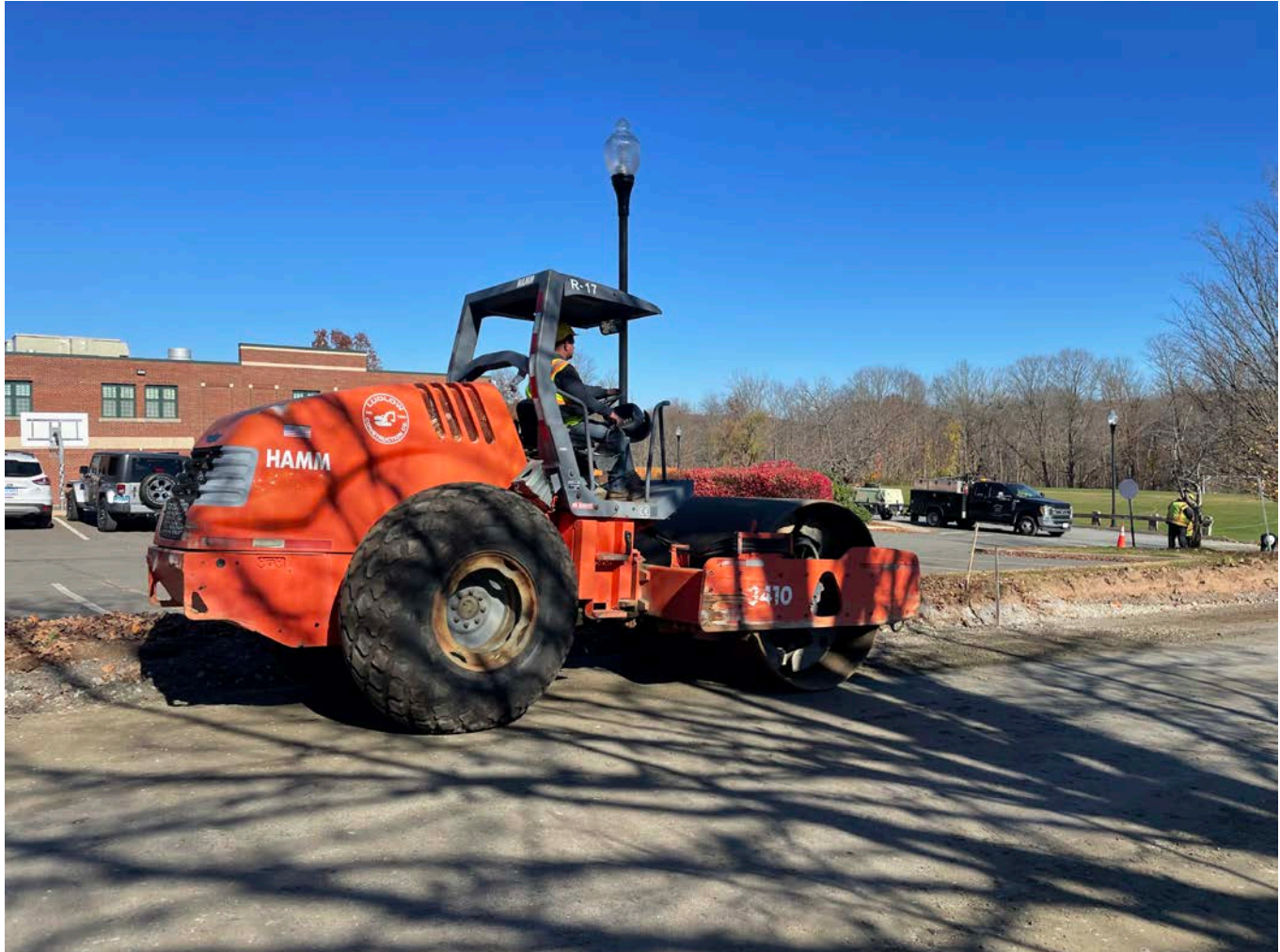
Picture 9: Ludlow compacting the 1.25" processed gravel that they placed between Stations 10+00 and 18+13. View to the northeast.
