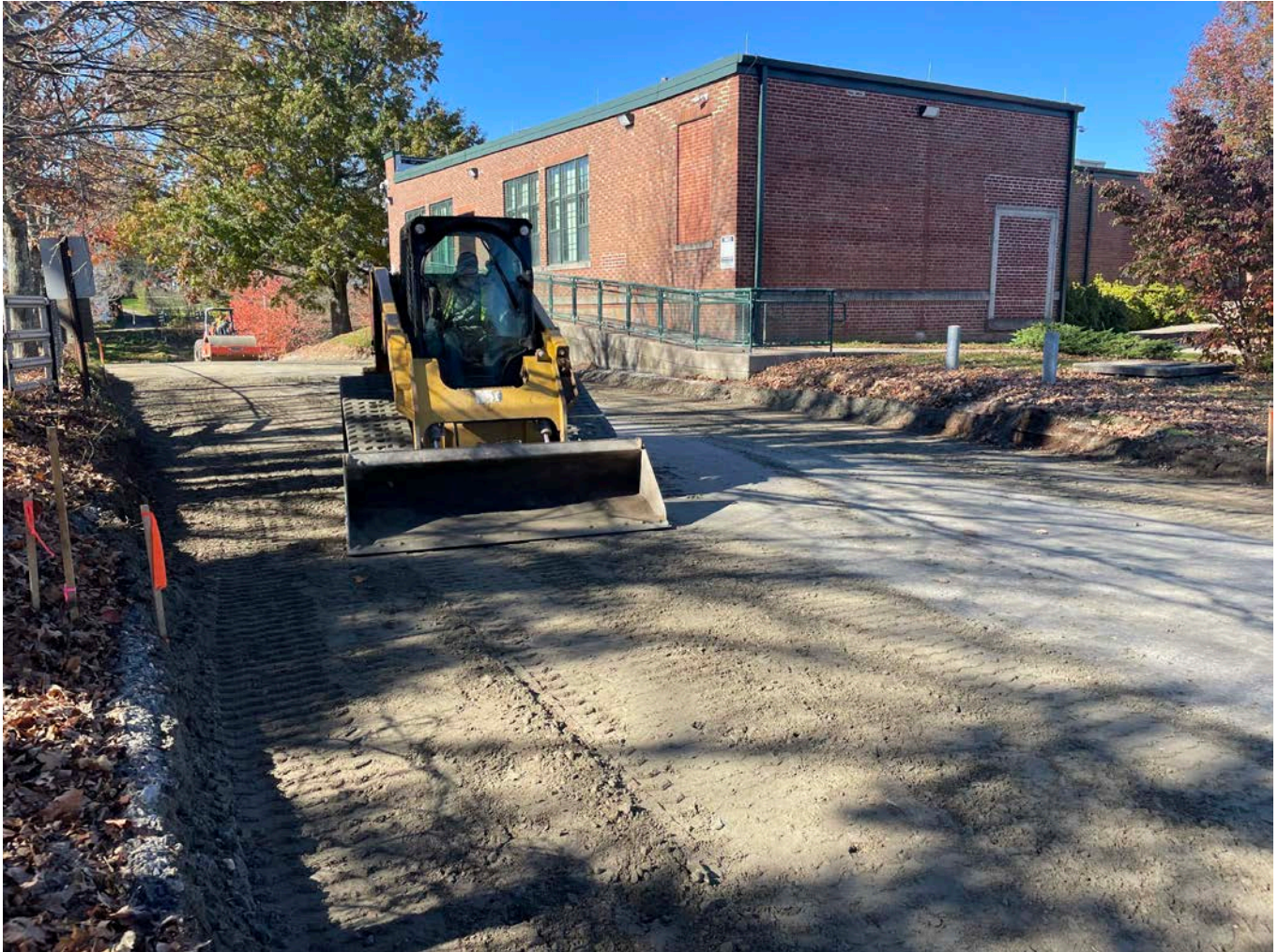
Picture 7: Ludlow grading the 1.25" processed gravel that they placed between Stations 10+00 and 18+13. View to the west.
