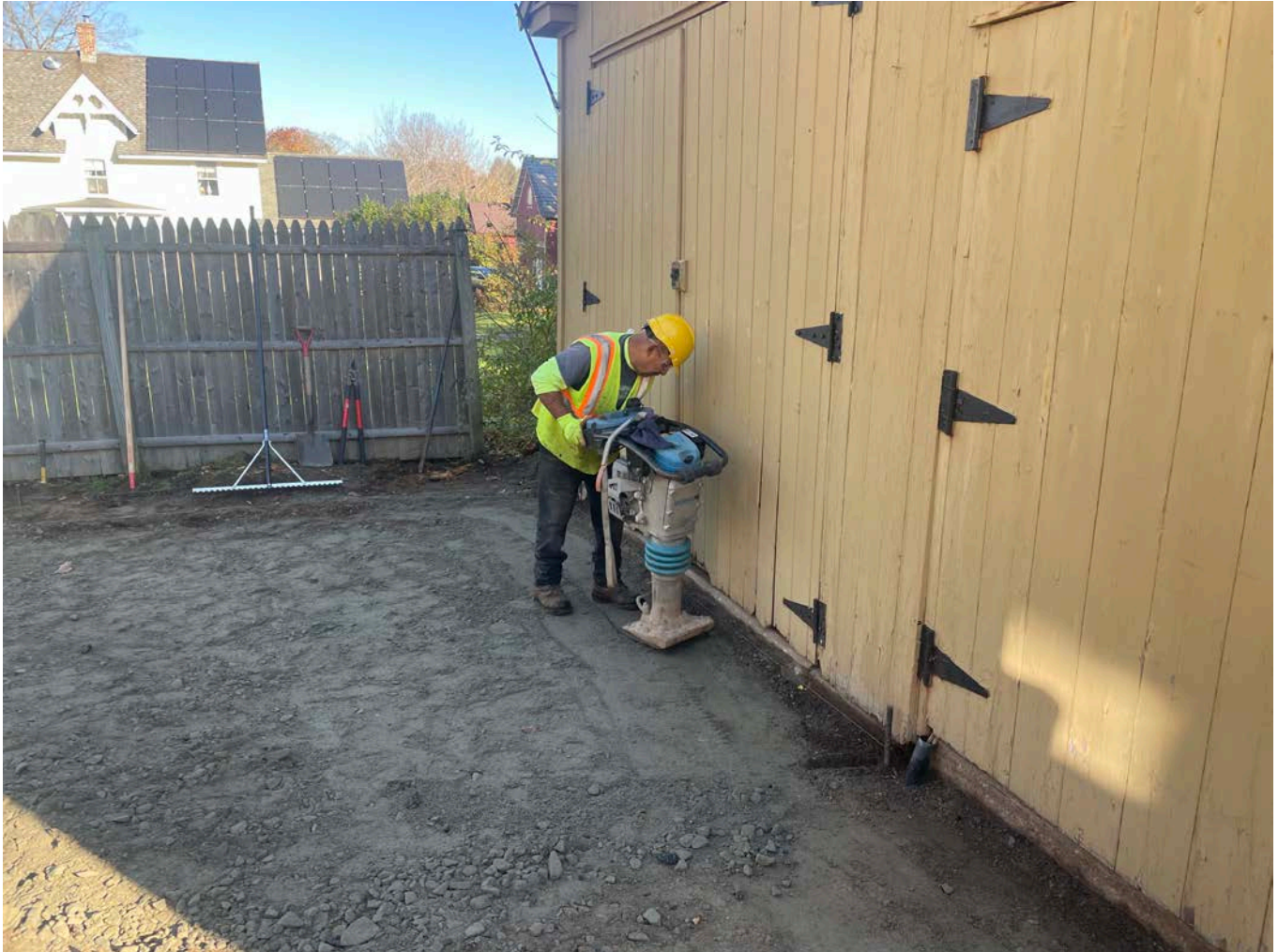
Picture 4: Ludlow compacting 1.25" processed gravel on the east side of the driveway located at the 257 Main Street, Durham, property with a jumping jack. View to the north.
