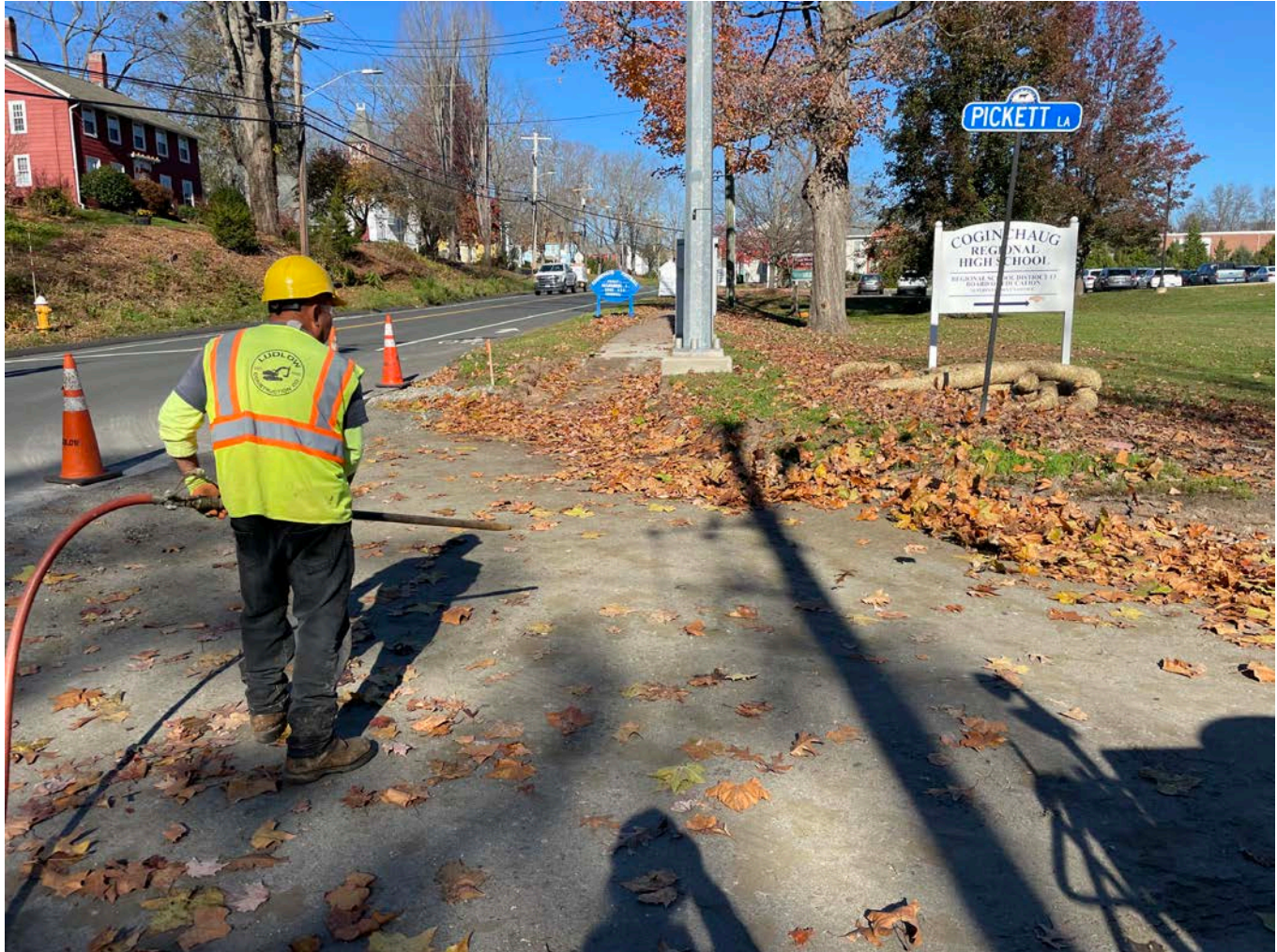
Picture 6: Ludlow using an air compressor to blow leaves off Pickett Lane prior to grading and compaction the 1.25" processed gravel that they placed between Stations 10+00 and 18+13. View to the north.
