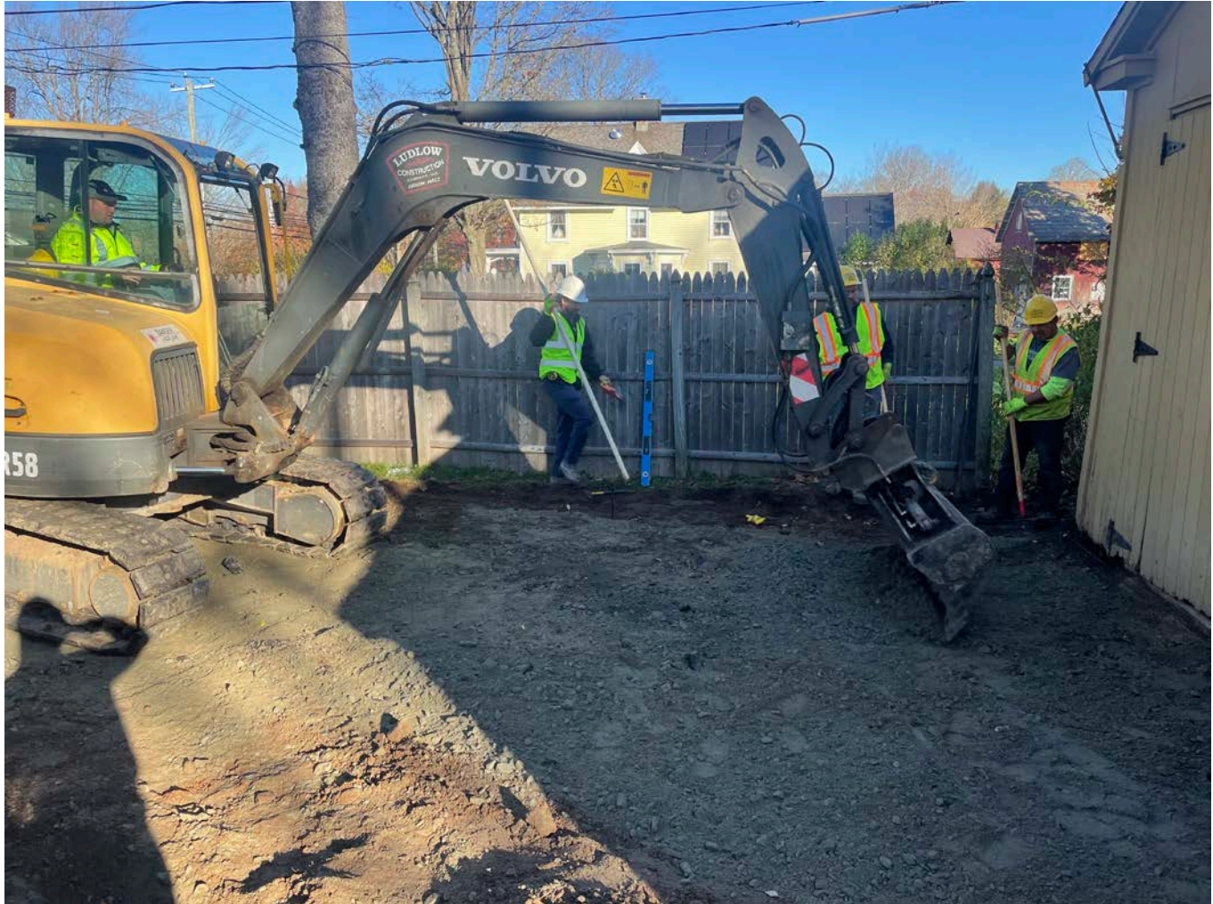
Picture 3: Ludlow placing 1.25" processed gravel on the east side of the driveway located at the 257 Main Street, Durham, property. View to the north.
