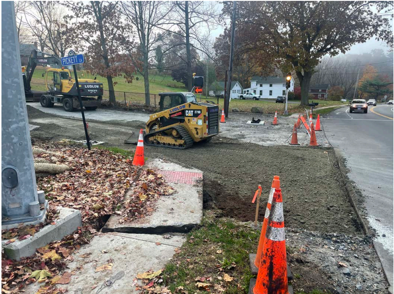
Picture 2: Ludlow grading the 1.25" processed gravel at Station ~10+20. Section of broken sidewalk in the foreground. View to the southeast.
