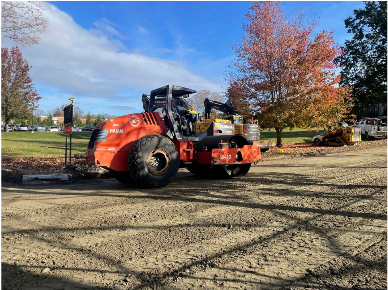
Picture 6: Ludlow compacting 1.25" processed gravel at Stations ~10+40 on Pickett Lane. View to the northeast.
