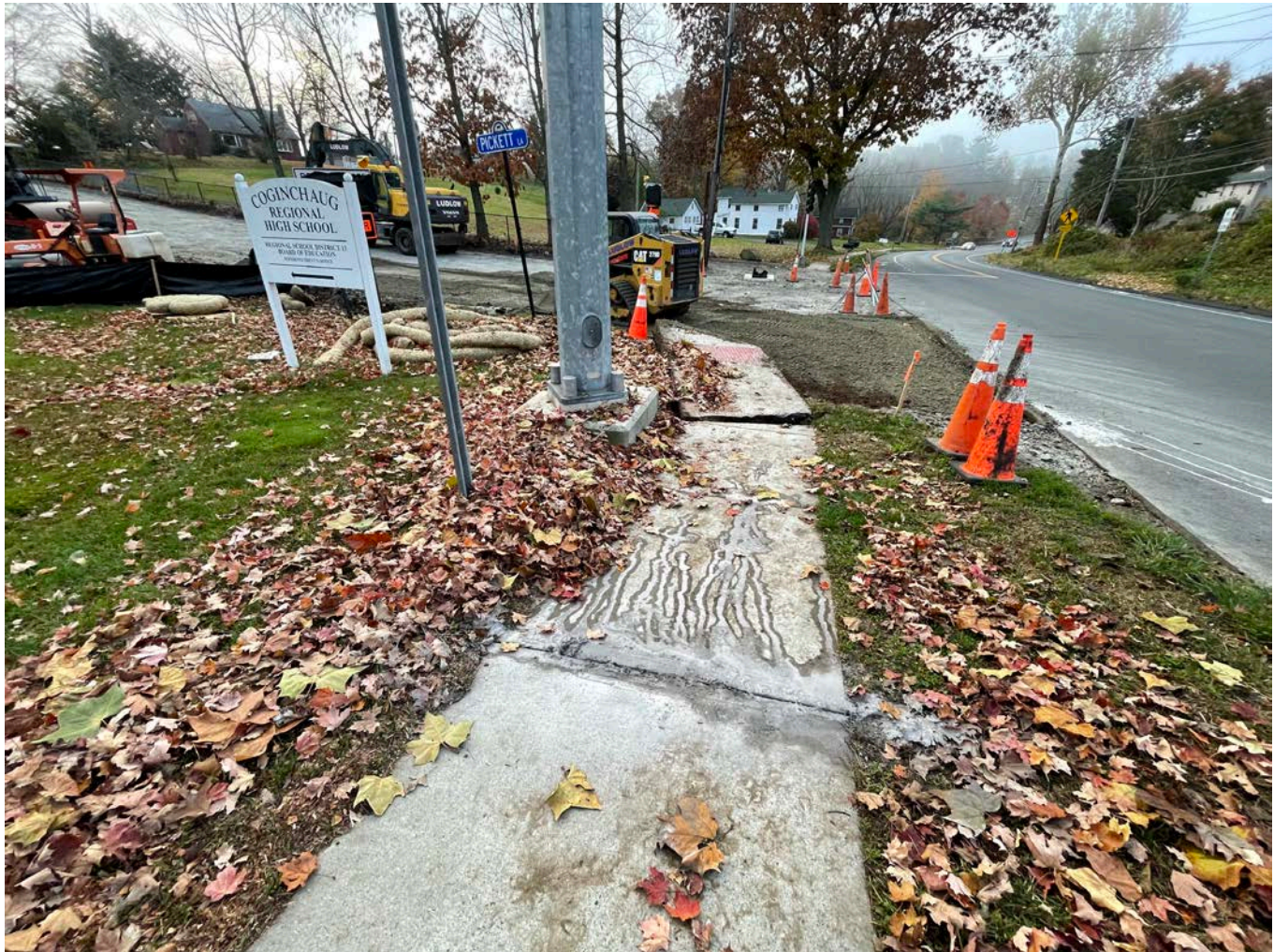
Picture 3: Section of concrete sidewalk that Ludlow cut several panels north of where a section of it broke at the intersection of Pickett Lane and Main Street. View to the south.
