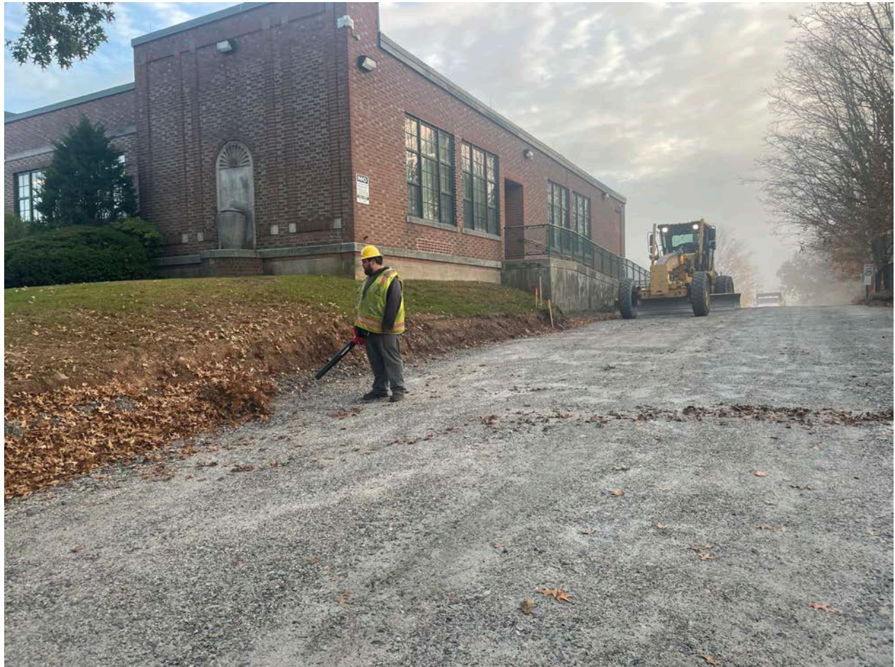
Picture 1: Ludlow using a leaf blower to move leaves off Pickett Lane before they grade and compact the 1.25" processed gravel they previously placed between Stations 10+00 and 18+13. View to the northeast.
