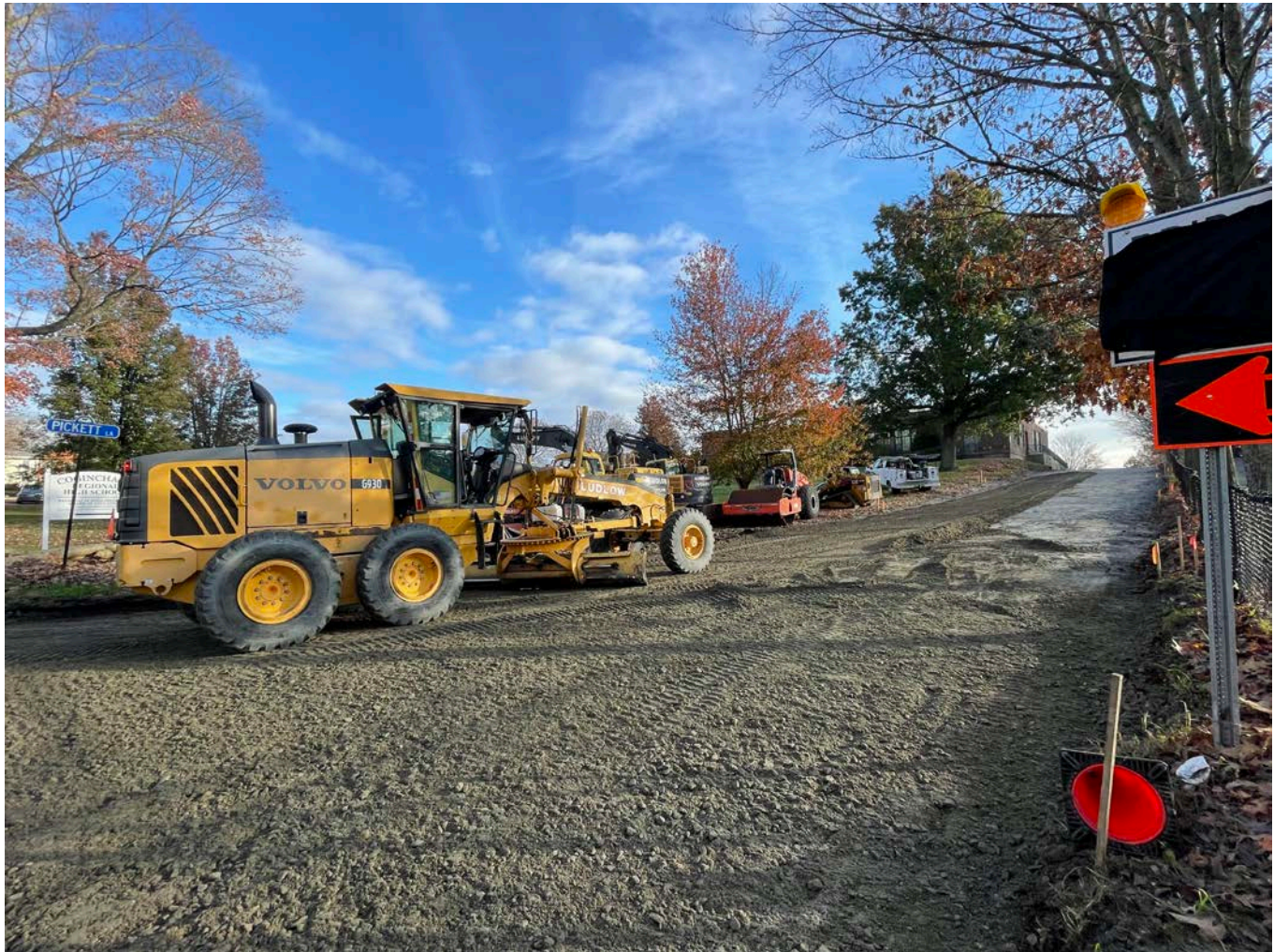
Picture 5: Ludlow grading 1.25" processed gravel at Stations 10+00 to ~12+00 on Pickett Lane. View to the east.
