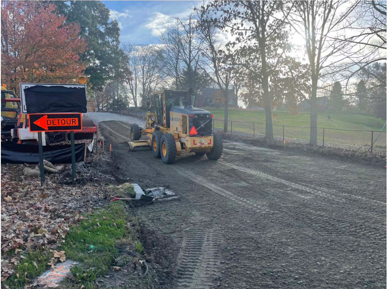
Picture 4: Ludlow grading 1.25" processed gravel at Stations ~11+50 on Pickett Lane. View to the southeast.
