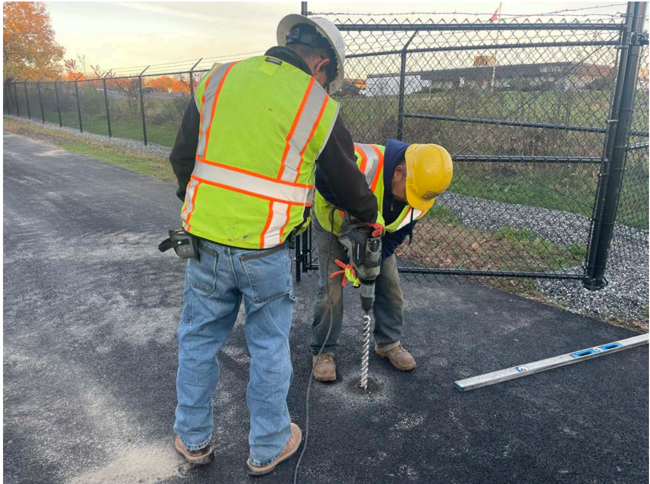
Picture 1: Ludlow drilling a hole in the pavement at the entrance to the Booster Station in order to install a stop post. View to the northwest.
