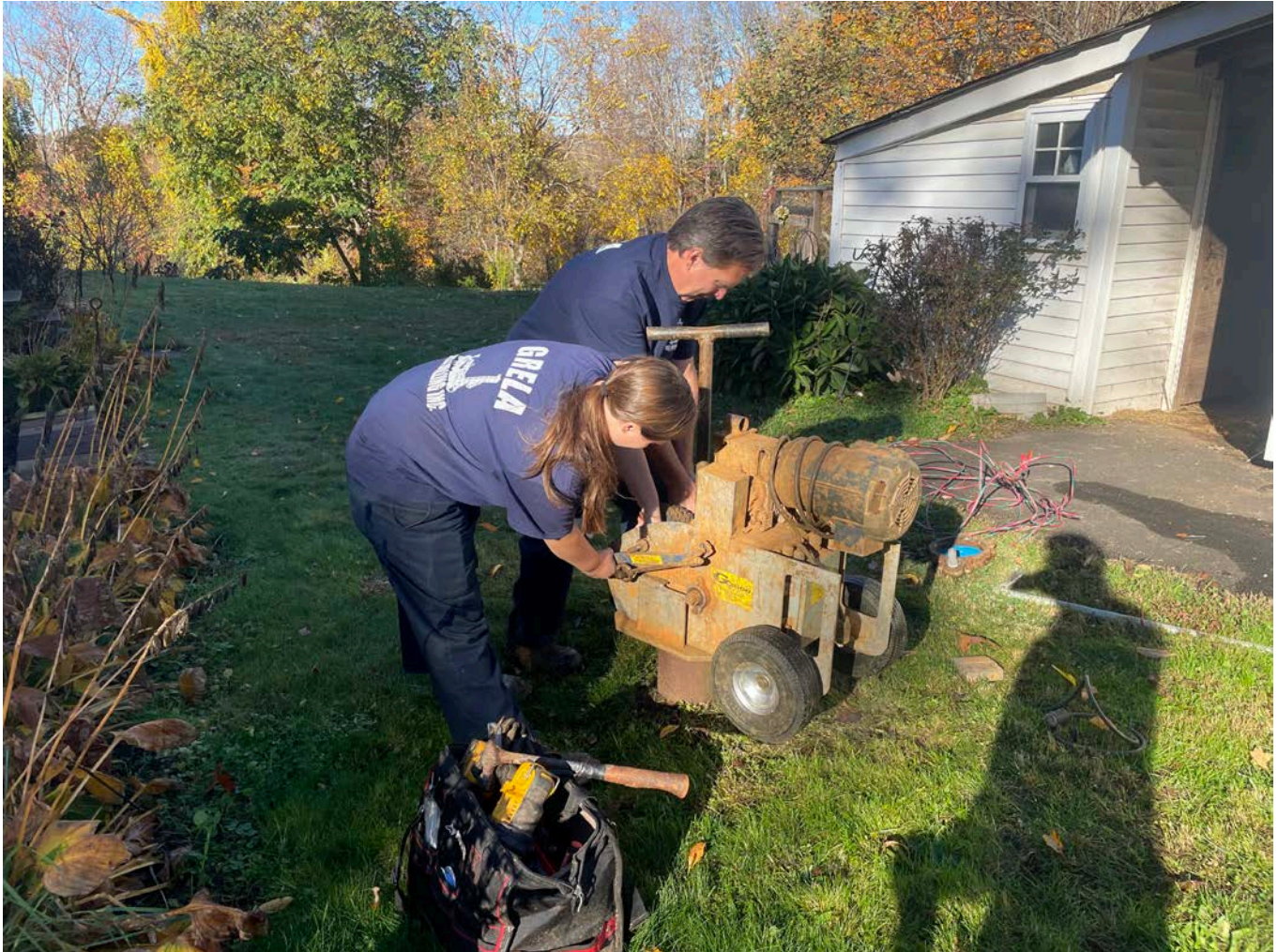
Picture 2: Grela setting up a pump puller on the well located on the northeast corner of the 228 Maple Avenue residence. View to the northwest.
