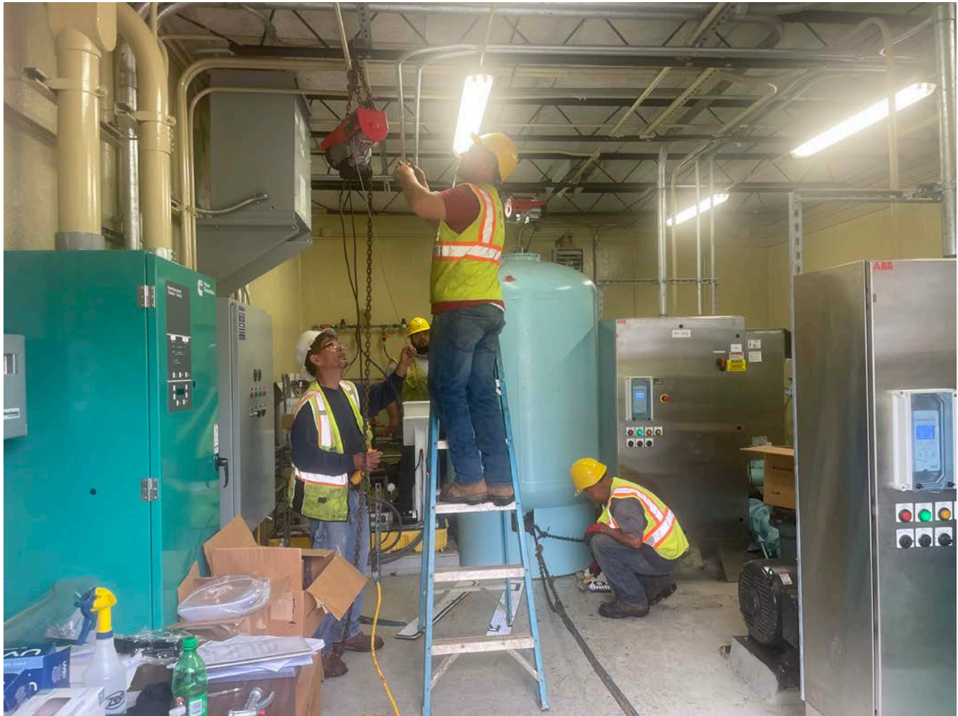
Picture 3: Ludlow connecting a second winch suspended from the ceiling of the Long Hill Pump Station to the expansion tank that they are in the process of removing today. View to the south.
