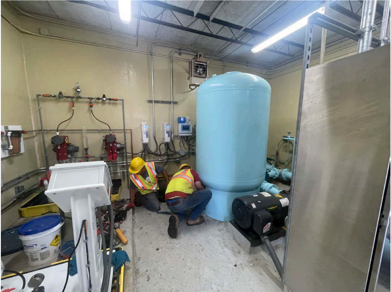
Picture 1: Ludlow draining the water from an expansion tank located on the south side of the Long Hill Pump Station located on Long Hill Road in Middletown. View to the south.
