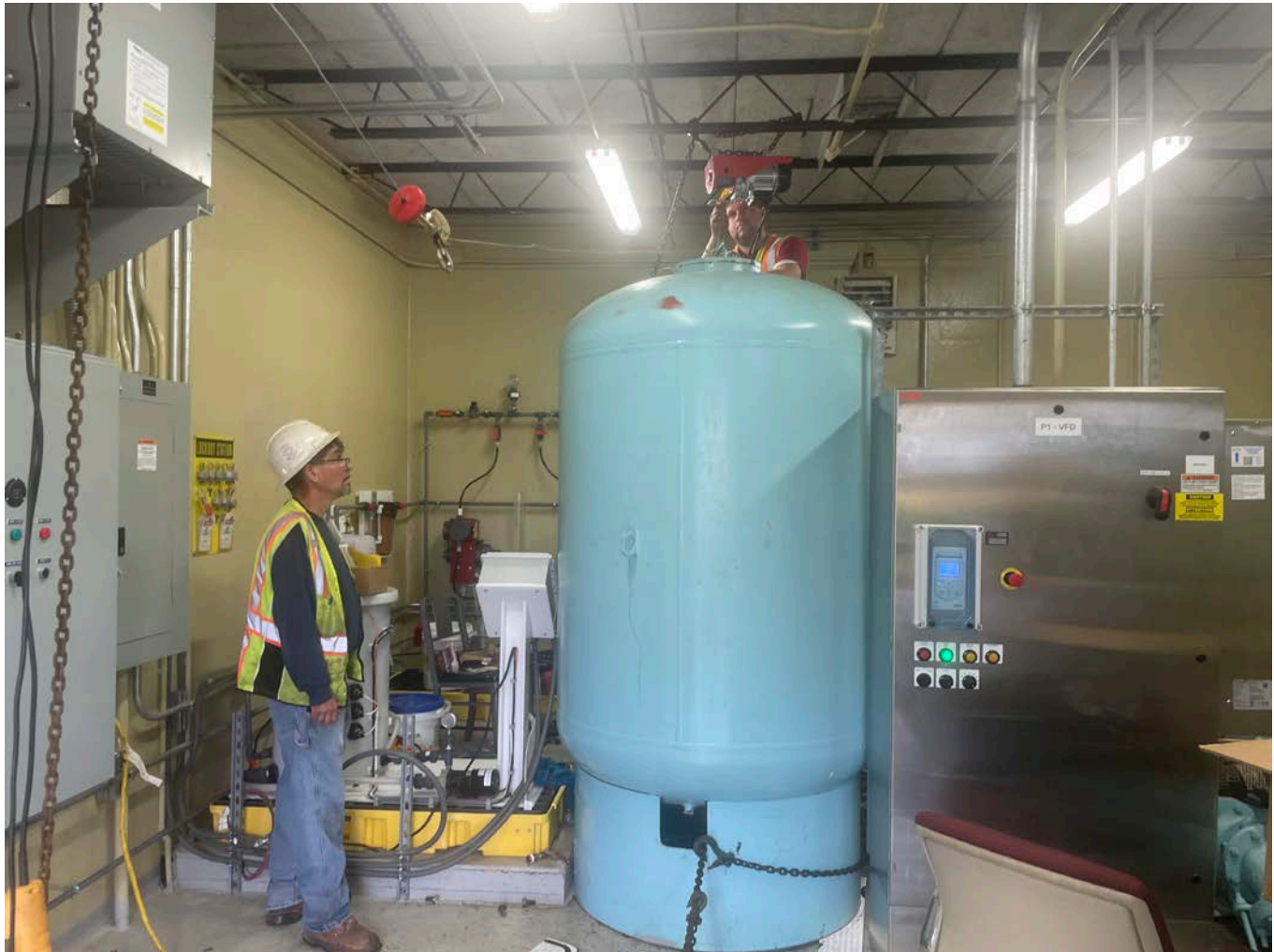
Picture 2: Ludlow connecting a winch suspended from the ceiling of the Long Hill Pump Station to the expansion tank that they are in the process of removing today. View to the south.
