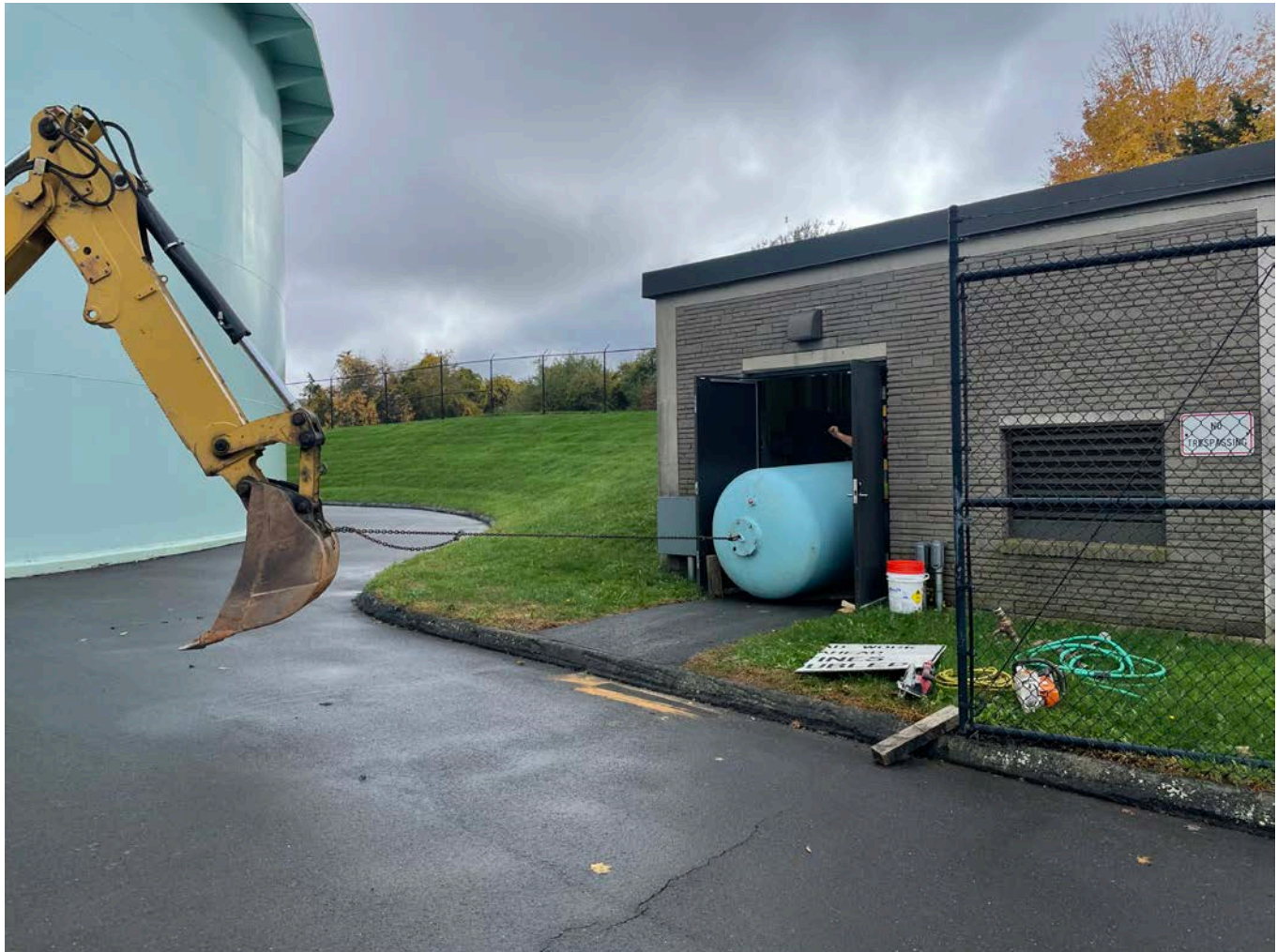
Picture 5: Ludlow using a back hoe to remove an expansion tank from the Long Hill Pump Station in Middletown. View to the southeast.
