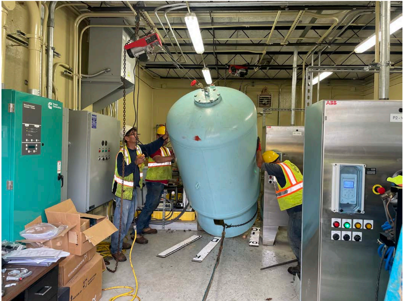
Picture 4: Ludlow in the process of removing an expansion tank from the Long Hill Pump Station in Middletown. View to the south.
