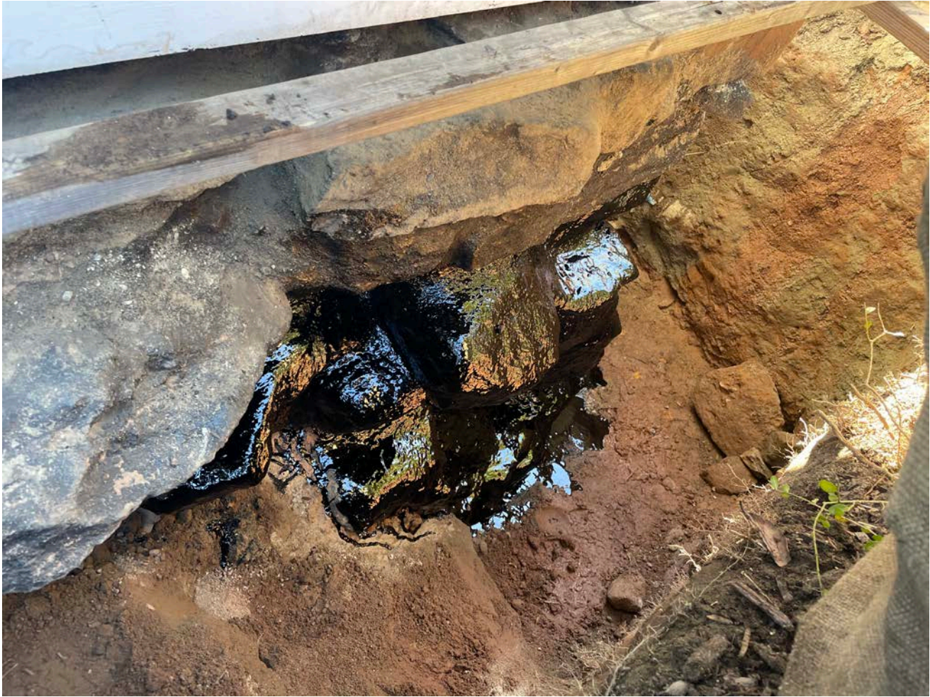
Picture 2: Foundation coating applied to the exterior of the foundation at 24 Maiden Lane, Durham
