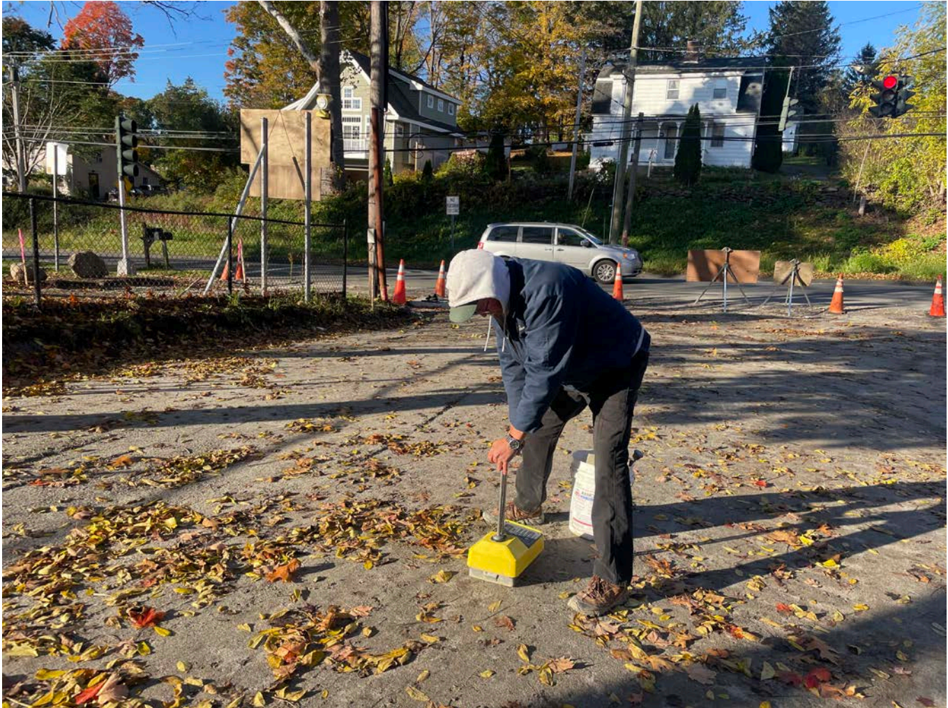
Picture 1: John Turner Consulting (JTC) on site performing compaction testing on the gravel base at Pickett Lane, Durham. View to the west.
