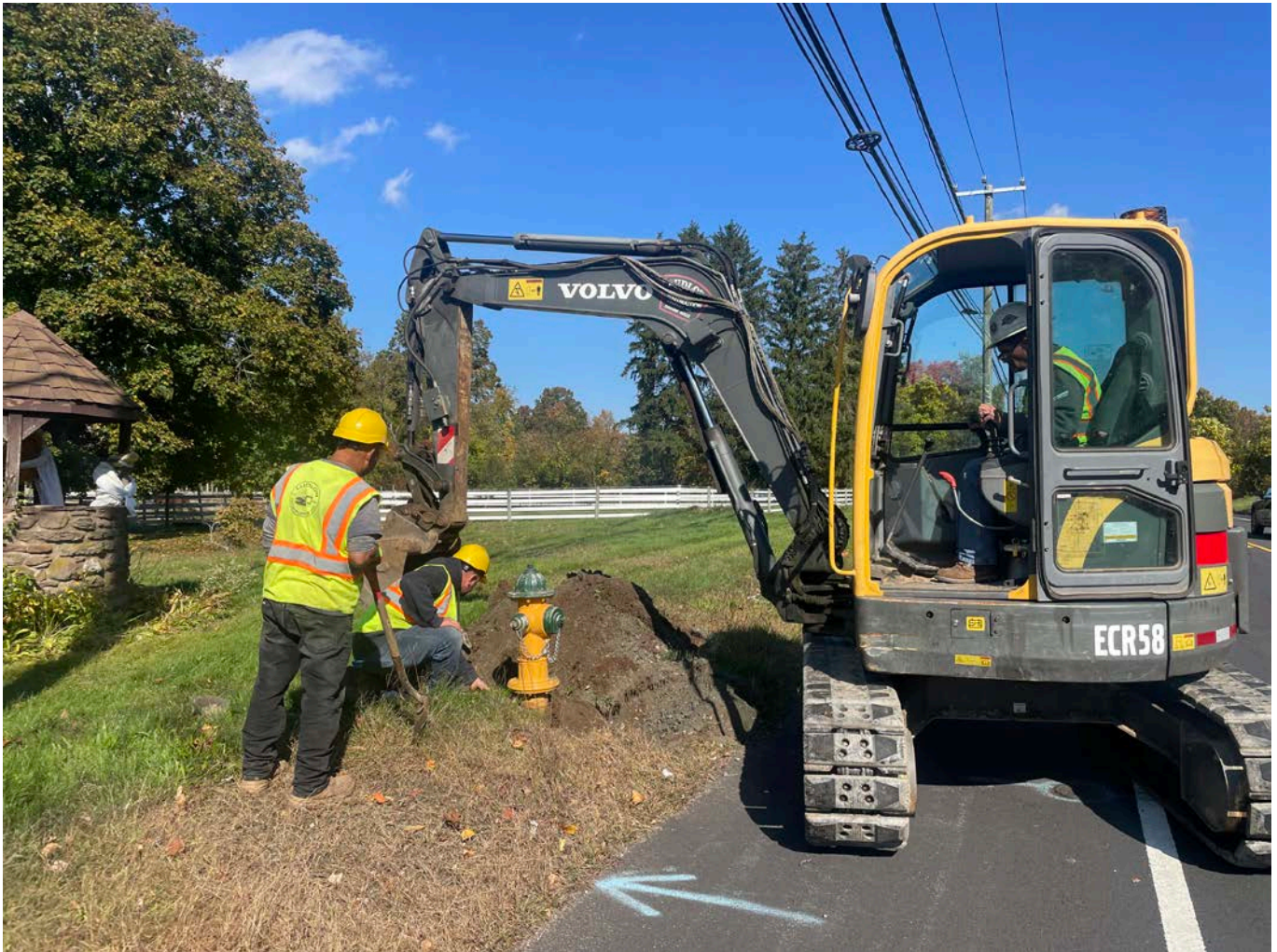
Picture 3: Ludlow realigning a hydrant located on the east side of the 2155 S. Main Street, Middletown. View to the north.
