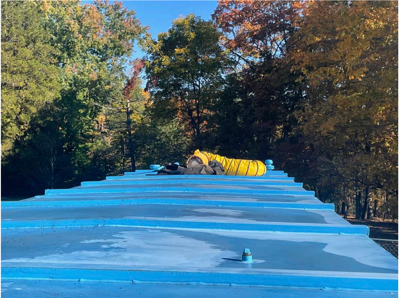
Picture 3: Fan that Ludlow placed on top of the frak tank located on the 281 Main Street, Durham, property in order to vent the tank prior to performing a confined space entry. View to the north.
