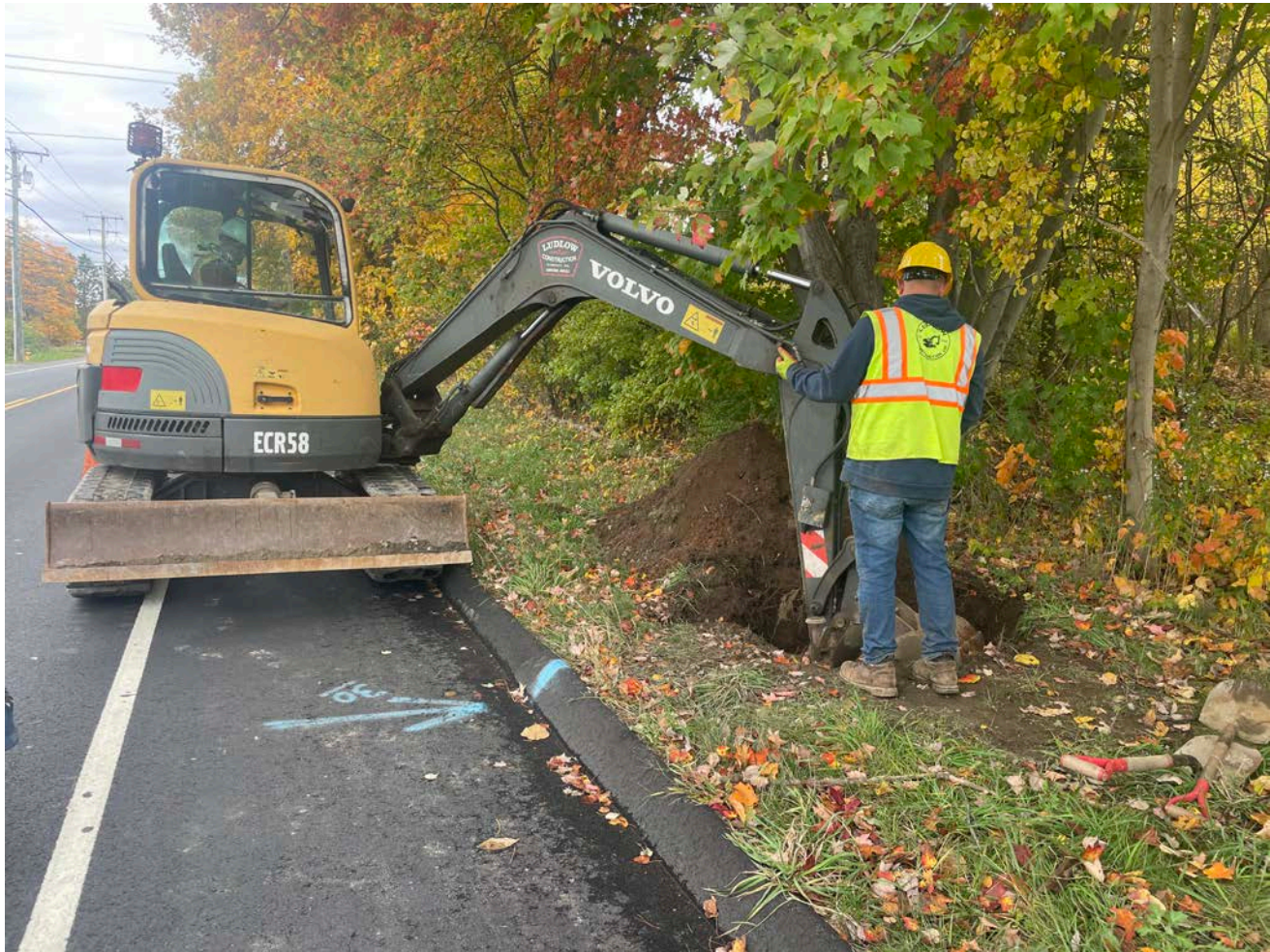
Picture 6: Ludlow replacing a curb box at the 2246-2266 S. Main Street, Middletown, property. View to the north.
