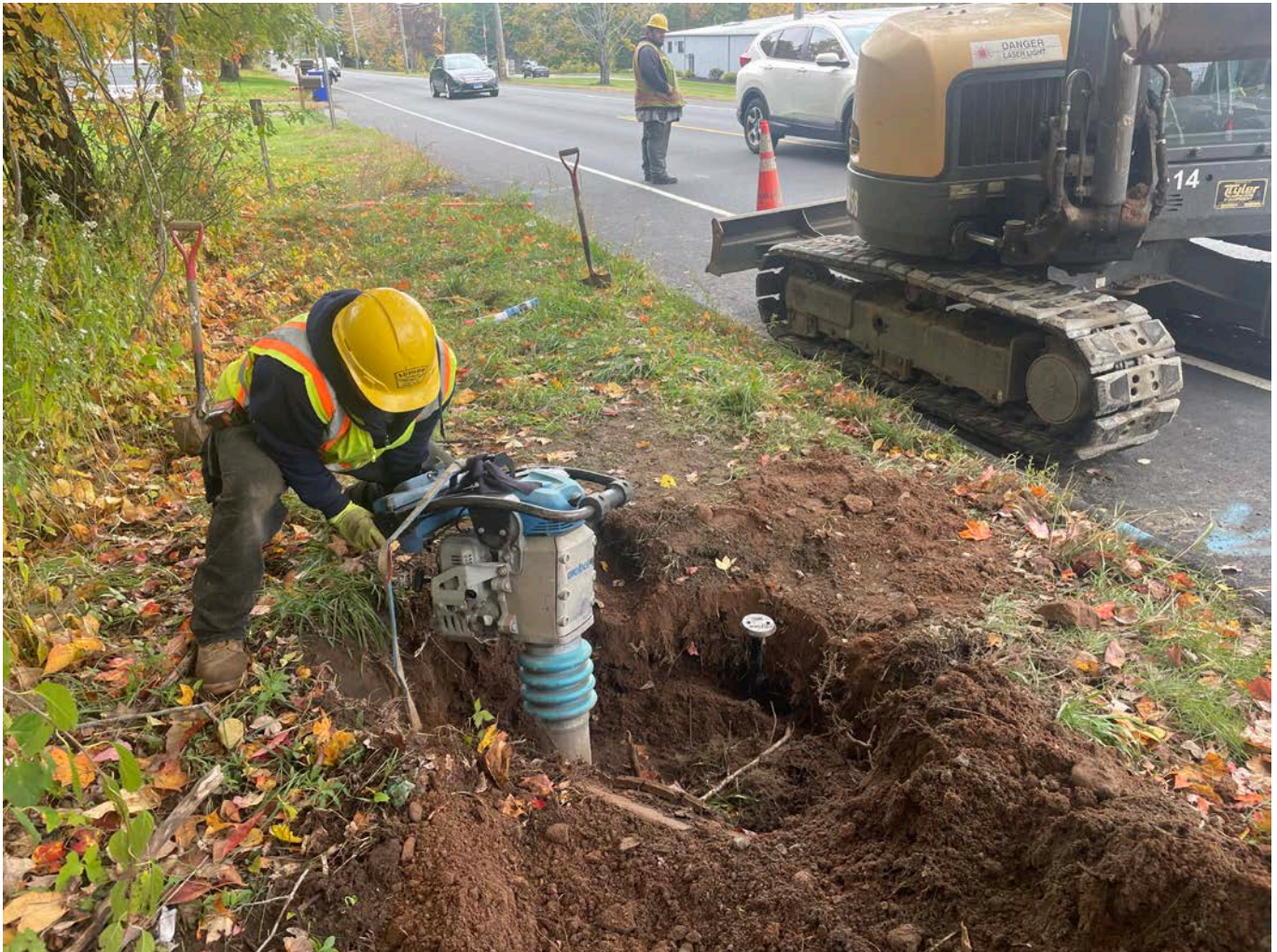
Picture 7: Ludlow compacting backfill that they placed around the new curb box they installed at the 2246-2266 S. Main Street, Middletown, property. View to the southwest.
