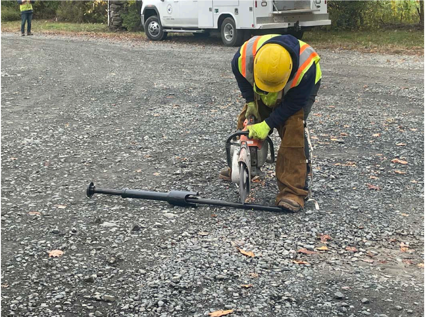
Picture 3: Ludlow cutting a piece from the upper section of a curb box that they are replacing at the 2175 S. Main Street, Middletown, property.
