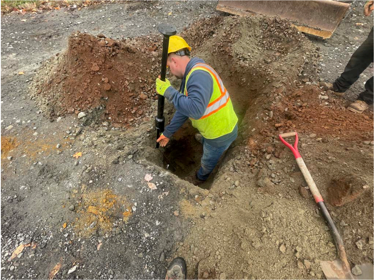
Picture 2: Ludlow replacing the curb box at the 2175 S. Main Street, Middletown. View to the southwest.
