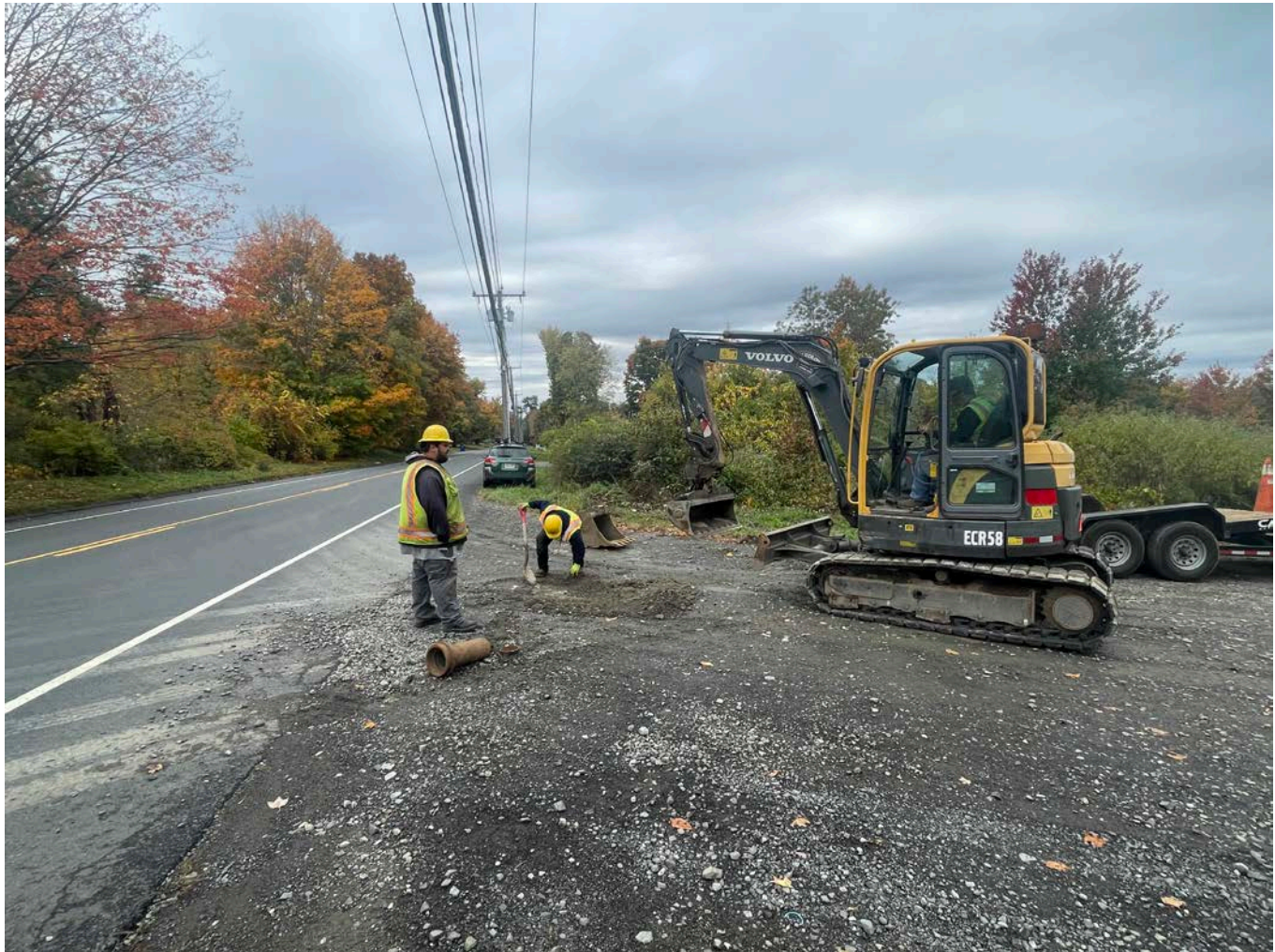
Picture 1: Ludlow daylighting a curb stop at the 2175 S. Main Street, Middletown, property to replace the curb box. View to the south.
