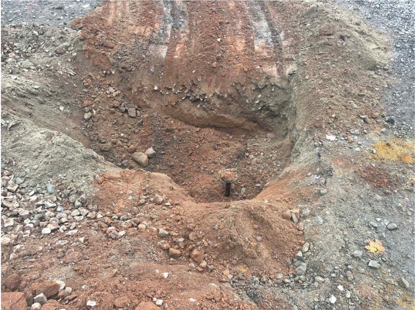
Picture 4: View of the curb box that Ludlow installed at the 2175 S. Main Street, Middletown property.
