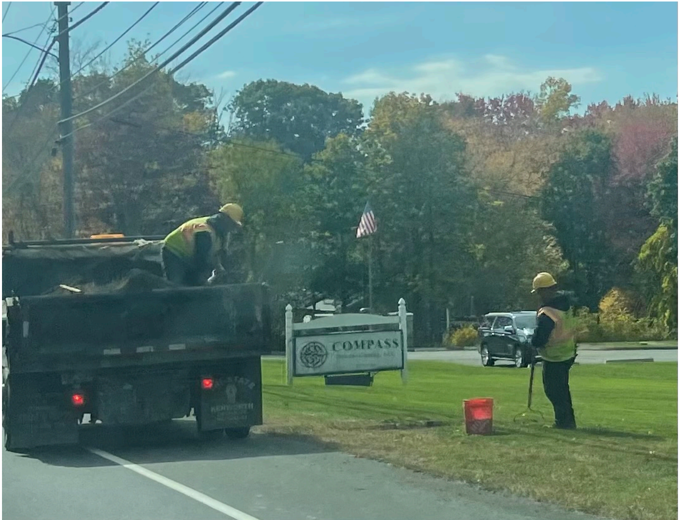
Picture 8: Ludlow placing loam and grass seed around the curb box located on the 2303 S. Main Street, Middletown, property. View to the southwest.
