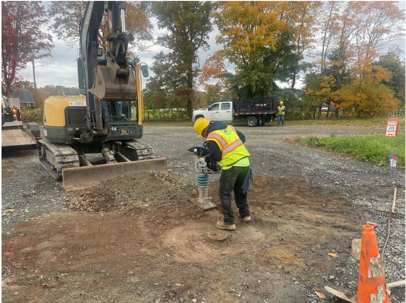
Picture 5: Ludlow compacting backfill placed around the new curb box that Ludlow installed at the 2175 S. Main Street, Middletown, property. View to the northwest.
