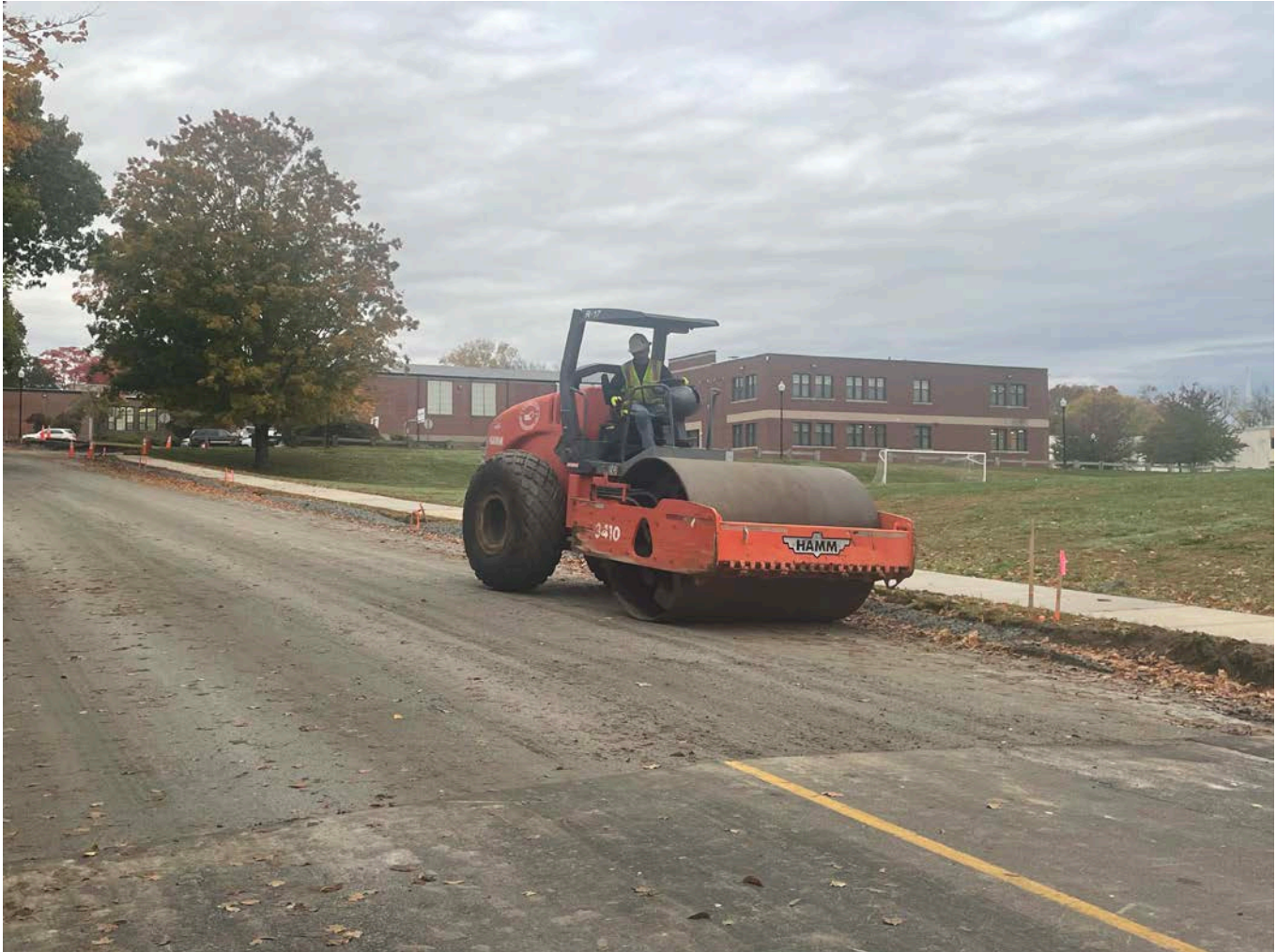
Picture 1: Ludlow using a Hamm 3410 soil compactor on the 1.25" processed gravel they placed between Stations 10+00 and 18+13 on Pickett Lane. View to the northwest.
