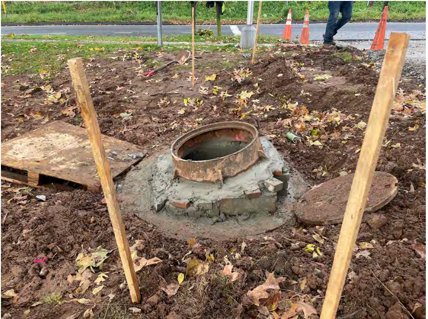
Picture 4: View of the manhole that Ludlow installed on the northwest corner of the 177R Main Street, Durham, property after Ludlow adjusted the height and the angle of the manhole. View to the west.
