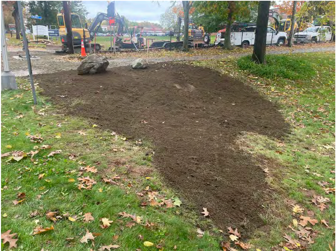
Picture 7: Loam and grass seed that Ludlow placed around the manhole they installed on the northwest corner of the 177R Main Street, Durham, property. View to the northeast.
