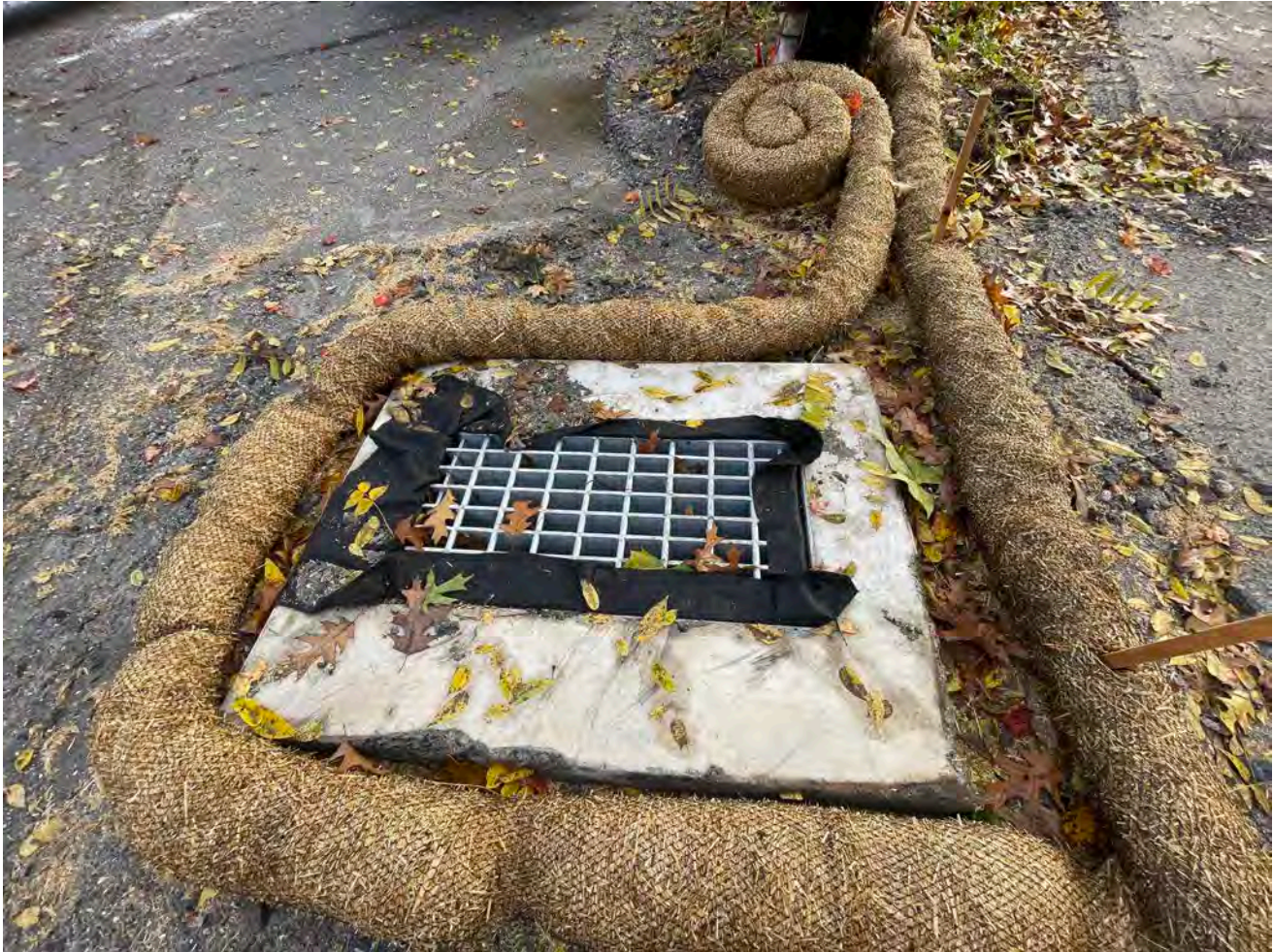
Picture 2: Hay wattle that Ludlow placed around the catch basin located at the southeast corner of the intersection of Pickett Lane and Main Street, Durham. View to the east.
