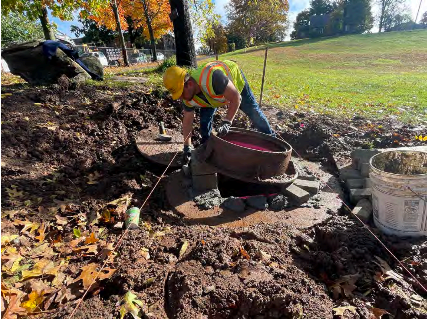
Picture 3: Ludlow adjusting the height and angle of the top of the manhole they installed on the northwest corner of the 177R Main Street, Durham, property. View to the east.
