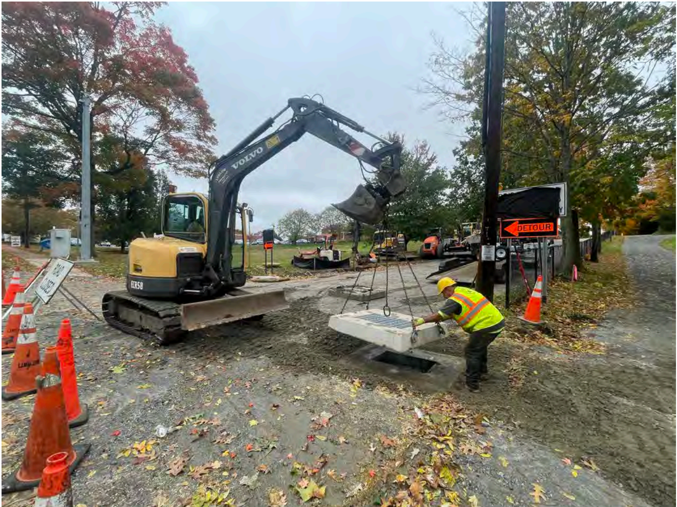
Picture 6: Ludlow changing out a damaged top on the catch basin they installed on the southeast corner of where Pickett Lane and Main Street intersect. View to the northeast.
