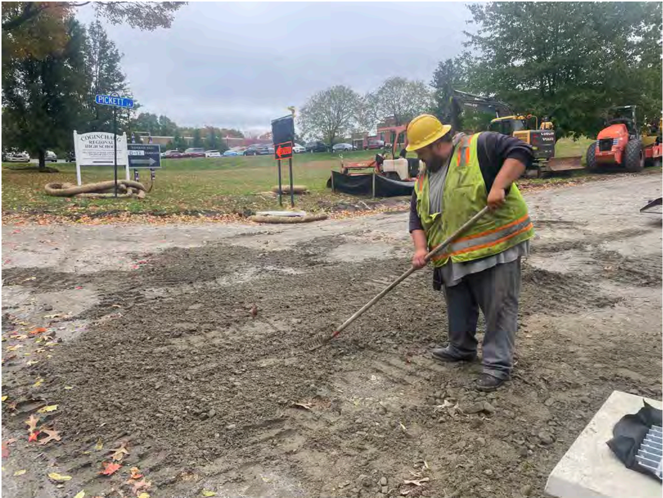
Picture 8: Ludlow raking out 1.25” processed gravel at Station 10_10 on Pickett Lane. View to the northeast.
