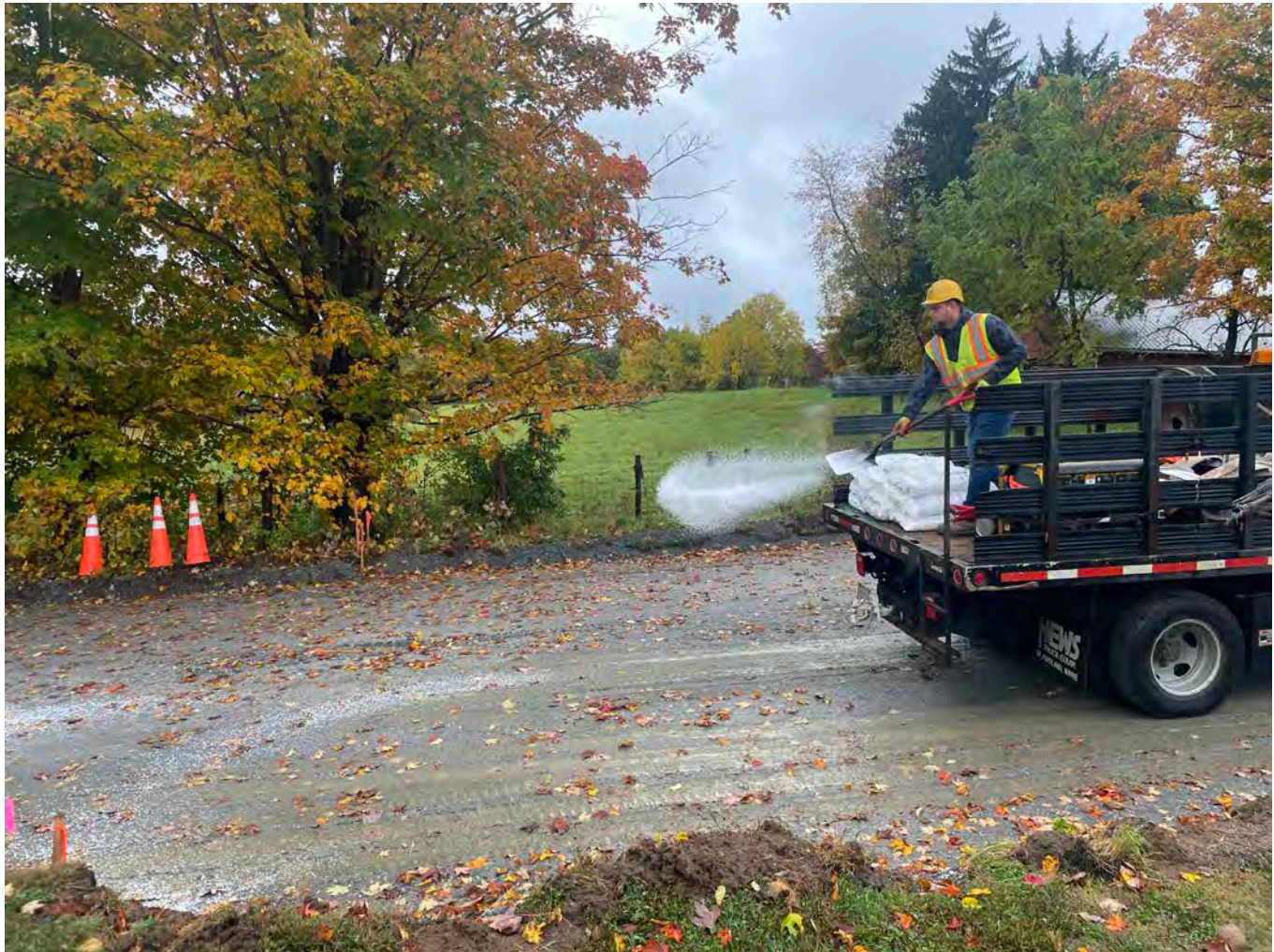
Picture 1: Ludlow spreading calcium chloride onto the 1.25" processed gravel they placed between Stations 10+00 and 18+13 on Pickett Lane. View to the south.
