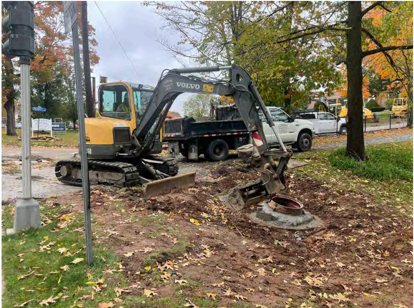
Picture 5: Ludlow placing 1.25" processed gravel around the manhole they installed on the northwest corner of the 177R Main Street, Durham, property. View to the northeast.
