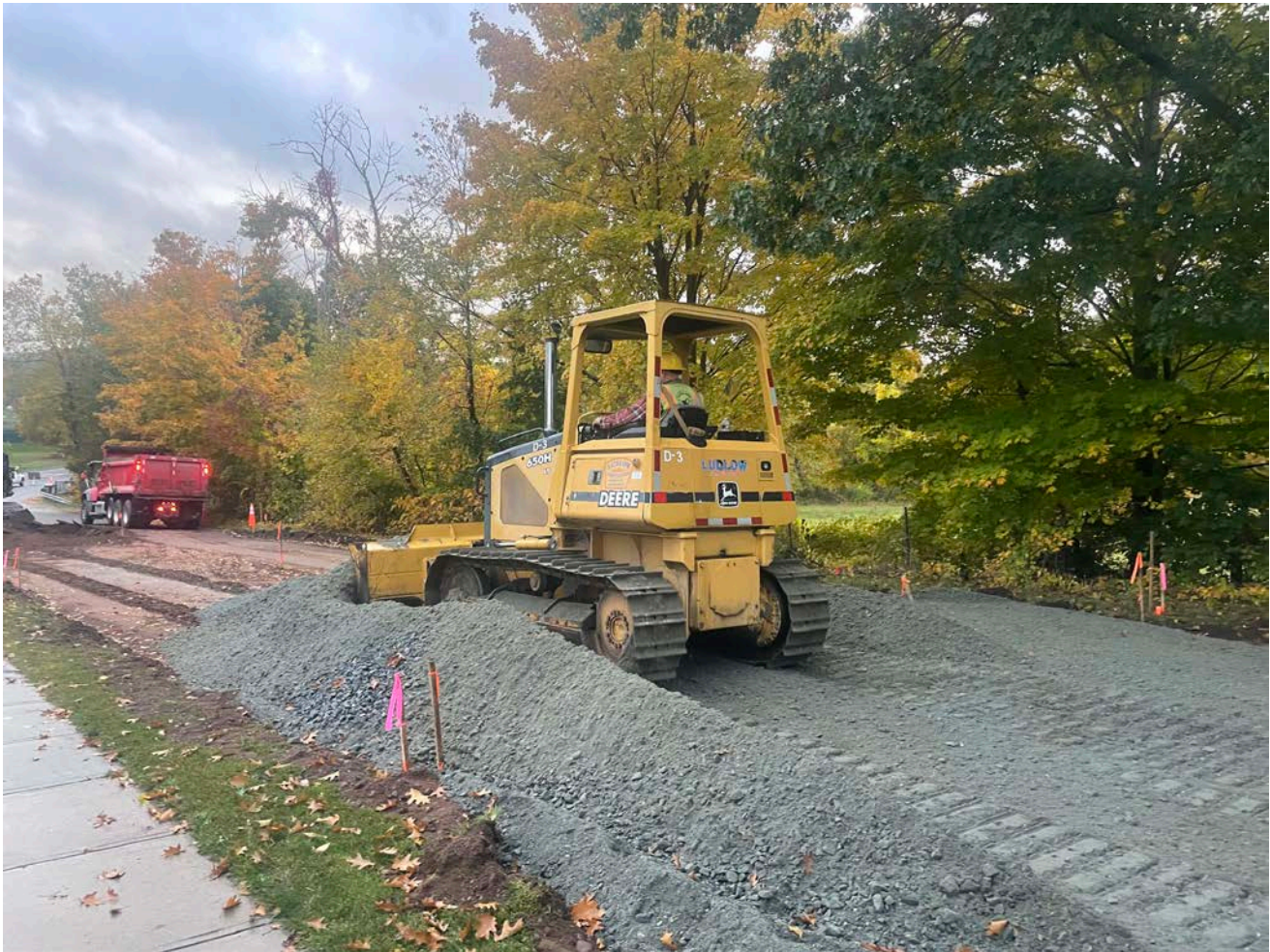
Picture 2: Ludlow grading 1.25" processed gravel at Station 17+15 on Pickett Lane with a Deere 650H dozer. View to the west.
