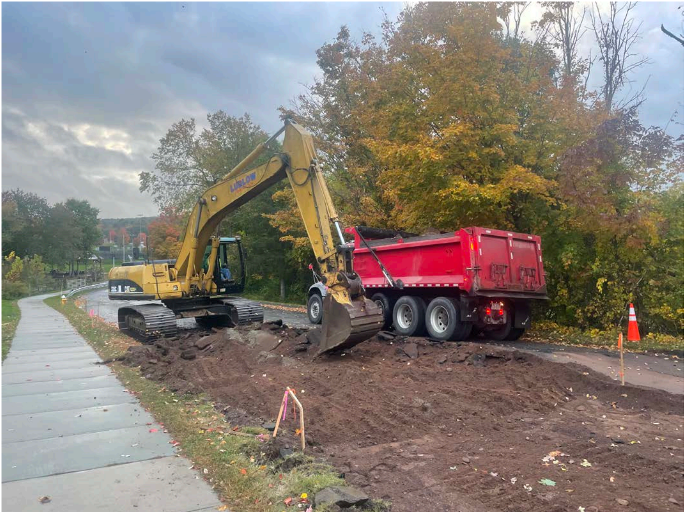
Picture 3: Ludlow removing existing asphalt and road base between Stations 18+00 and 18+13. View to the southeast.
