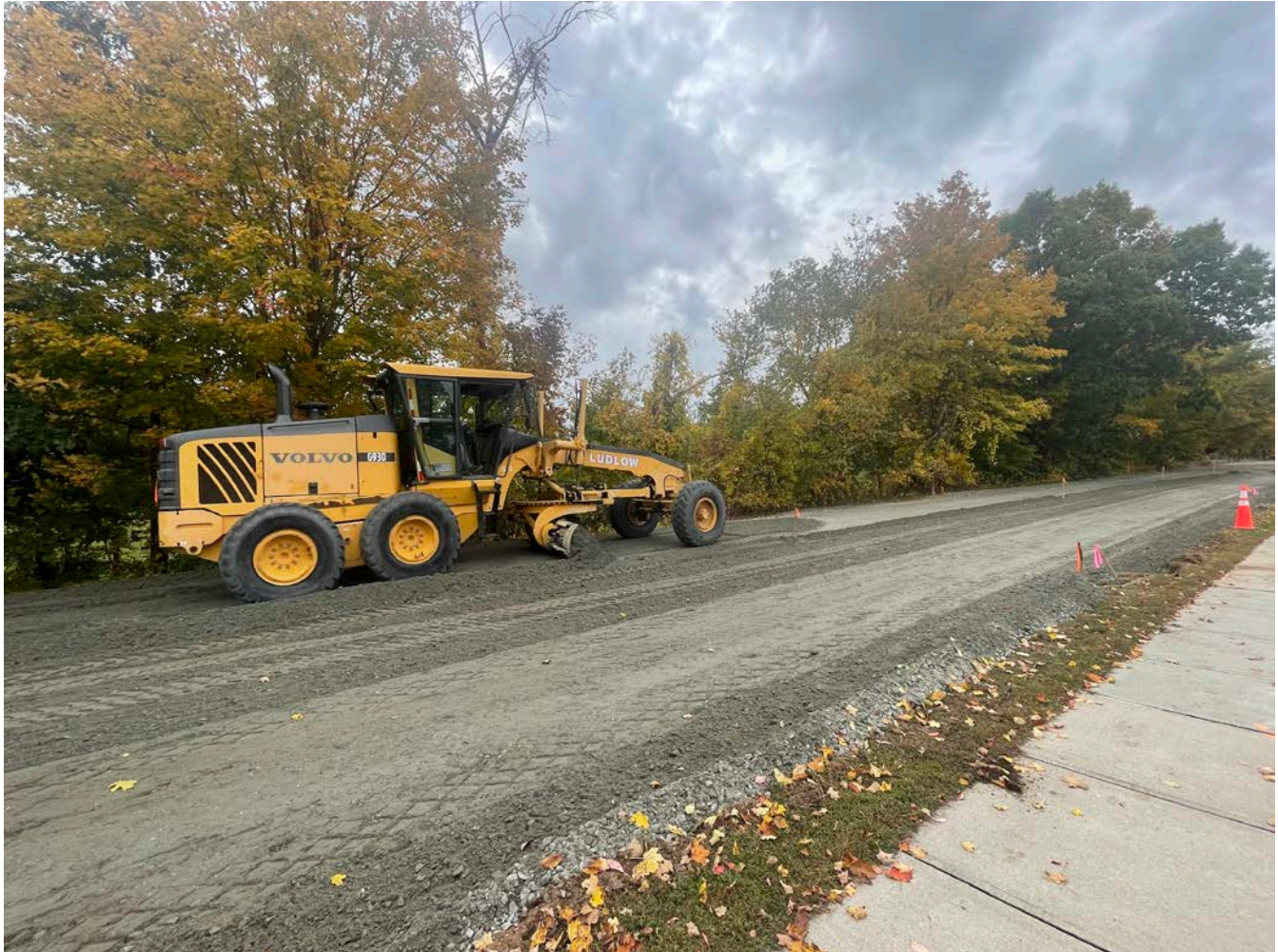
Picture 7: Ludlow grading 1.25" processed gravel on Pickett Lane with a Volvo G930 grader. View to the southwest.
