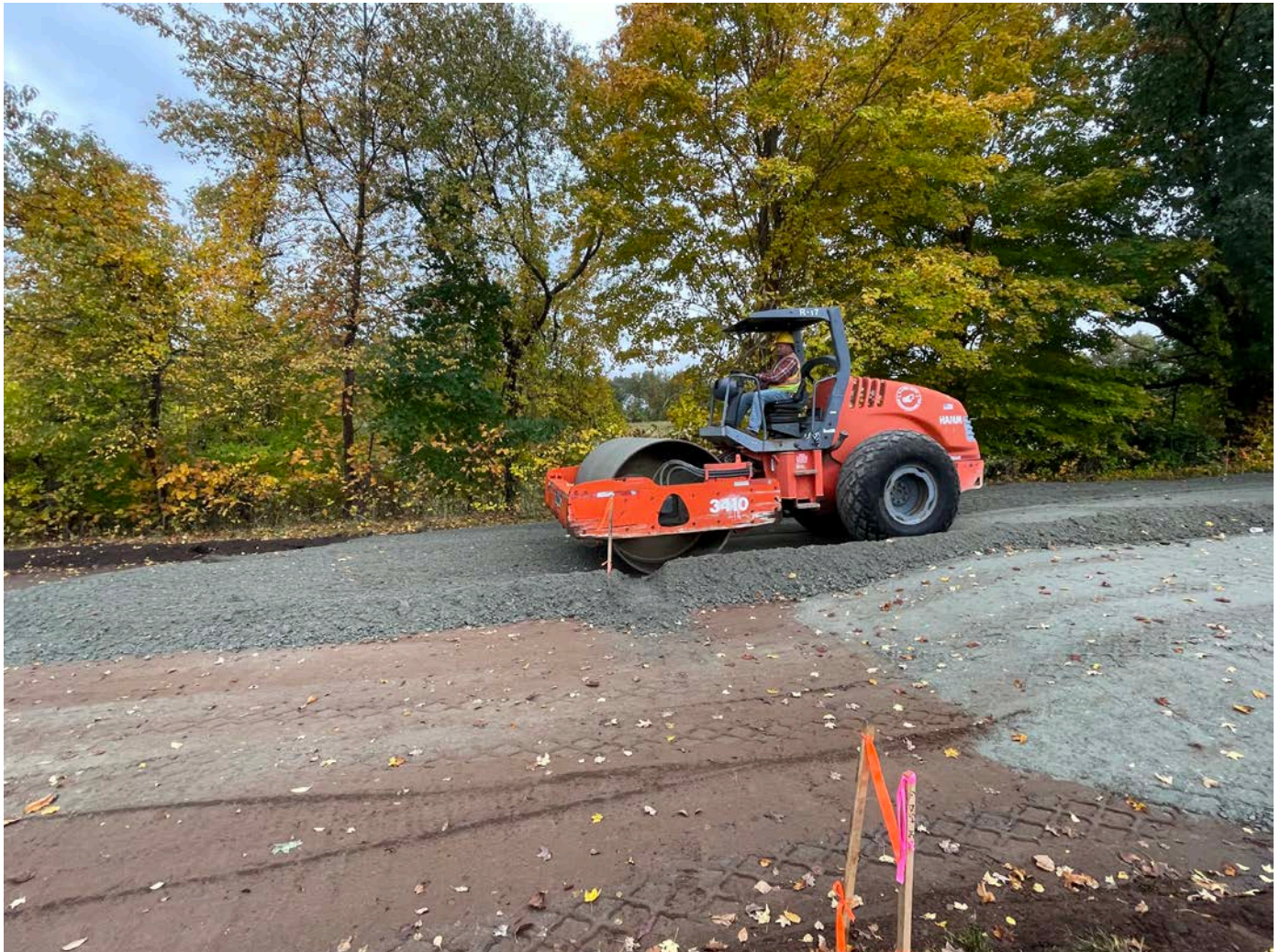
Picture 4: Ludlow using a Hamm 3410 soil compactor to compact the first of two lifts of 1.25" processed gravel between Station 17+00 and 17+15. View to the south.
