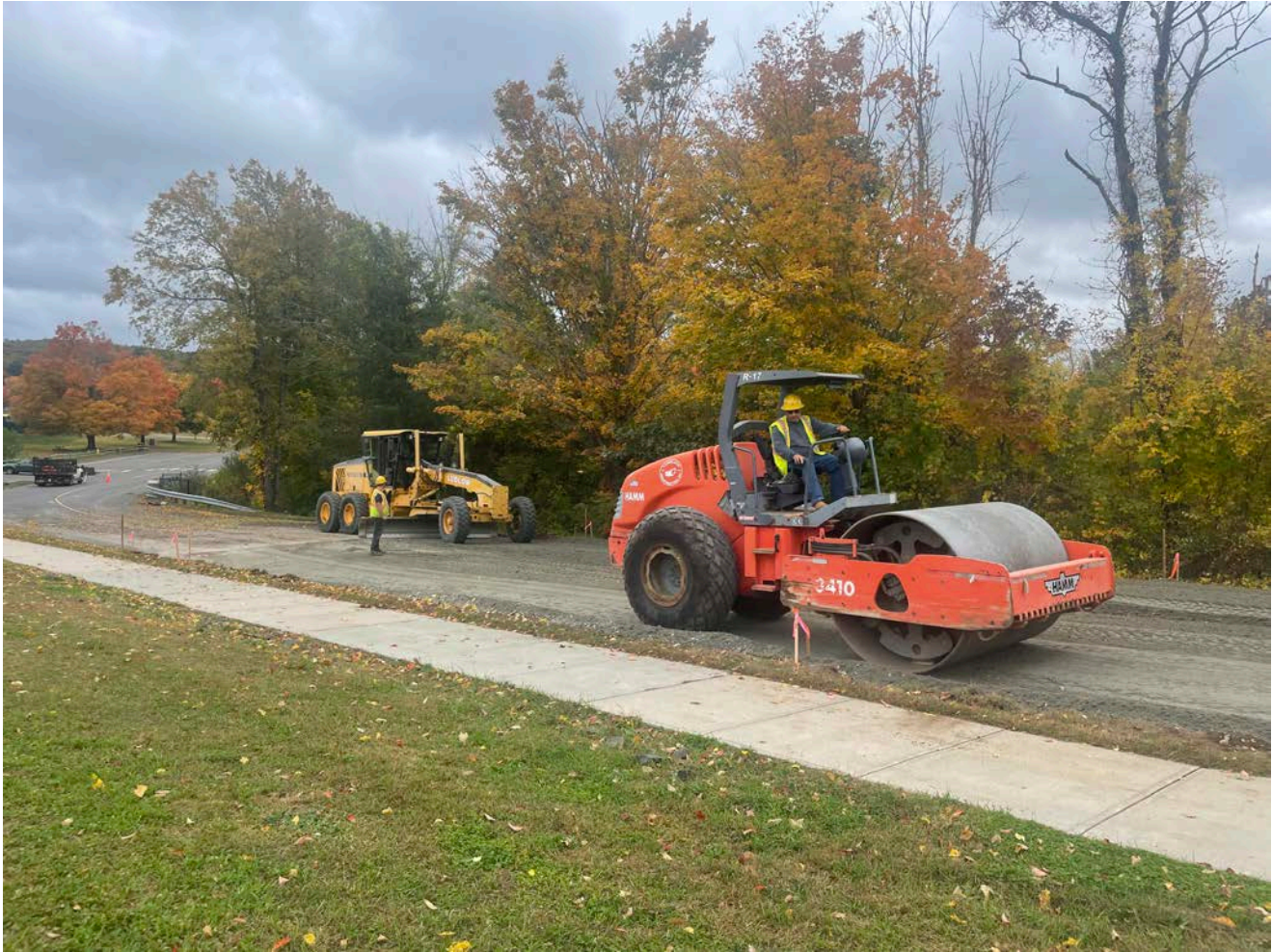
Picture 8: Ludlow grading and compacting 1.25" processed gravel between Stations 17+50 and 18+13 on Pickett Lane. View to the southeast.
