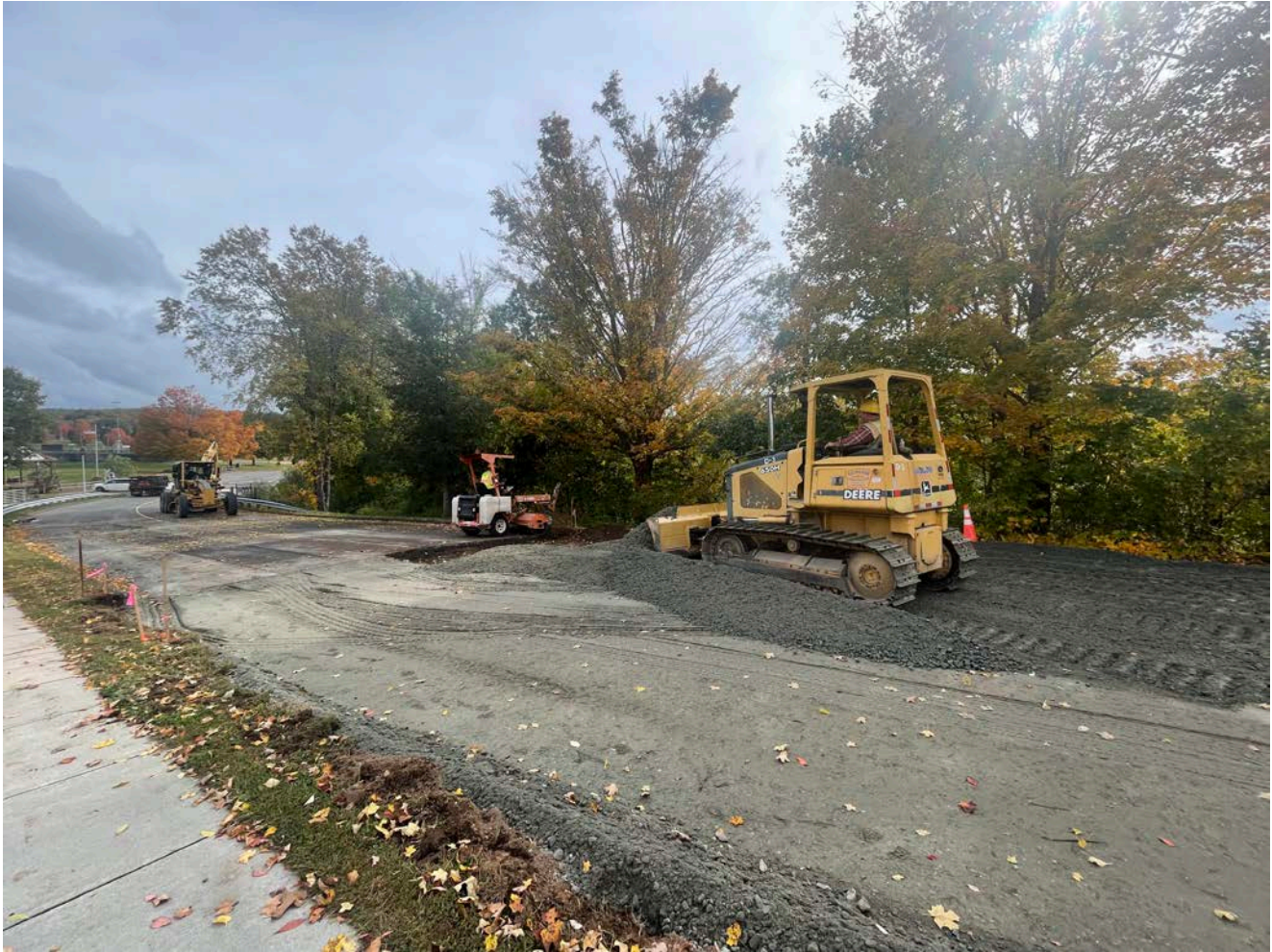
Picture 6: Ludlow grading 1.25” processed gravel at Station 18+00 on Pickett Lane with a Deere 650H dozer. View to the southeast.
