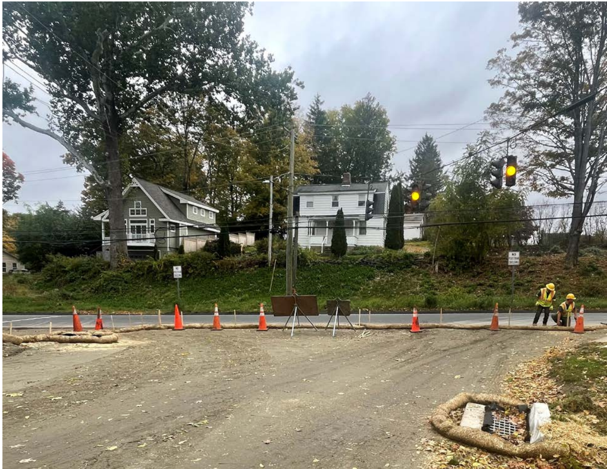
Picture 9: Straw wattles that Ludlow placed around two catch basins and across the intersection of Pickett Lane and Main Street. View to the west.
