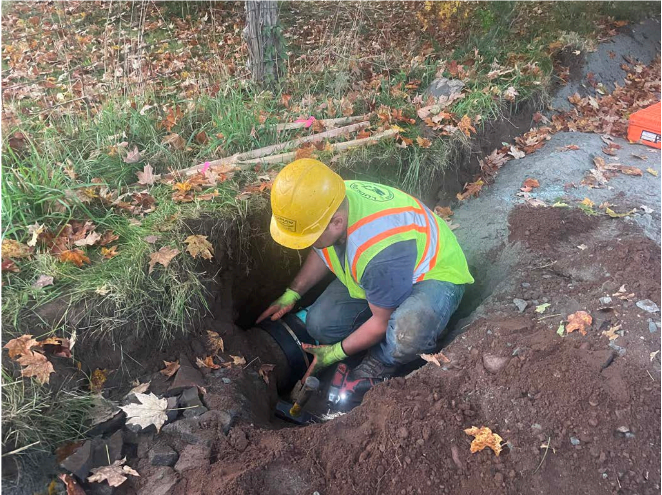
Picture 1: Ludlow fixing an 8" clay drain pipe located on the south side of Pickett Lane with Fernco boot and a section of 8" PVC at Station 14+50. View to the southwest.
