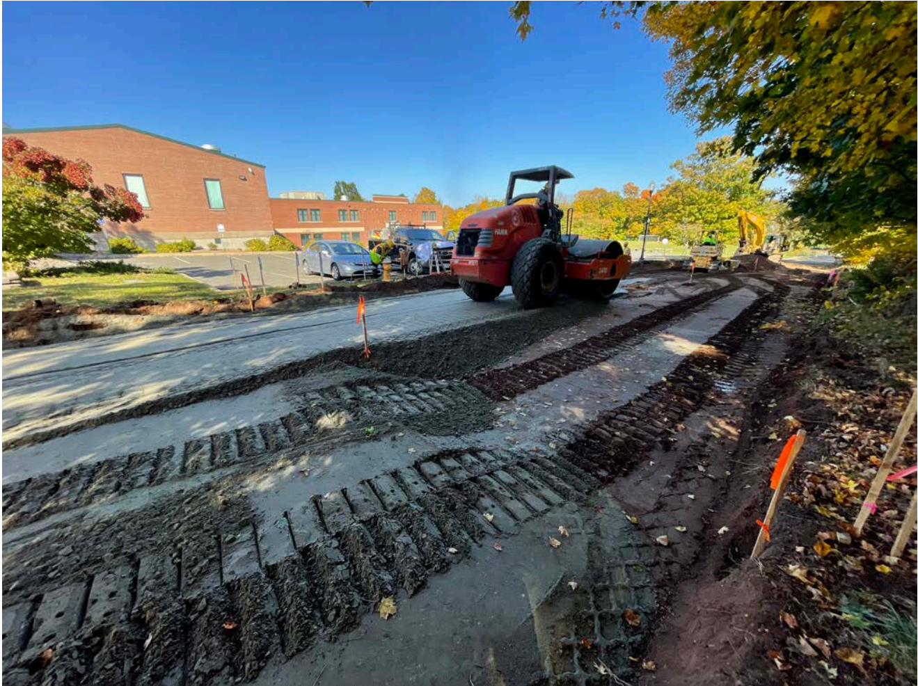
Picture 7: Ludlow using a Hamm 3410 soil compactor on 1.25" processed gravel at Station ~14+00. View to the northeast.
