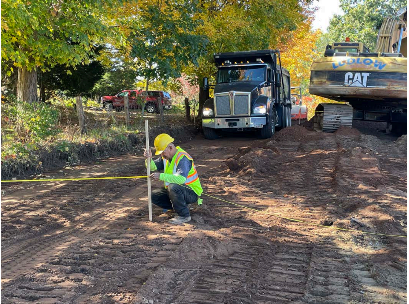
Picture 3: Ludlow placing a grade stake on the centerline of Pickett Lane at Station ~15+00. View to the west.
