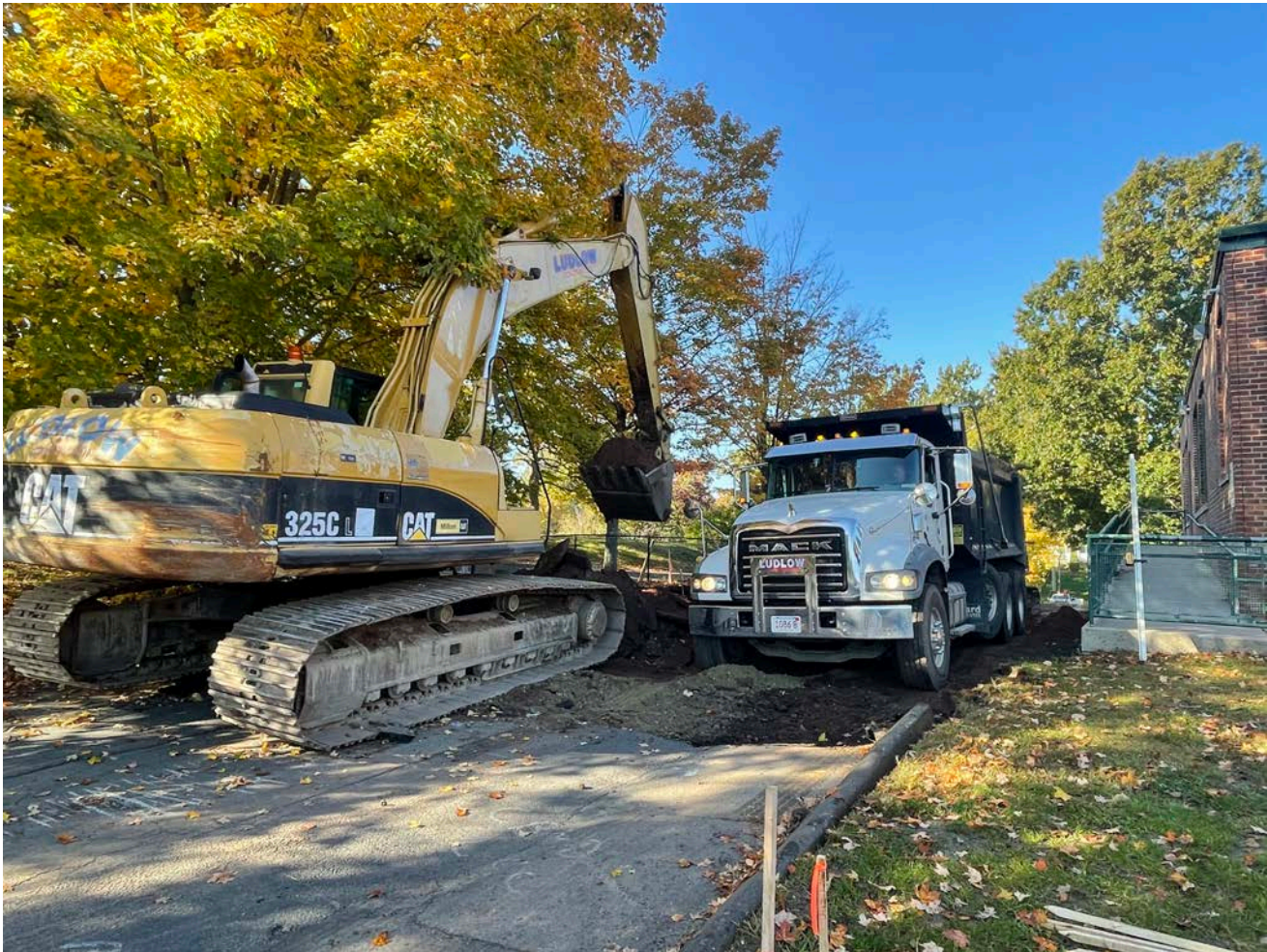
Picture 2: Ludlow excavating the existing road base on Pickett Lane at Station ~13+15. View to the west.
