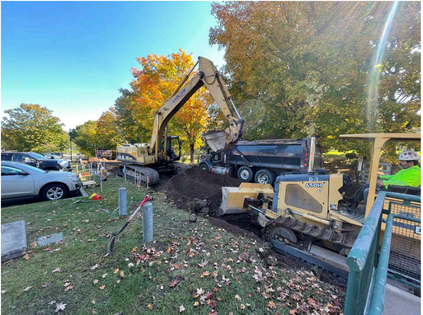
Picture 4: Ludlow excavating existing road base on the footprint of Pickett Lane at Station 13+50. View to the southeast.
