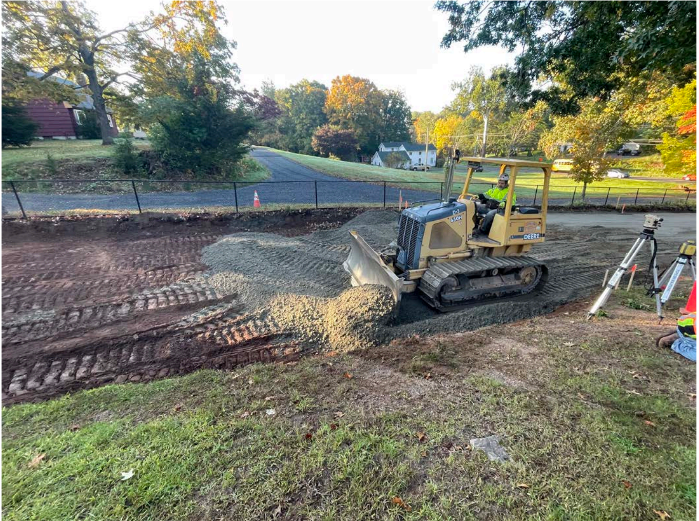
Picture 1: Ludlow grading 1.25" processed gravel on the footprint of Pickett Lane, Durham at Station ~11+70. View to the southwest.
