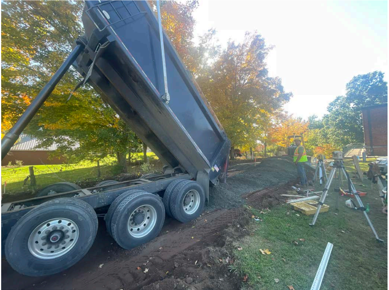
Picture 6: Ludlow placing 1.25" processed gravel on the footprint of Pickett Lane at Station ~14+50. View to the west.
