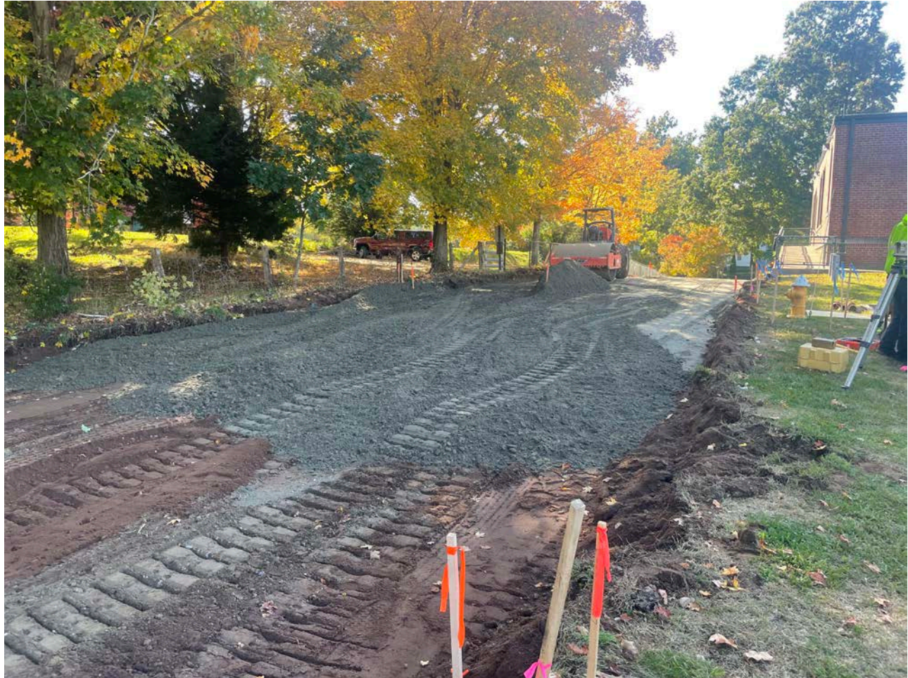
Picture 8: View from Station 14+00 looking west at the end of the day, where Ludlow has placed 1.25” processed gravel up to Station 13+90.
