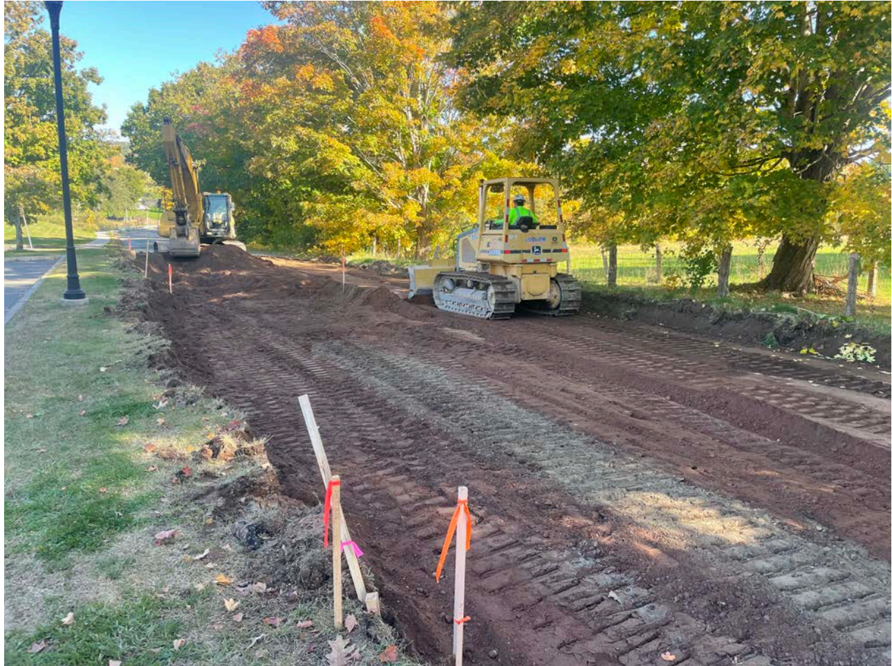
Picture 9: View from Station 14+00 looking east at the end of the day, where Ludlow has removed the majority of the existing road base.
