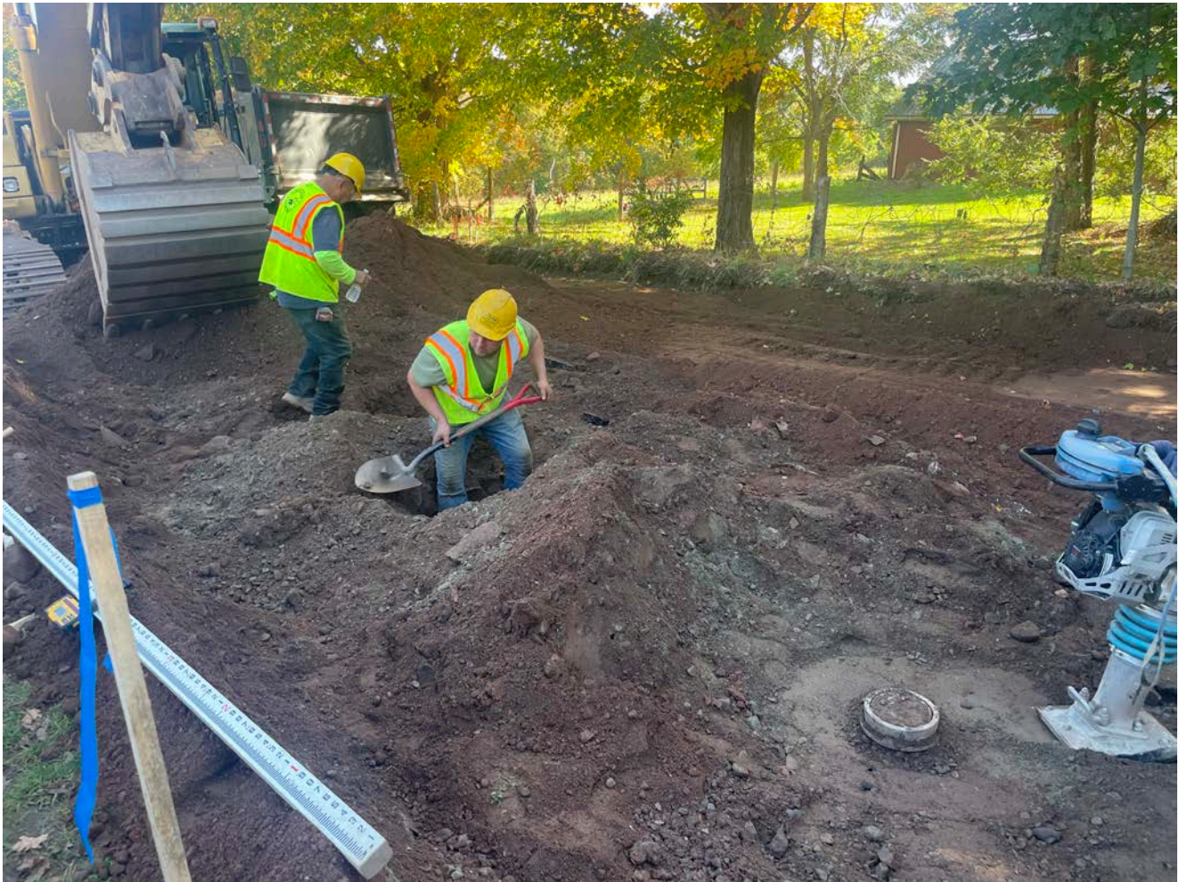
Picture 5: Ludlow adjusting the height of three road boxes located approximately between Stations 13+20 and 13+57 on Pickett Lane, Durham. View to the southeast.
