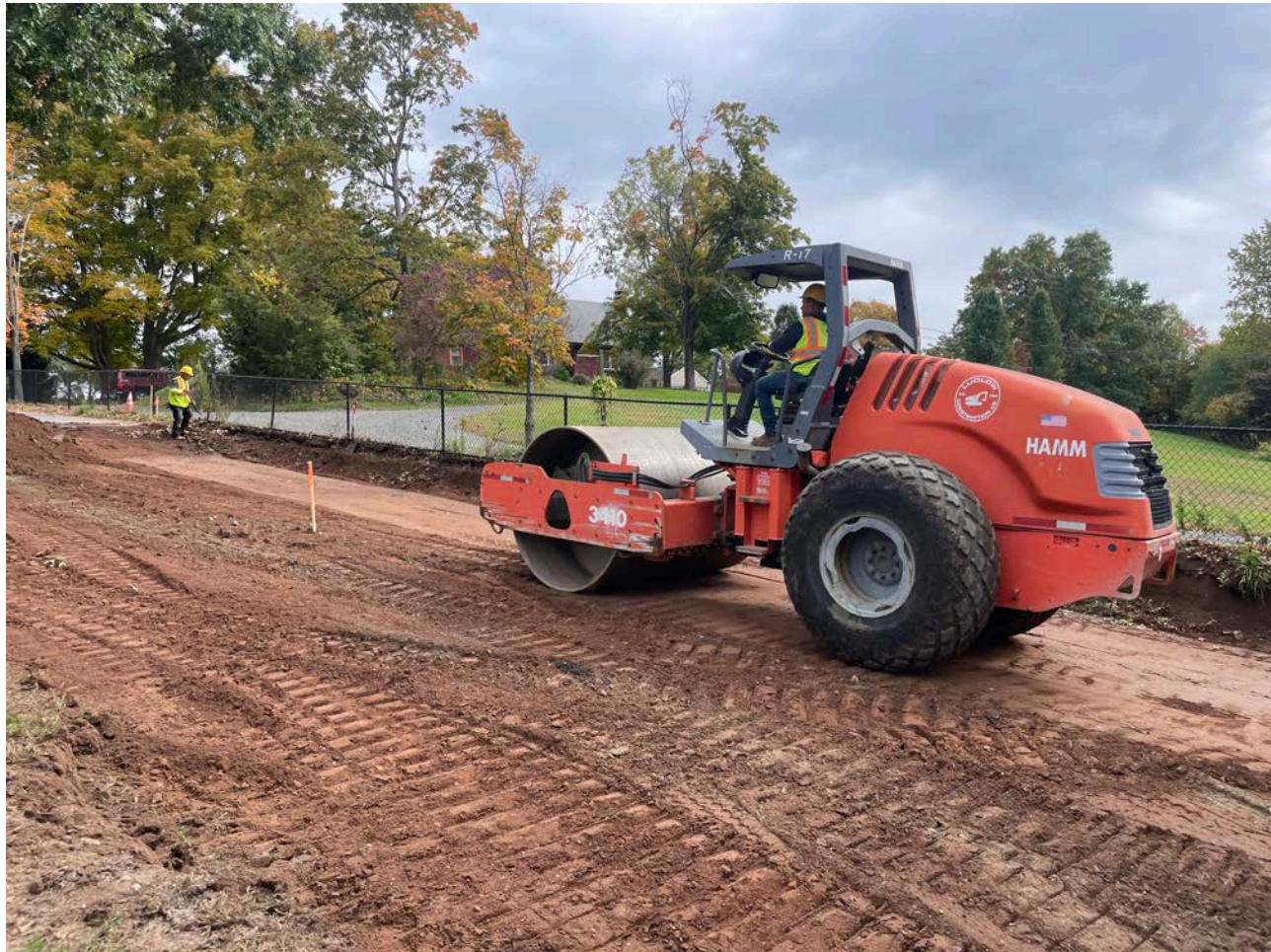
Picture 8: Ludlow compacting soils within the footprint of Pickett Lane prior to the placement of 1.25" processed gravel. View to the southeast.
