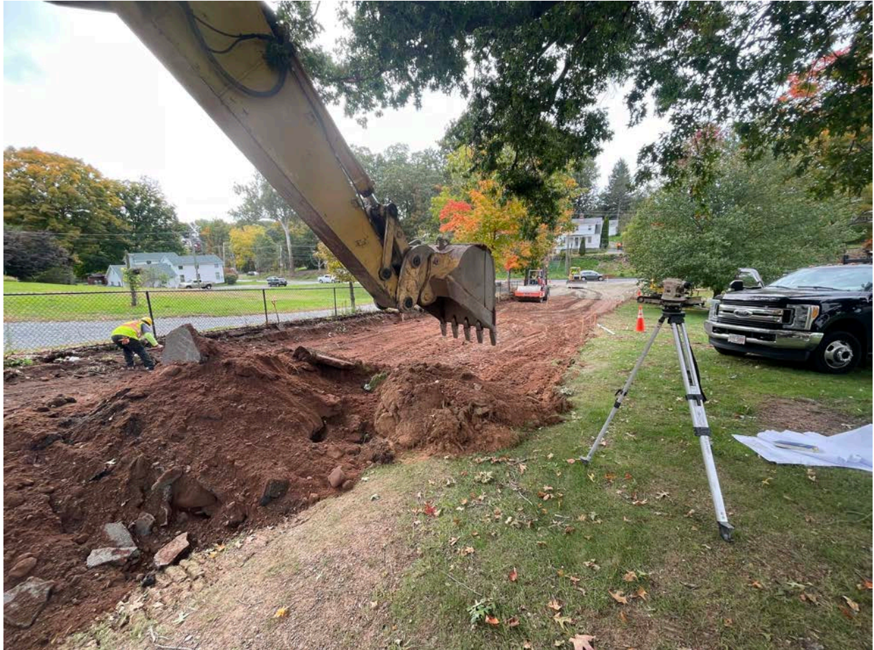
Picture 7: Ludlow removing old pavement and road base at Station 11+75 on Pickett Lane. View to the west.
