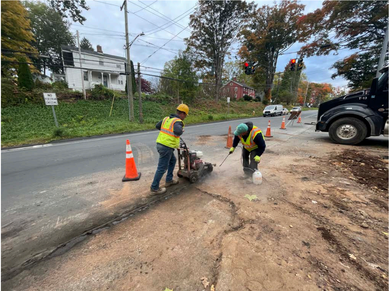
Picture 2: Ludlow saw-cutting pavement where the driveway for the 177R Main Street, Durham, property intersects with Main Street. View to the northwest.
