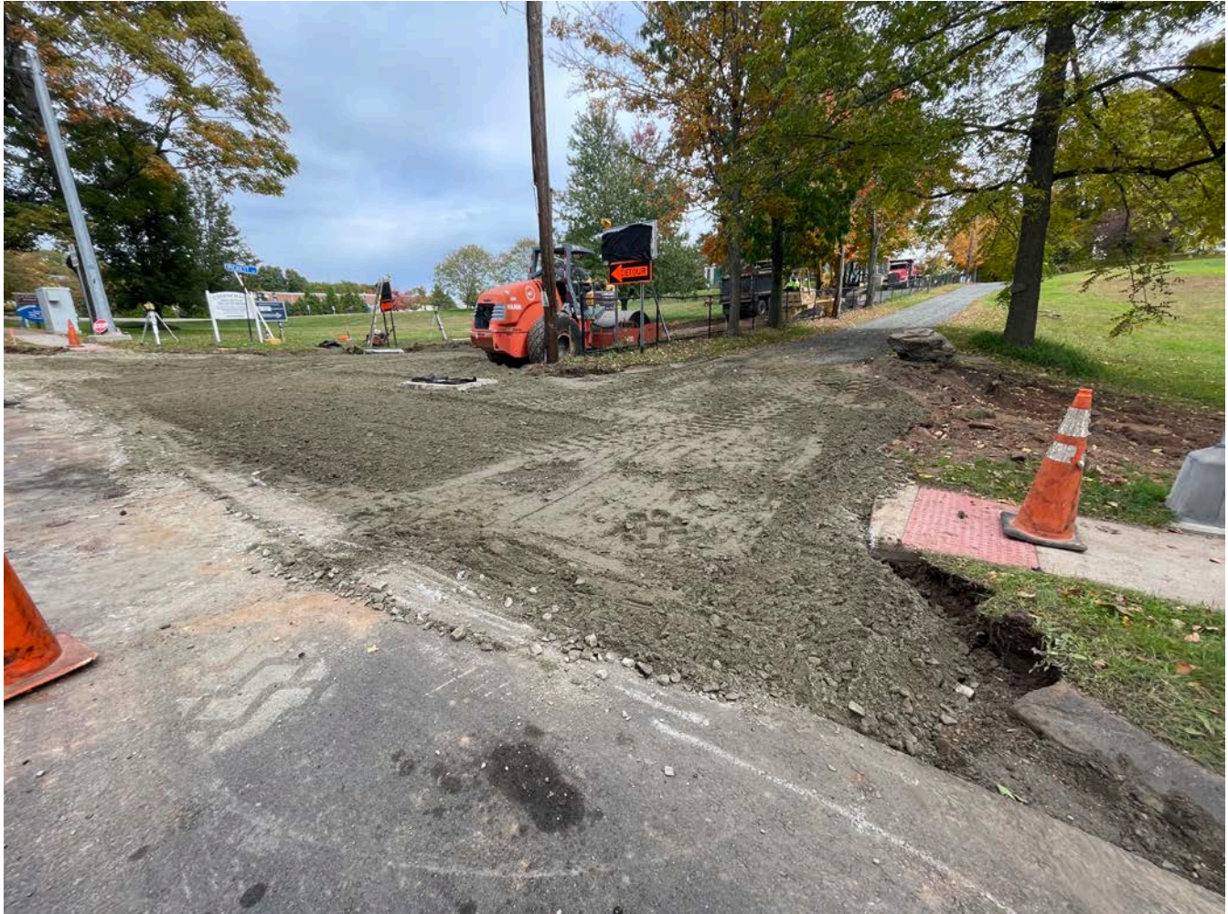
Picture 6: View to the northeast where Ludlow has placed 1.25" processed gravel where Picket Lane and the driveway for the 177R Main Street address where they intersect with Main Street.
