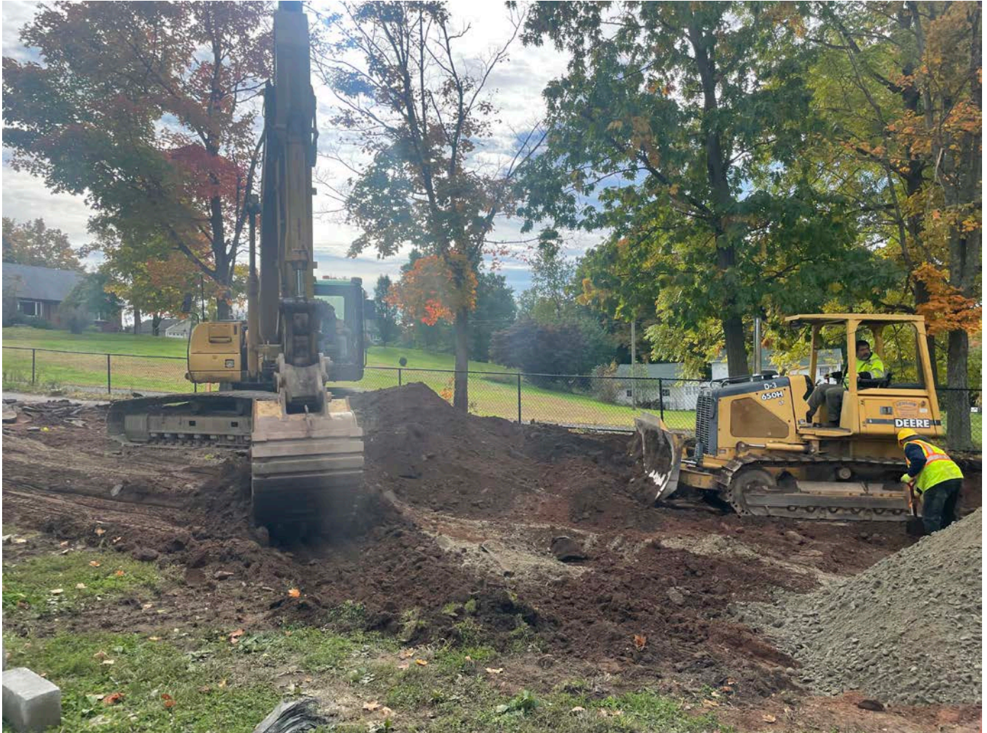
Picture 4: Ludlow excavating the old road base at Station 11+00 on Pickett Lane. View to the south.
