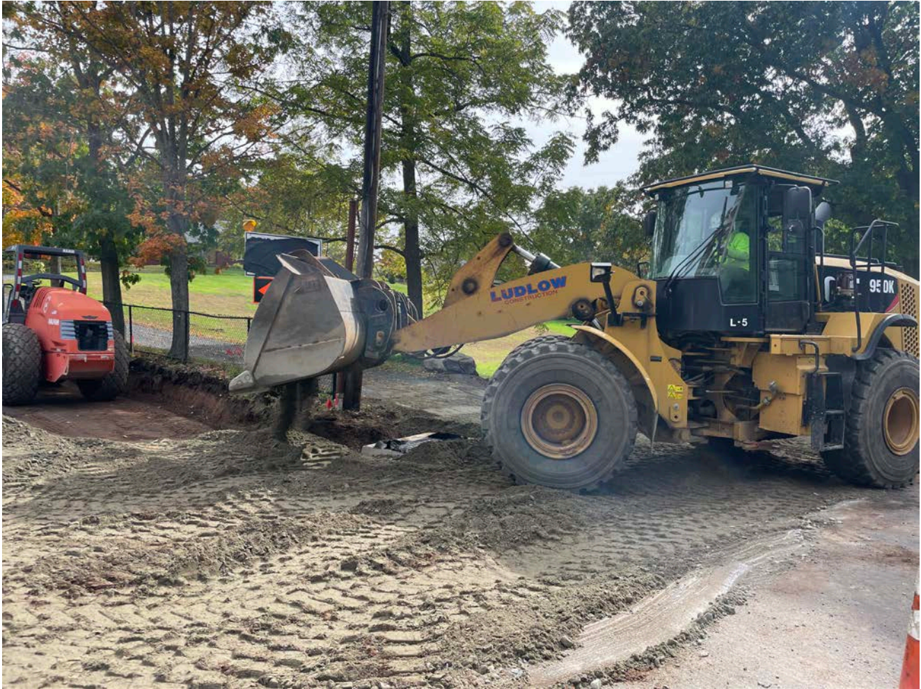
Picture 5: Ludlow placing 1.25" processed gravel at Station 10+25 on Pickett Lane. View to the southeast.
