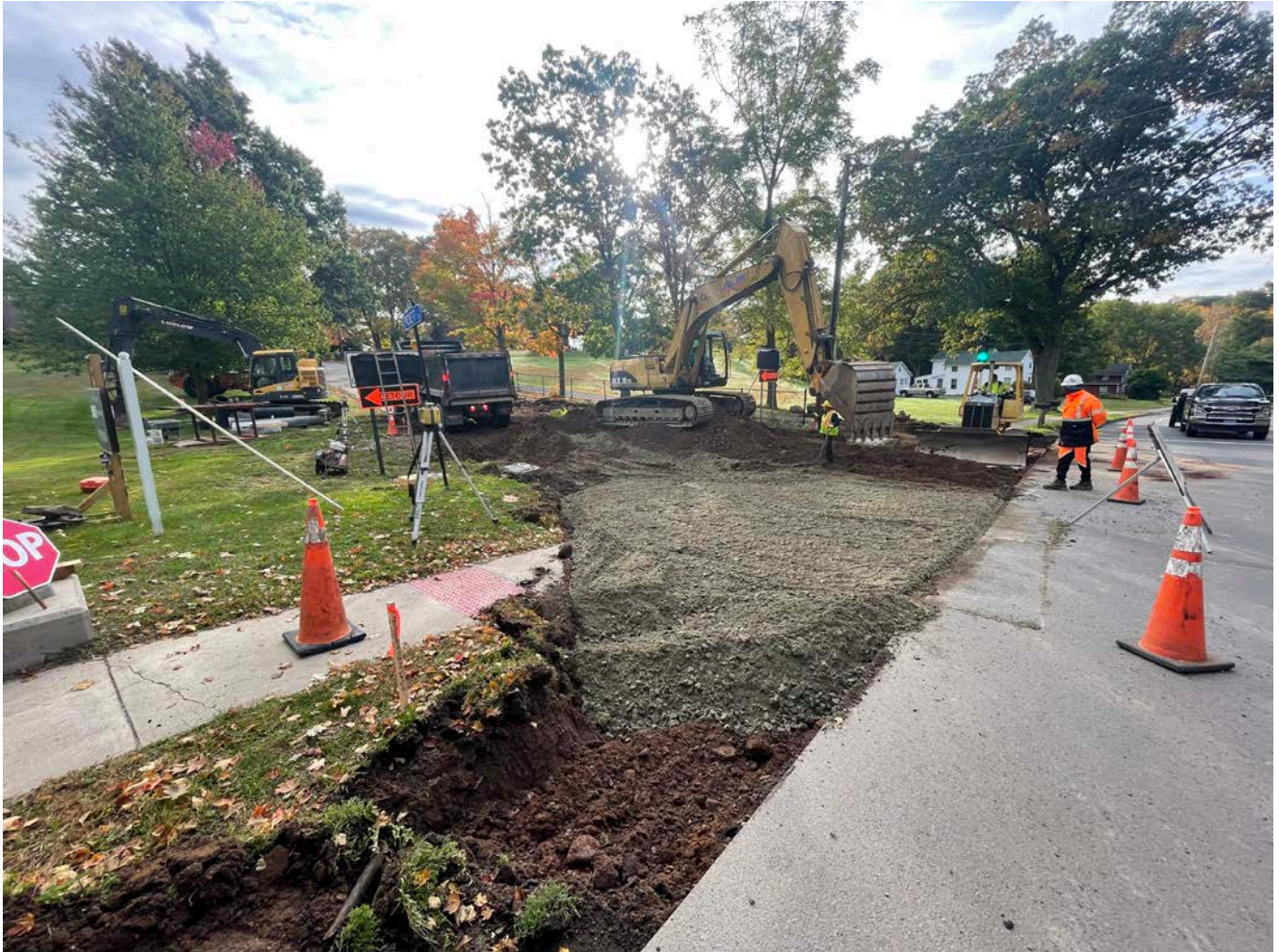
Picture 3: View to the southeast looking from Station 10+00 on Pickett Lane where Ludlow has placed a load of 1.25" processed gravel and continues earthwork in the background.
