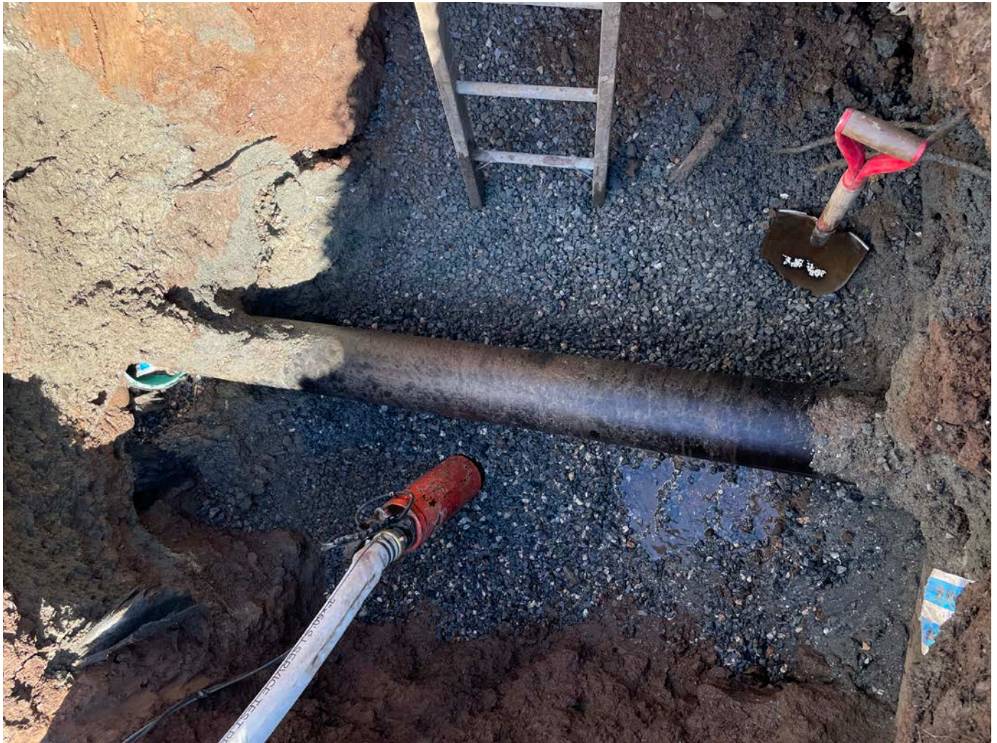
Picture 4: 8" DIP line that Ludlow daylighted on the east side of the Booster Station as they prepare to install an 8" gate valve. View to the north.
