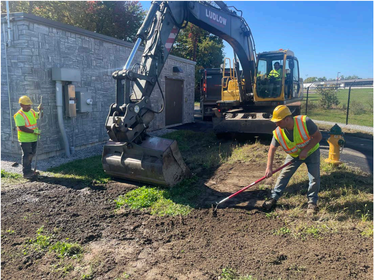
Picture 11: Ludlow placing loam and grass seed on those areas that were disturbed during the installation of an 8” gate valve on the east side of the Booster Station. View to the west.
