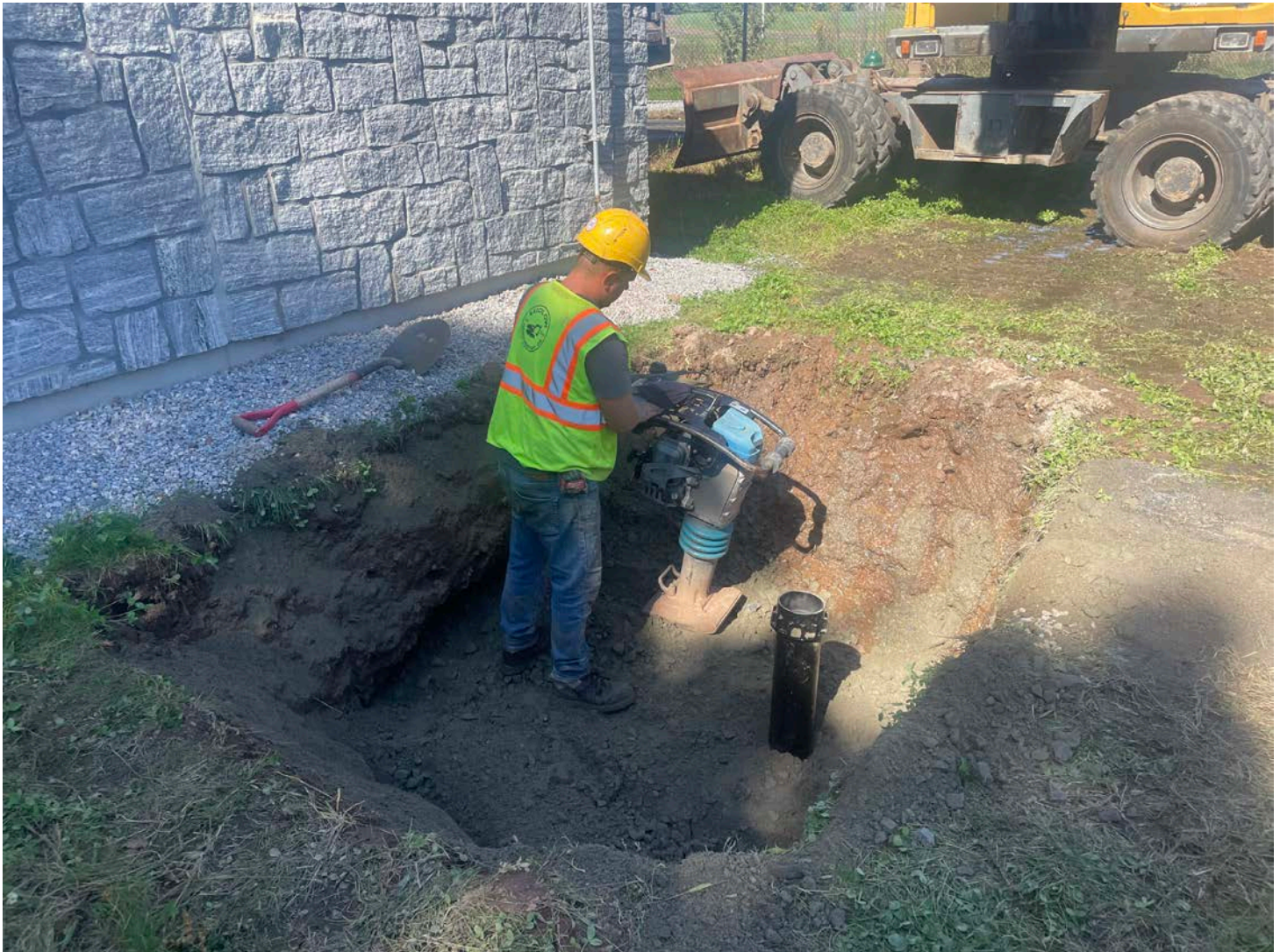
Picture 9: Ludlow compacting the 1.25" processed gravel they placed east side of the Booster Station. View to the northwest.
