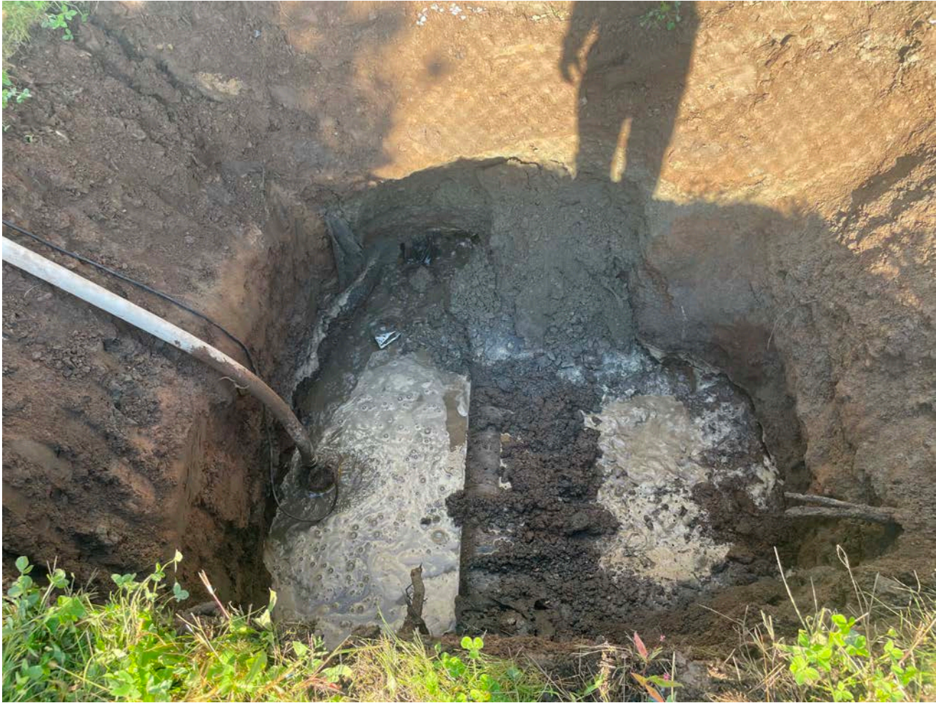
Picture 2: A pump that Ludlow set into the excavation they made while daylighting the 8" discharge line located on the east side of the Booster Station. View to the west.
