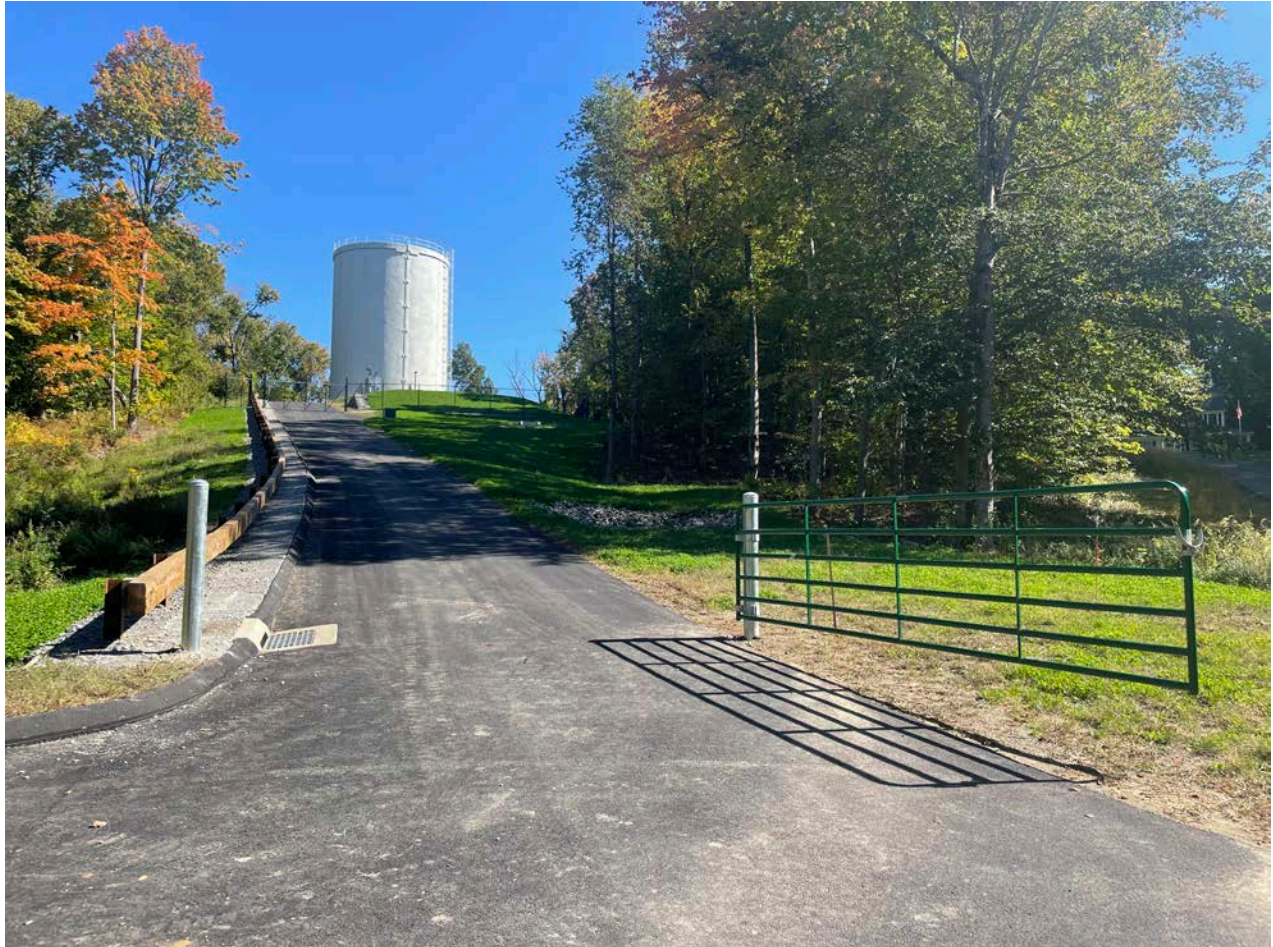
Picture 7: Fence that Eagle Fence finished installing near Station 14+00 on the Shared Access Road in Middletown. View to the east.
