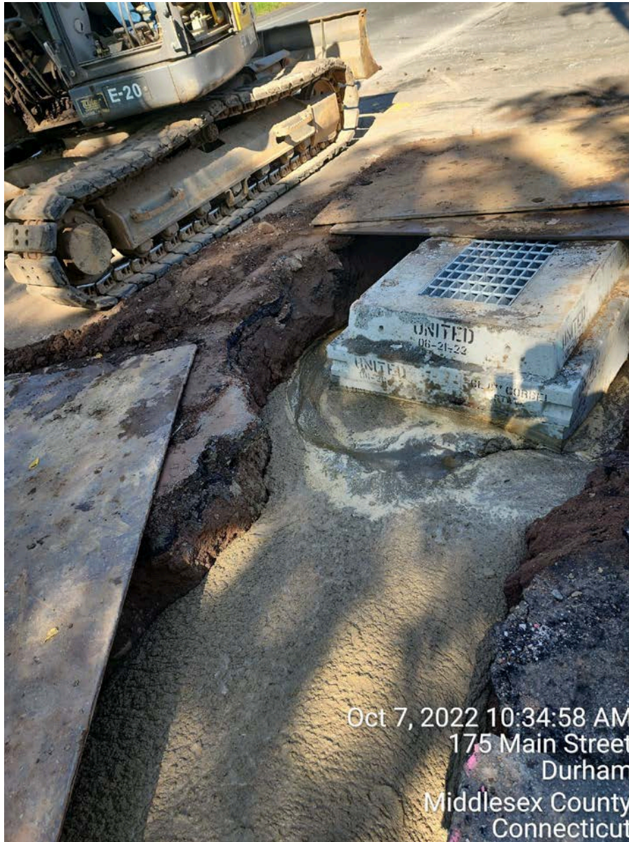
Picture 10: Flowable fill that Ludlow placed around the catch basin they installed on Pickett Lane and in the trench connecting the catch basin to the manhole they installed on 177R Main Street property. View to the north.
