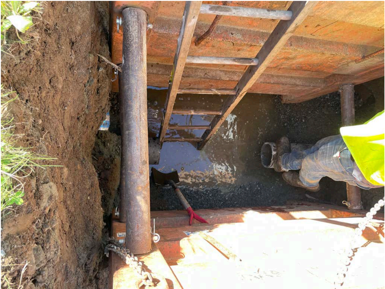
Picture 5: 8" DIP line that Ludlow daylighted on the east side of the Booster Station after having cut out a section of the pipe in order to install an 8" gate valve. View to the south.
