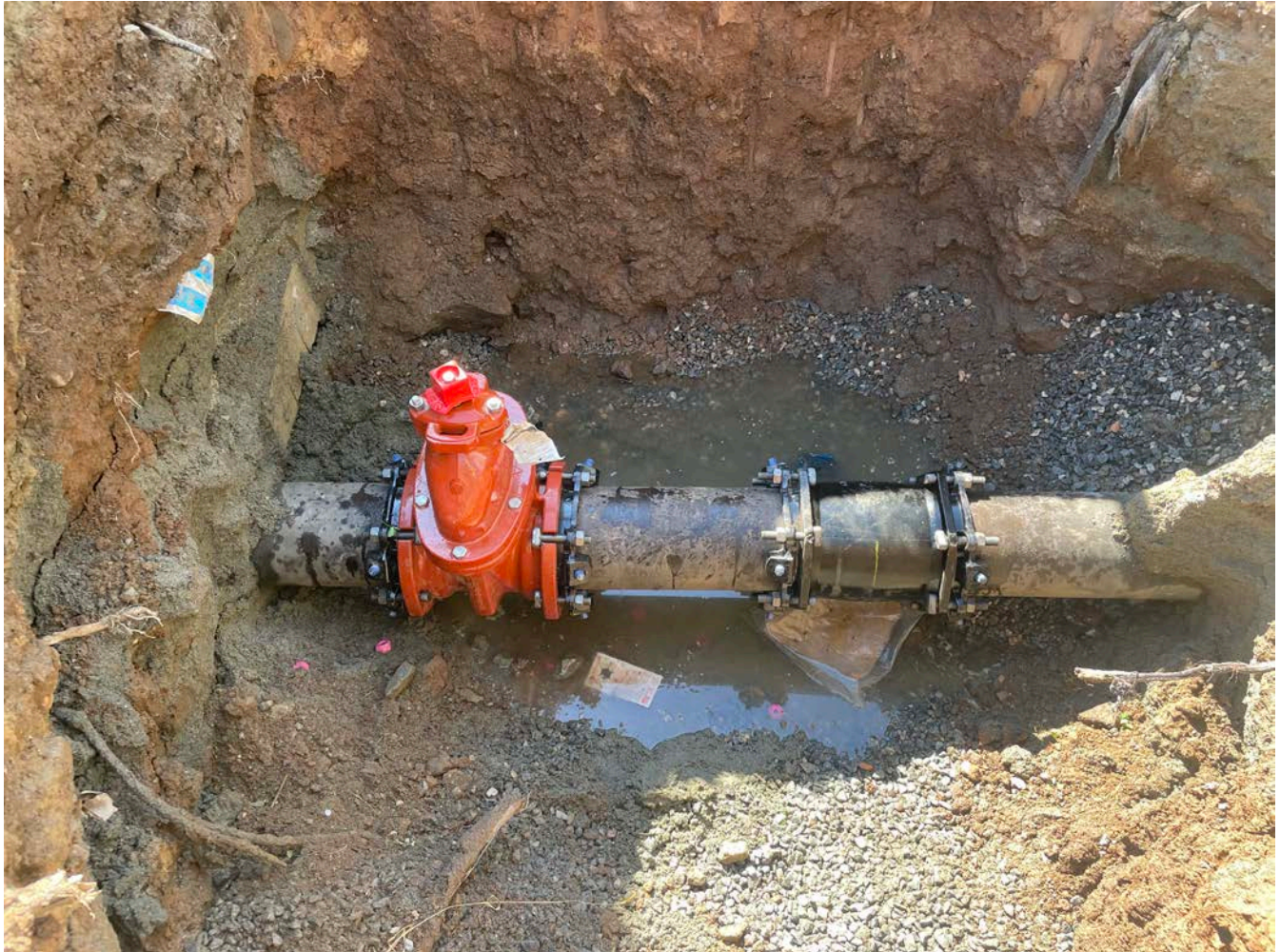
Picture 6: 8" gate valve that Ludlow installed on the 8" discharge line located on the east side of the Booster Station. View to the south.
