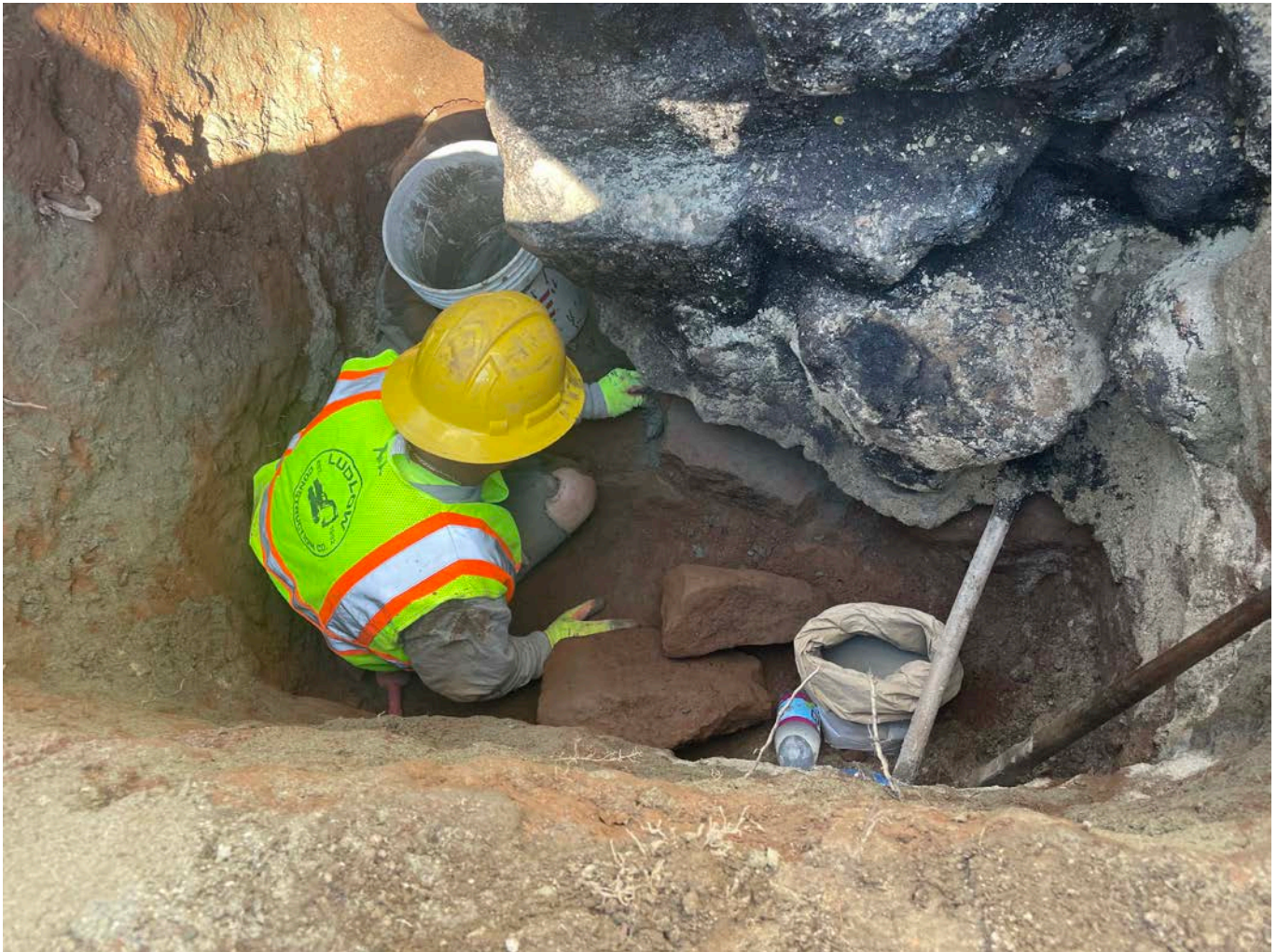
Picture 3: Ludlow placing portland cement on the southwest exterior of the foundation of the 24 Maiden Lane, Durham, residence. View to the north.
