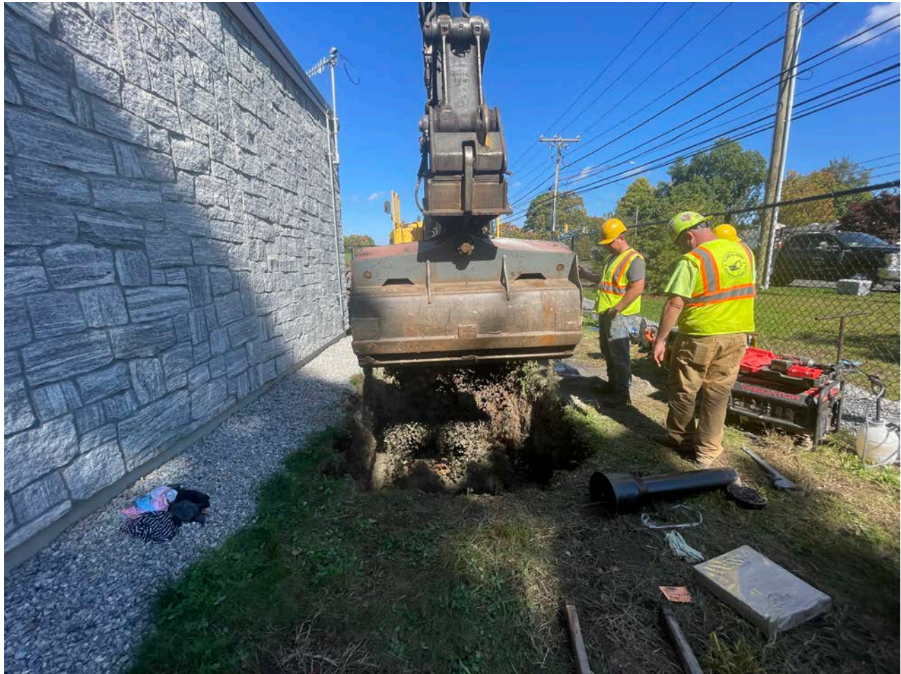
Picture 8: Ludlow placing 1.25" processed gravel over the sand they placed on the 8" gate valve they installed on the east side of the Booster Station. View to the north.
