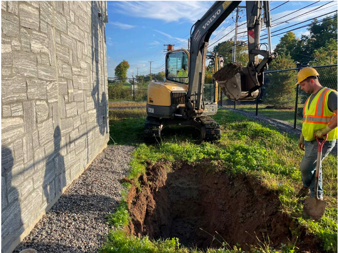
Picture 1: Ludlow excavating on the east side of the Booster station to install a gate valve on the 8" DIP discharge line. View to the north.
