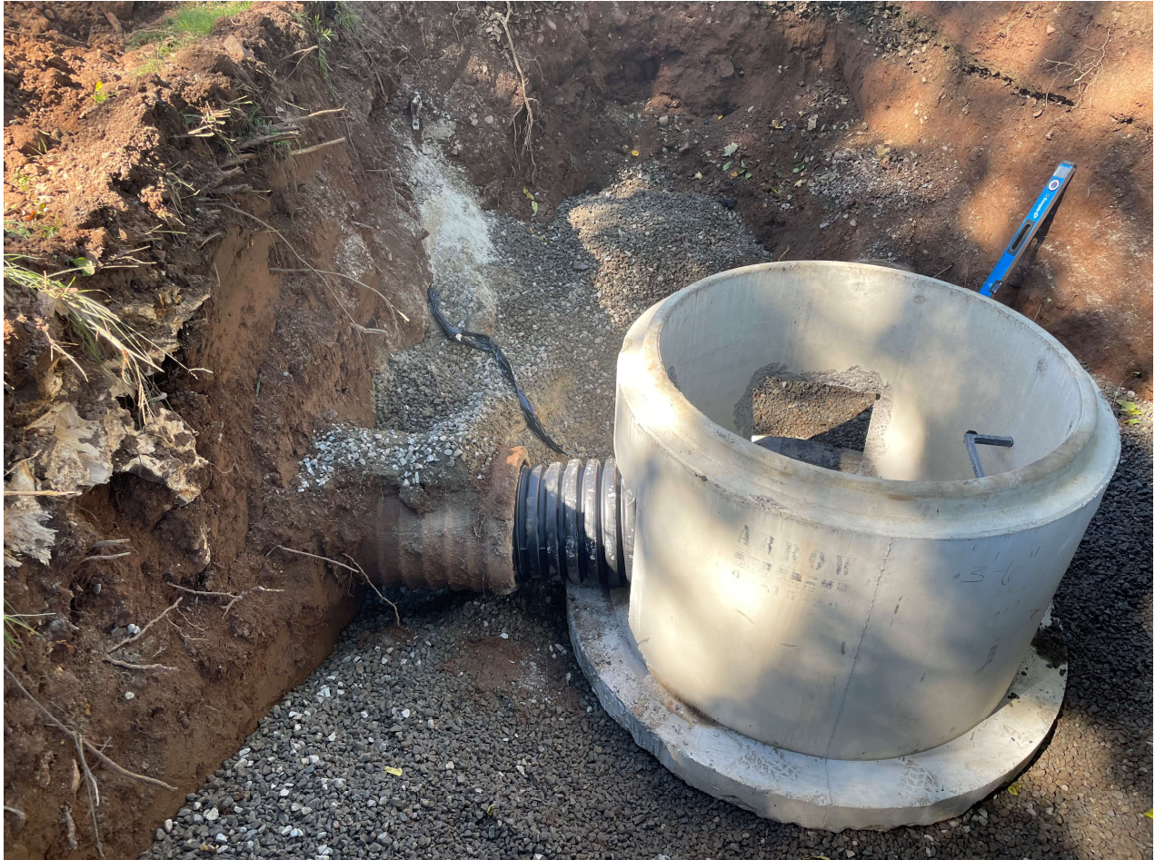
Picture 7: The base of the manhole that Ludlow placed into the excavation they made at the northeast corner of the 177R Main Street property. Ludlow has begun to connect the manhole to a section of existing 15" RCP located on the southwest side of the manhole with 15" black corrugated CPEP. View to the northwest.
