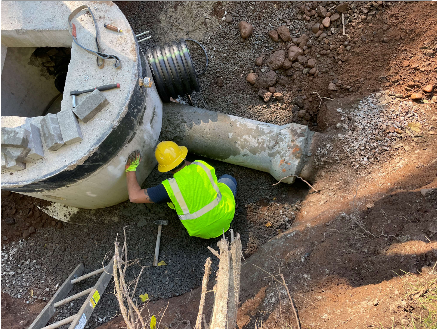
Picture 10: Ludlow placing brick and cement on the north side of the manhole they installed on the northwest corner of the 177R Main Street, Durham, property to secure a new section of 15" RCP that connects to existing 15" RCP coming into the excavation from the northeast. View to the northwest.
