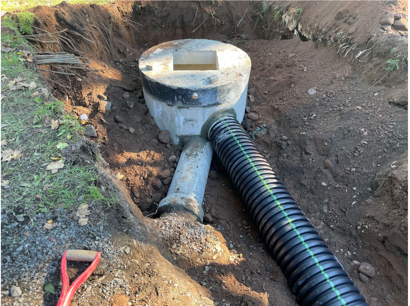
Picture 12: View of the 15" RCP and CPEP that Ludlow secured with brick and cement on the north side of the manhole they installed on the 177R Main Street property. View to the south.
