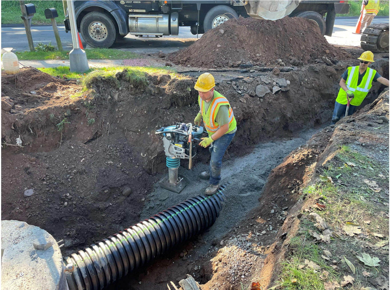
Picture 13: Ludlow using a jumping jack to compact the sand they are placing around the 15" CPEP they installed between the manhole on the 177R Main Street property and the catch basin they installed on the southeast corner of Pickett Lane and Main Street, Durham. View to the northwest.
