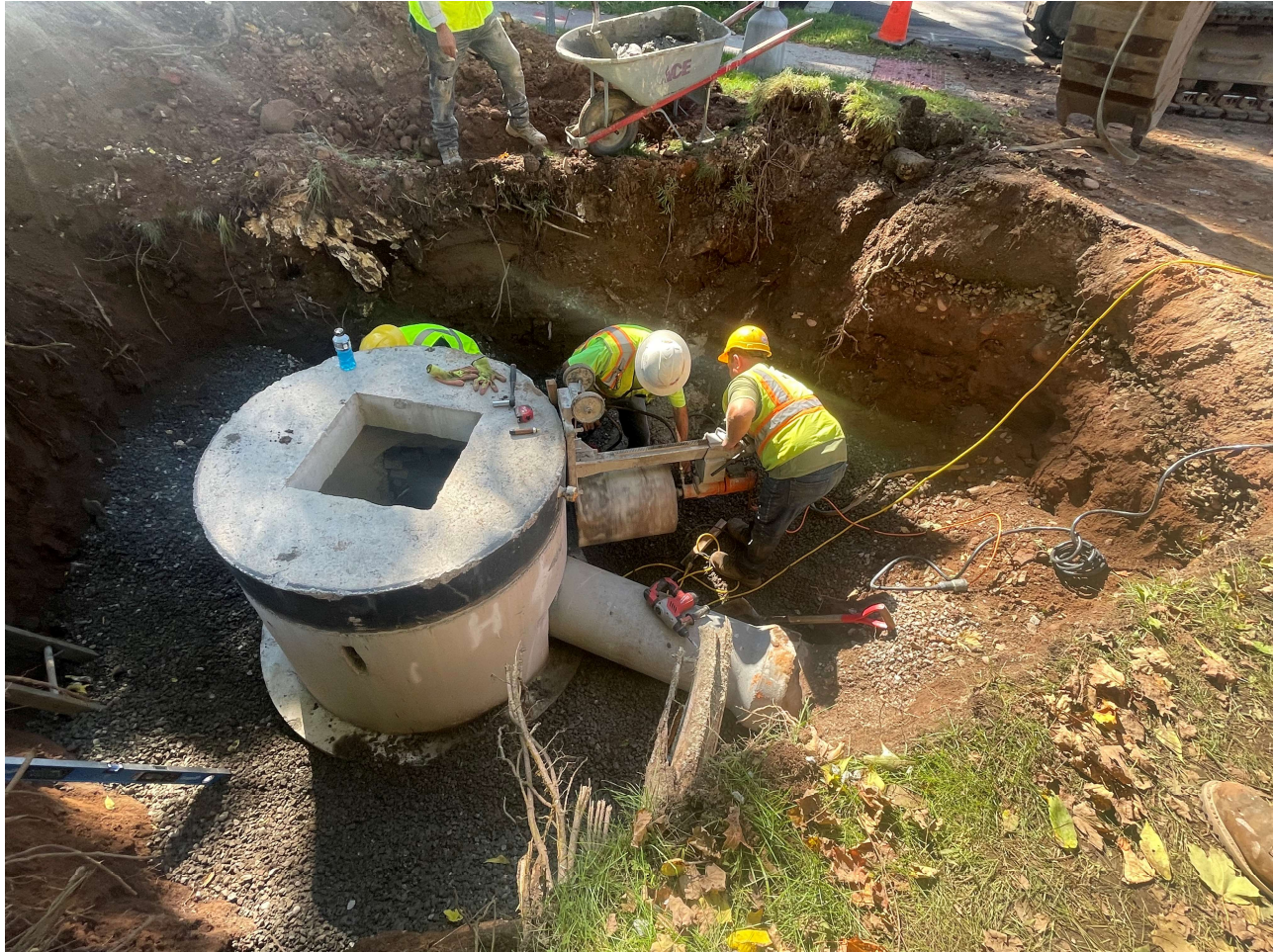
Picture 9: Ludlow coring a hole into the north side of the manhole they just installed on the northwest corner of the 177R Main Street, Durham, property. View to the northwest.
