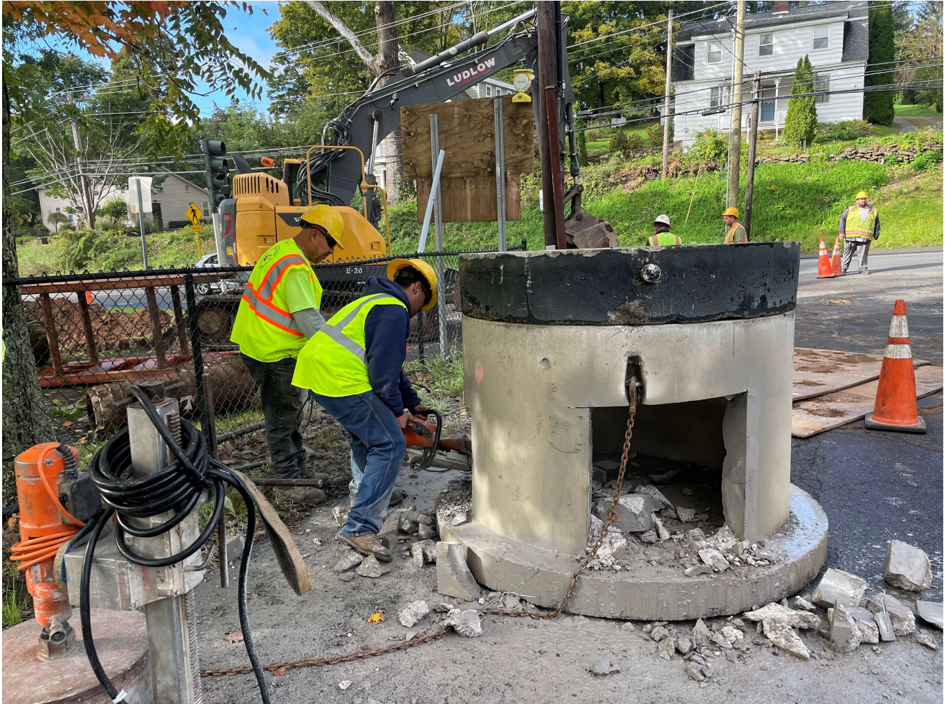
Picture 3: Ludlow using a cutoff saw to enlarge the openings in the side of the catch basin they plan to install on the northwest corner of the 177R Main Street property.
