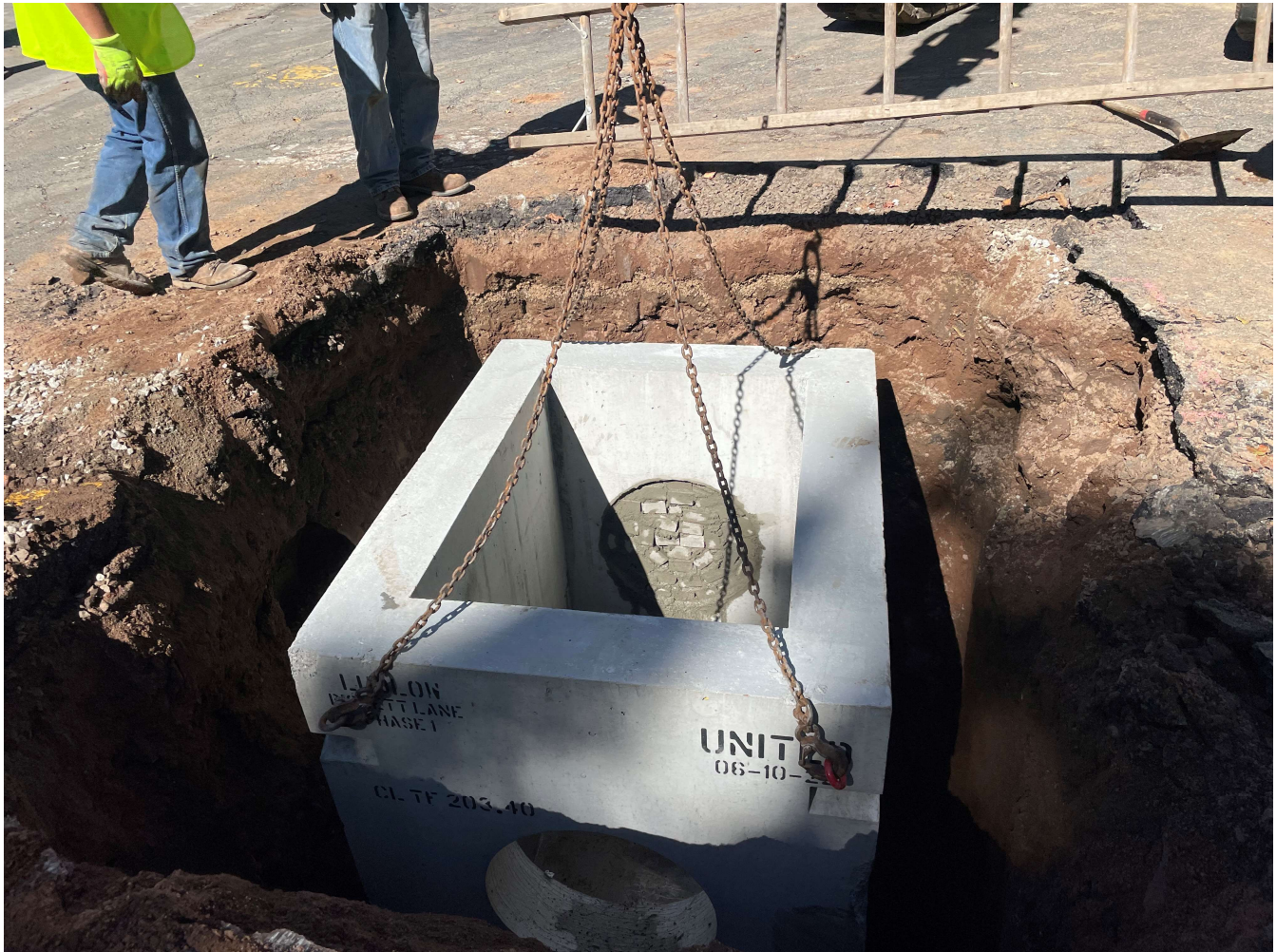
Picture 6: Ludlow setting the base of a catch basin at the southeast corner of the intersection of Pickett Lane and Main Street in Durham. View to the north.
