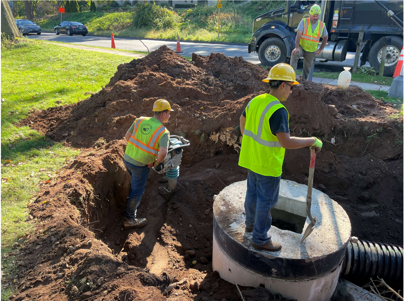
Picture 14: Ludlow compacting backfill they placed around the manhole they installed today on the northwest corner of the 177R Main Street, Durham, property. View to the west.
