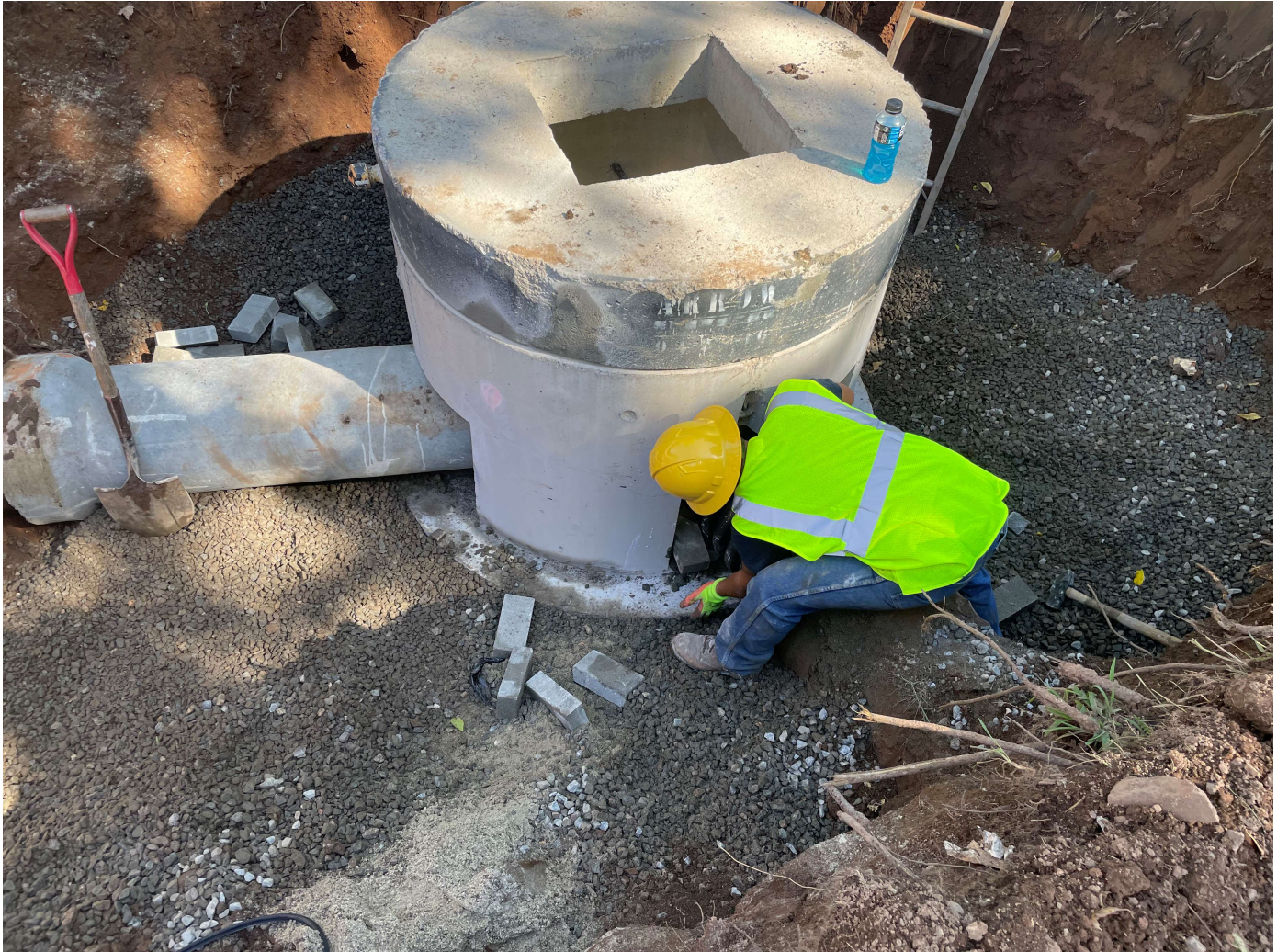
Picture 8: Ludlow placing brick and cement around the section 15" black corrugated CPEP they just installed on the southwest side of the manhole they just placed at the northwest corner of the 177R Main Street property. View to the southeast.
