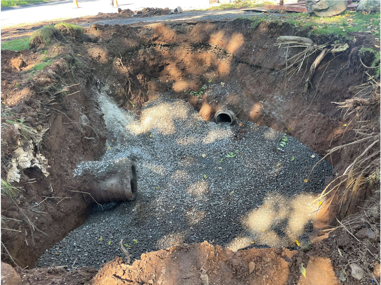
Picture 5: The excavation that Ludlow made on the northwest corner of the 177R Main Street property where they have daylighted two existing sections of 15" RCP. Ludlow has also placed ¾" stone on the bottom of the excavation. View to the northwest.
