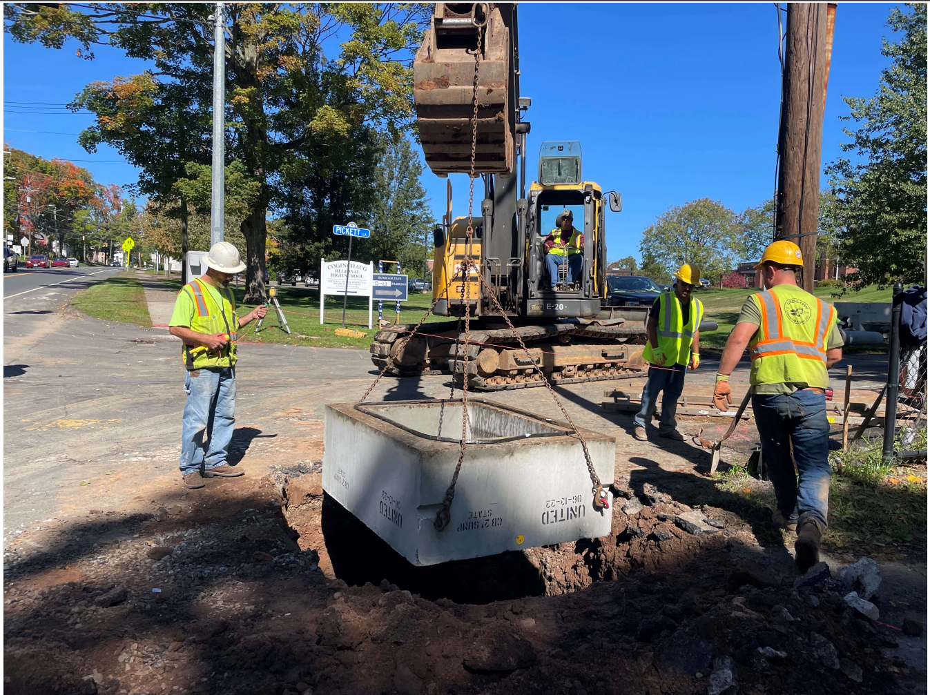
Picture 4: Ludlow setting the base of a catch basin into the excavation they made on the southeast corner of the intersection of Pickett Lane and Main Street, Durham. View to the north.
