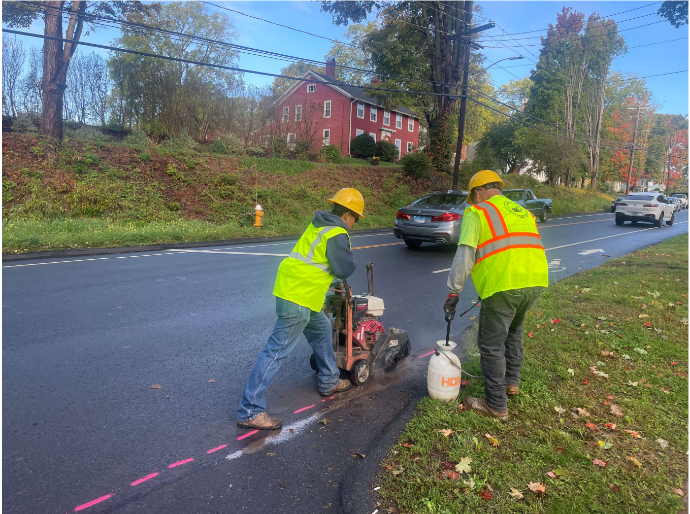
Picture 1: Ludlow saw cutting the pavement where Pickett Lane intersects with Main Street in Durham in preparation of upcoming road repair/repaving activities on Pickett Lane. View to the northwest.
