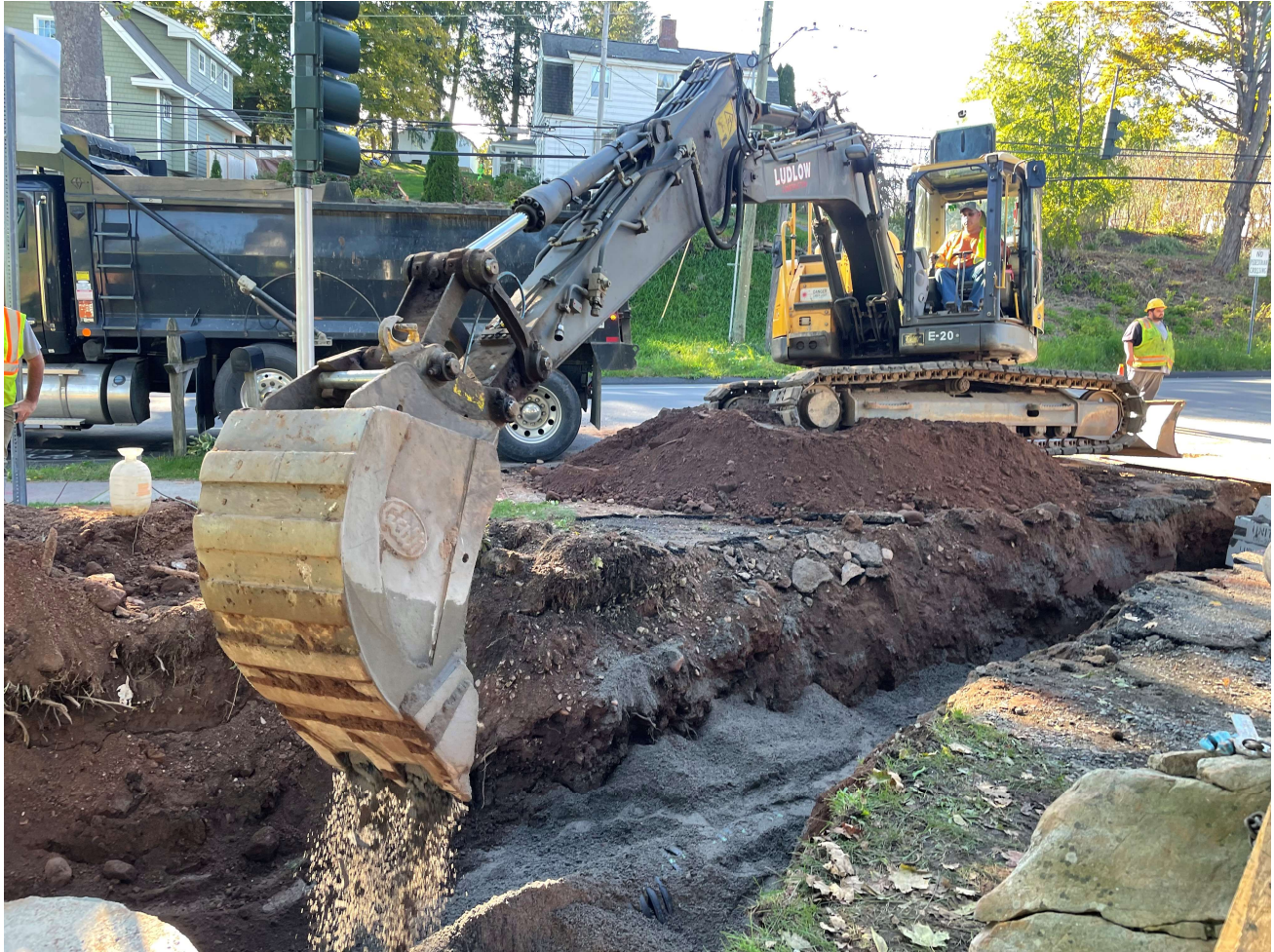
Picture 15: Ludlow placing sand over the 15" CPEP they installed between the manhole on the 177R Main Street property and the catch basin they installed on the southeast corner of Pickett Lane and Main Street, Durham. View to the northwest.
