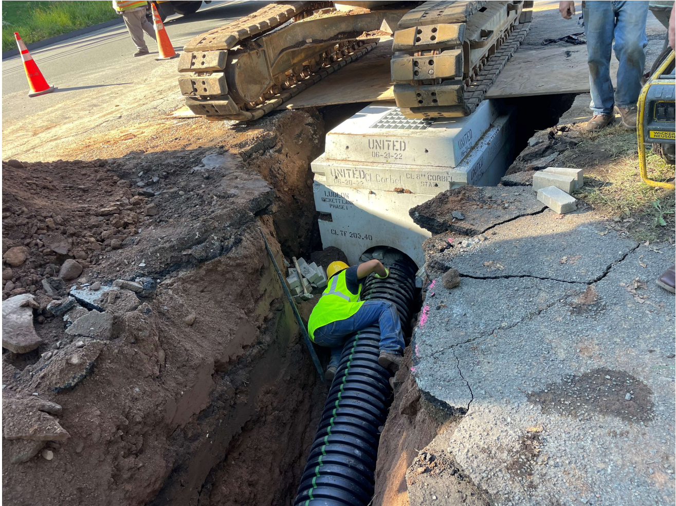
Picture 11: Ludlow placing brick and cement around 15" CPEP that they ran from the manhole they installed on the 177R Main Street property to the catch basin they installed on the southeast corner of the intersection of Pickett Lane and Main Street. View to the north.
