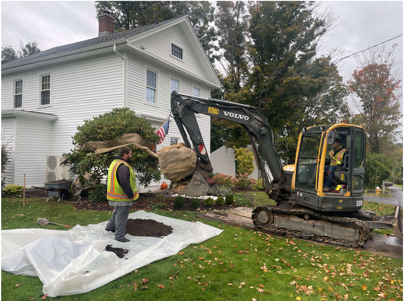
Picture 2: Ludlow moving a shrub from the 24 Maiden Lane property as they prepare to daylight the southwest corner of the home's foundation. View to the northeast.
