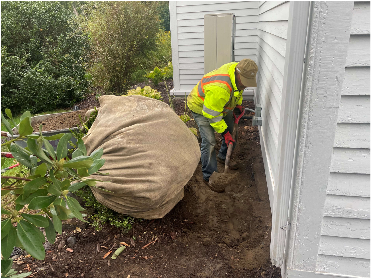
Picture 3: Ludlow hand-excavating around the southwest corner of the 24 Maiden Lane, Durham, residence. View to the north.
