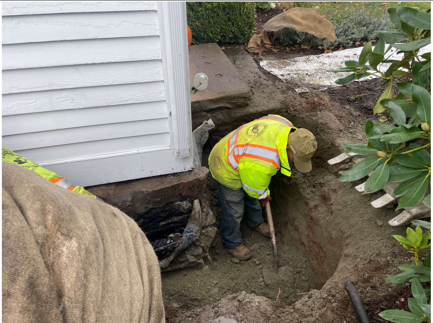
Picture 4: Ludlow hand-excavating around the southwest corner of the 24 Maiden Lane, Durham, residence. View to the east.
