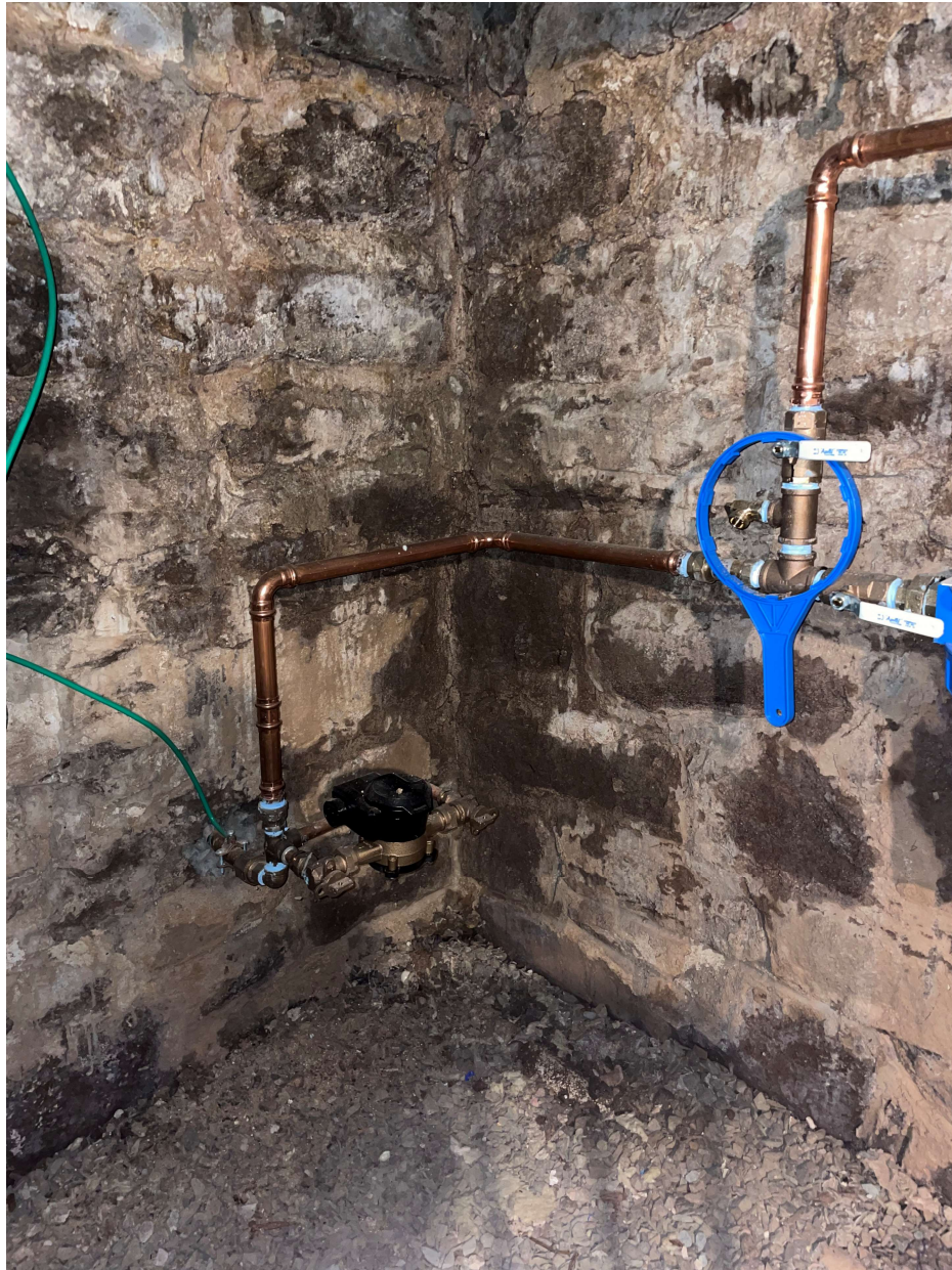
Picture 1: Southwest corner of the 24 Maiden Lane foundation. View to the southeast.
