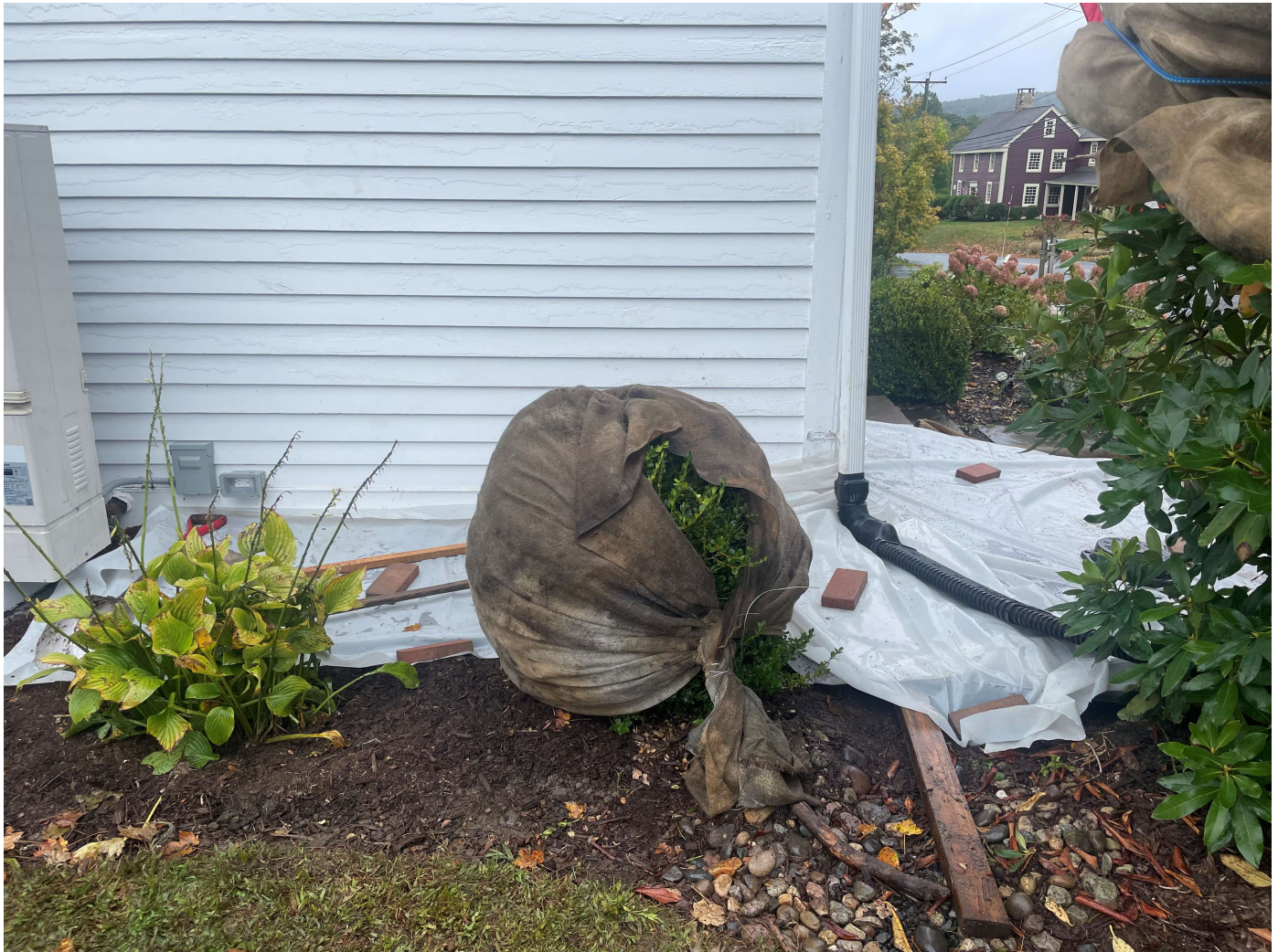
Picture 5: The southwest corner of the 24 Maiden Lane residence after Ludlow covered the open excavation with plywood and poly sheeting. View to the east
