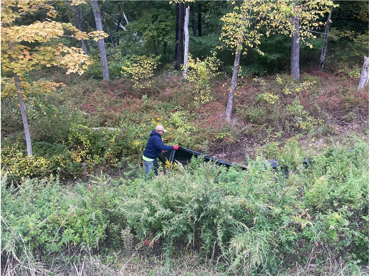
Picture 1: Ludlow removing silt fence from the north side of the Shared Access Road in Middletown at Station ~14+00. View to the northeast.
