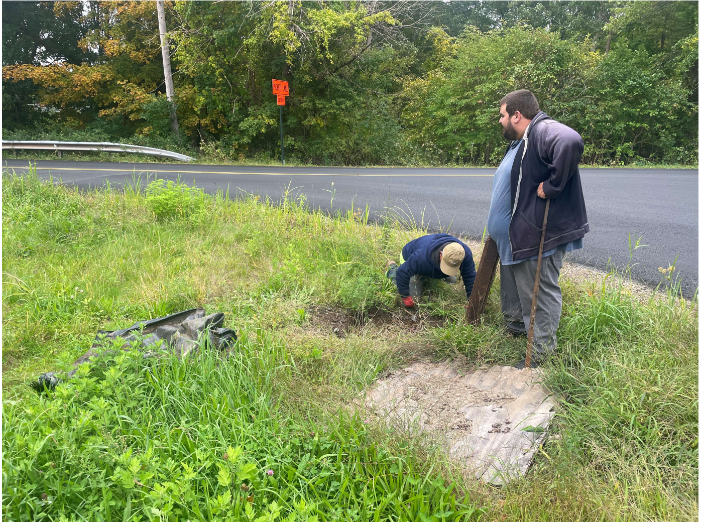
Picture 2: Ludlow is removing filter fabric from a catch basin located at the east side of where Brick Lane intersects Maiden Lane. View to the southeast.
