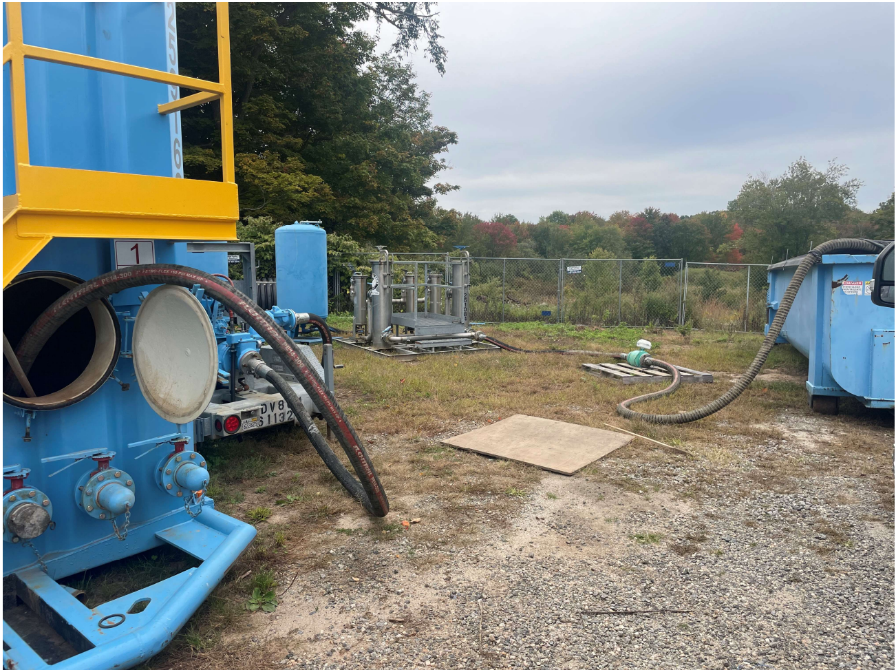
Picture 3: Ludlow running groundwater that was collected during well assessment and well decommissioning activities through a treatment system staged at the 281 Main Street, Durham work yard. Treated groundwater is being stored in the rolloff container located on the right side of the photograph.
