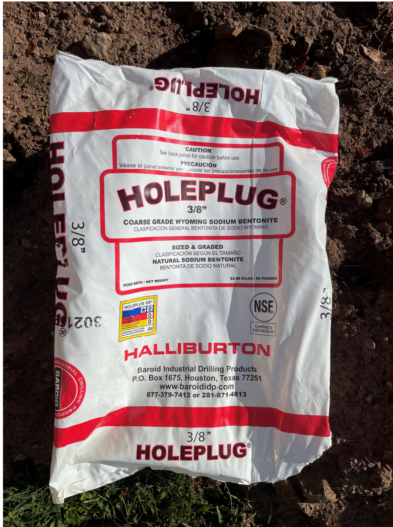
Picture 3: The brand of bentonite chips that Grela is placing into the well located on the north side of the CRHS as part of well decommissioning activities.
