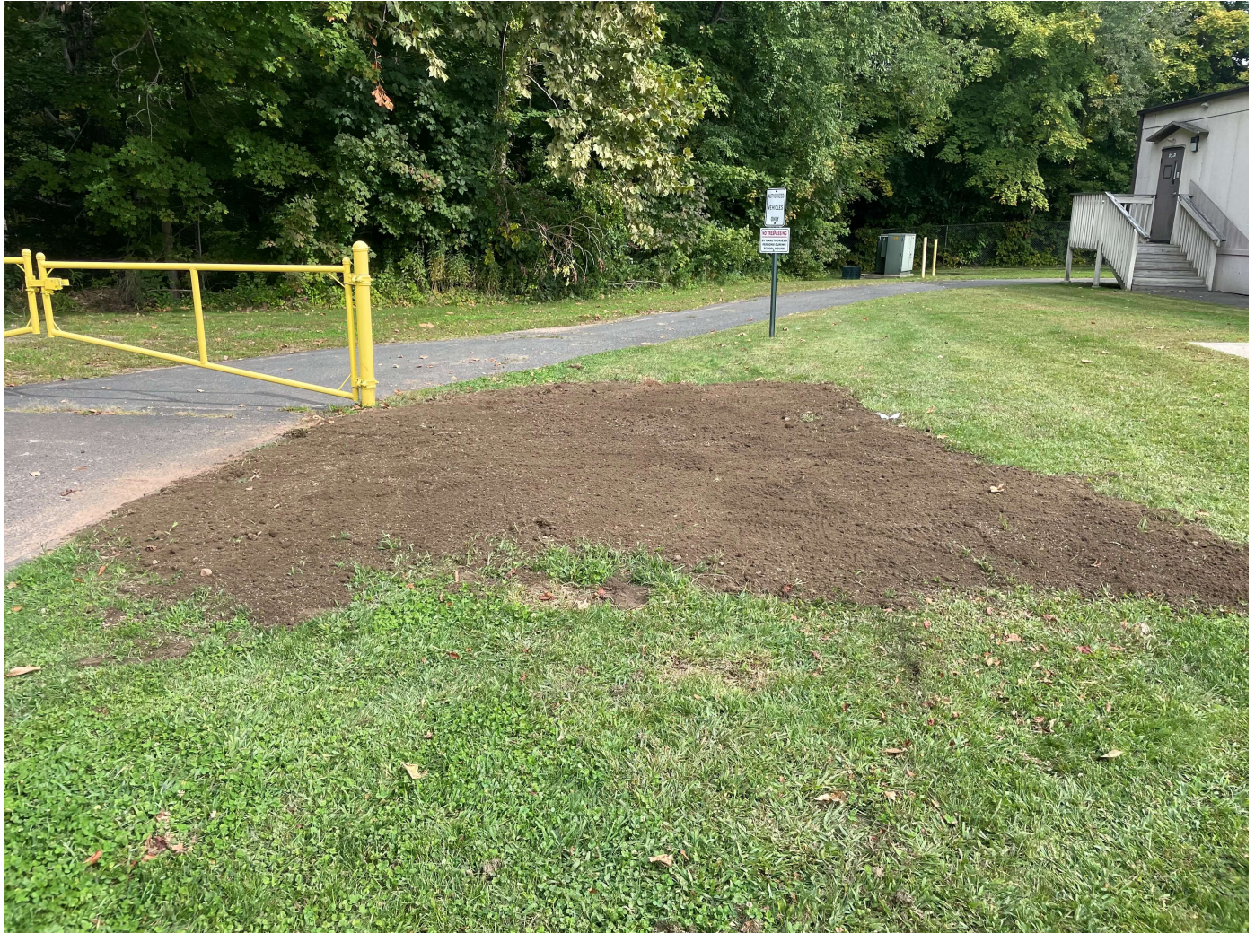
Picture 8: The area located on the north side of the CRHS after Ludlow placed loam and grass seed after Grela decommissioned a well. View to the east.
