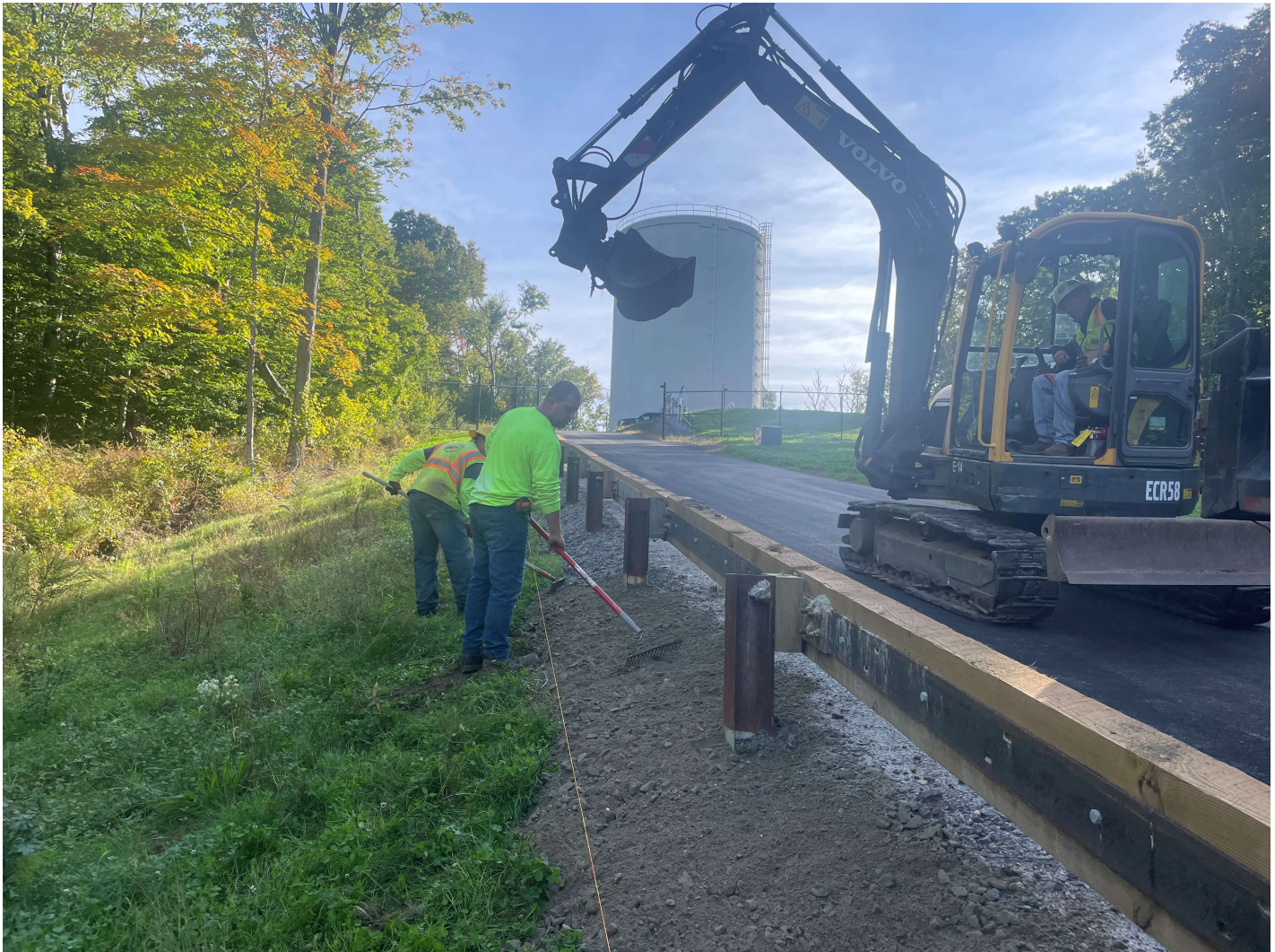
Picture 1: Ludlow placing 1.25" processed gravel on the north side of the guard rail located on the north side of the Shared Access Road in Middletown. View to the east.
