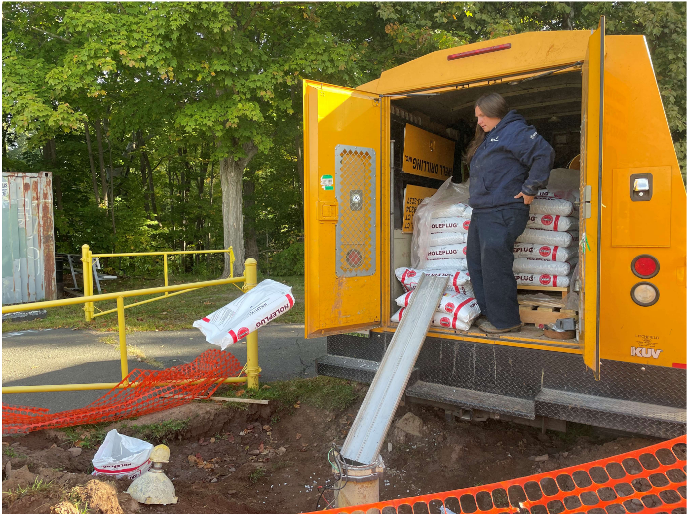
Picture 2: Grela set up to continue placing bentonite chips into the well located on the north side of the CRHS as part of well decommissioning activities. View to the northeast.
