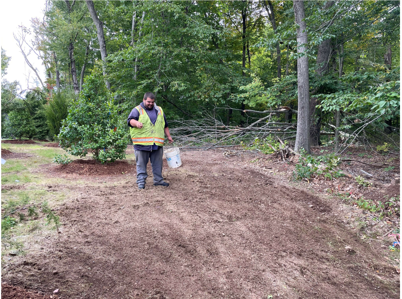
Picture 5: Ludlow spreading grass seed around the trees that were recently planted on the south side of the water tank located east of the Shared Access Road in Middletown. View to the east
