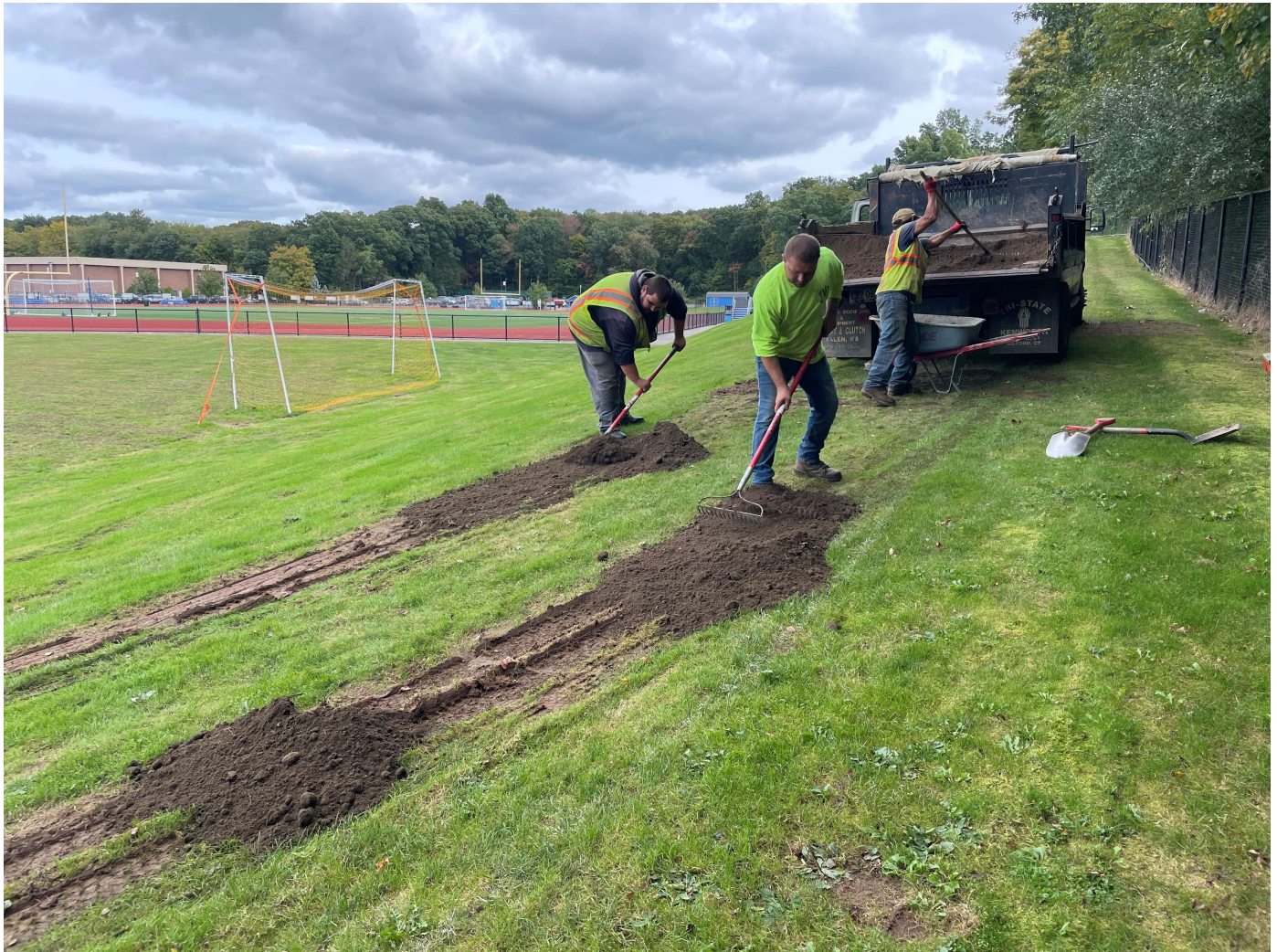
Picture 7: Ludlow raking out loam that they placed on the west side of the CRHS soccer field to repair the areas that were damaged when Grela Drilling decommissioned a well. View to the east.
