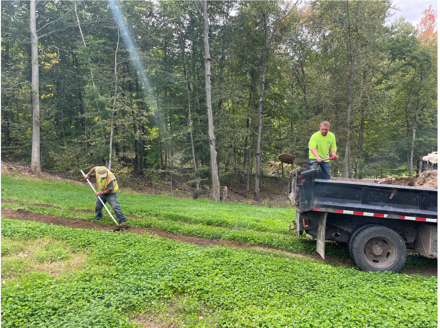
Picture 6: Ludlow raking out loam that they placed on the south side of the Shared Access Road in Middletown to repair the areas that were damaged when Jays Landscaping planted trees on the south side of the water tank. View to the south.
