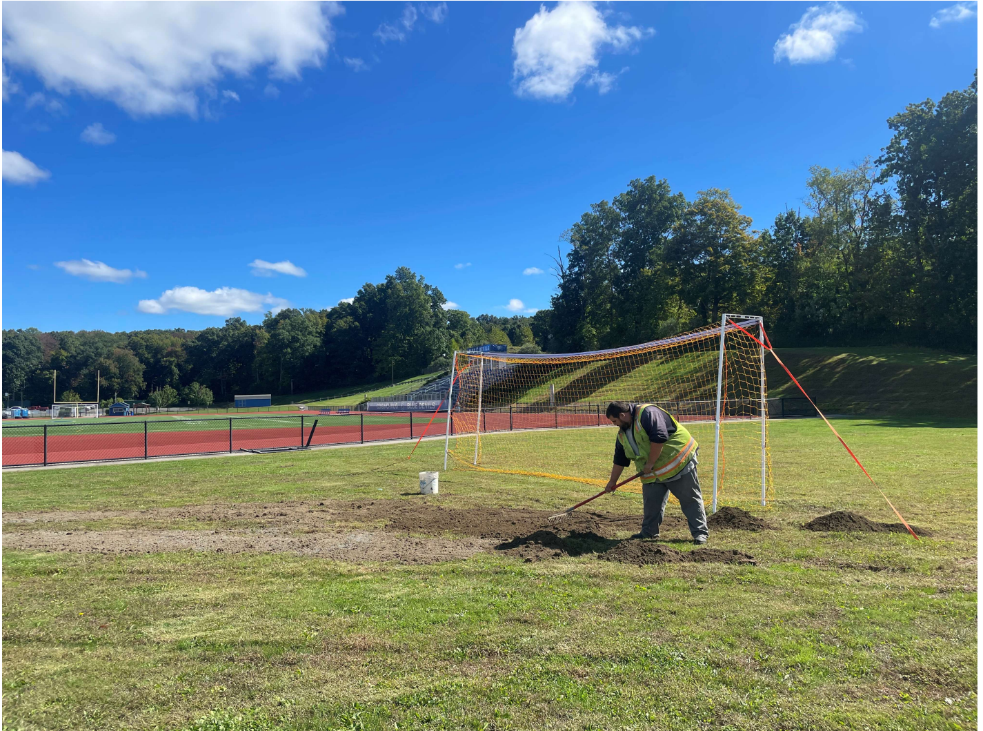
Picture 6: Ludlow raking out loam that they placed on the west side of the CRHS soccer field to repair those sections of the field that were disturbed during the decommissioning of a well by Grela. View to the southeast.
