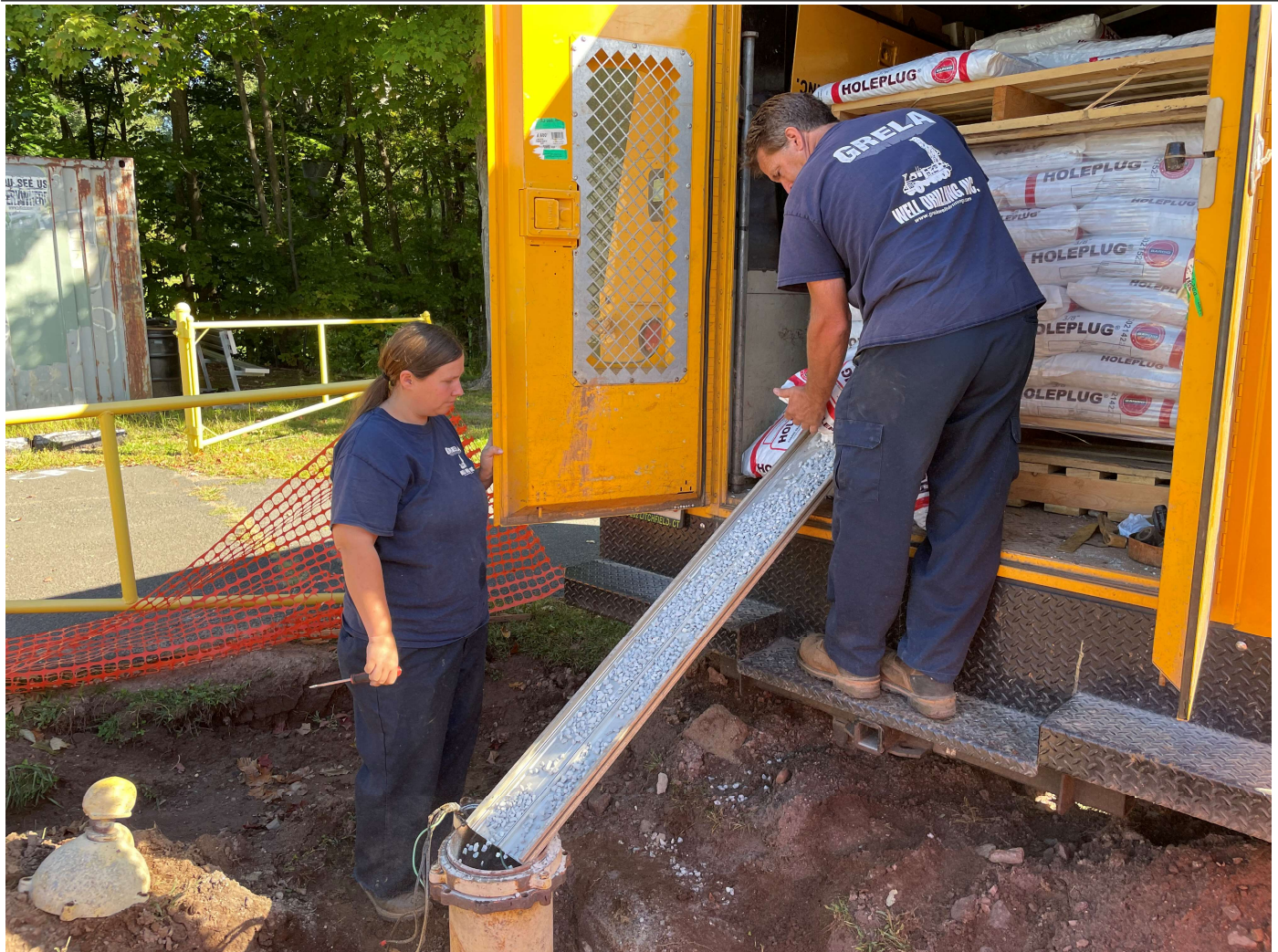
Picture 5: Grela placing bentonite chips into the well located on the north side of the CRHS. View to the northeast.
