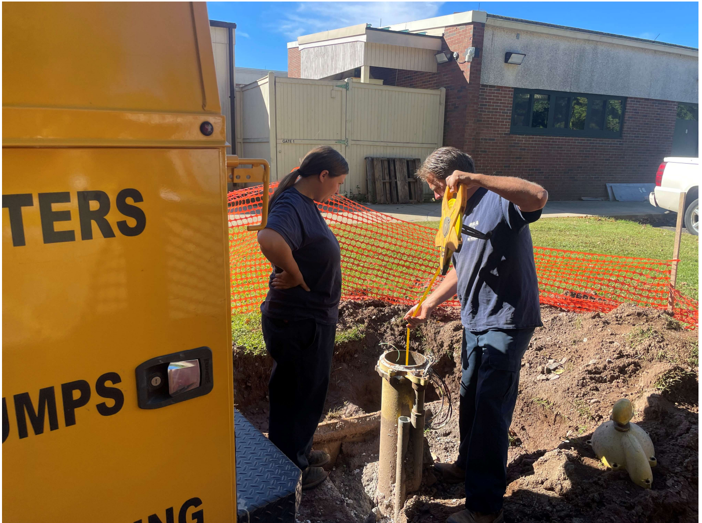
Picture 4: Grela measuring the depth to the top of the bentonite chips they placed in the well located on the north side of the CRHS yesterday before placing additional chips into the well. View to the southwest.
