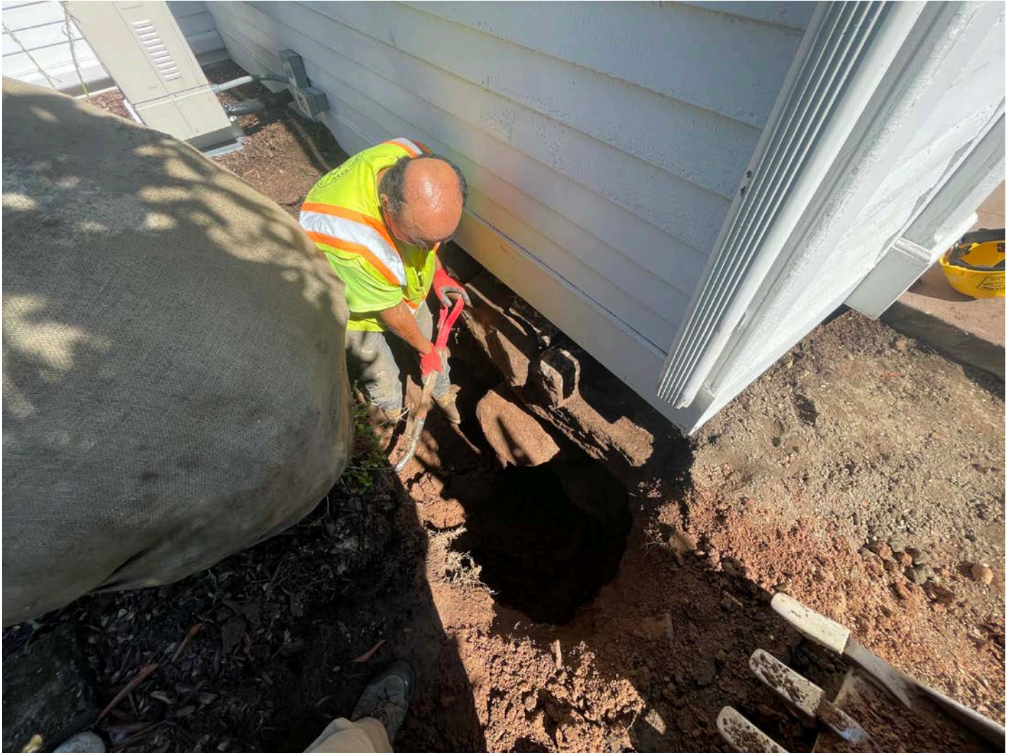
Picture 3: Ludlow hand-excavating at the southwest corner of the 24 Maiden Lane, Durham, residence as they work to address a leak in the home's foundation. View to the northeast.
