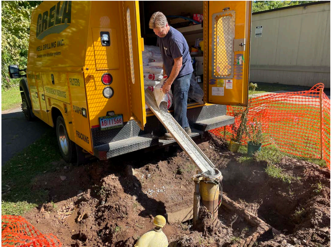
Picture 4: Grela placing bentonite chips into the well located on the north side of the Cuginchaug Regional High School as part of well decommissioning activities. View to the northwest.
