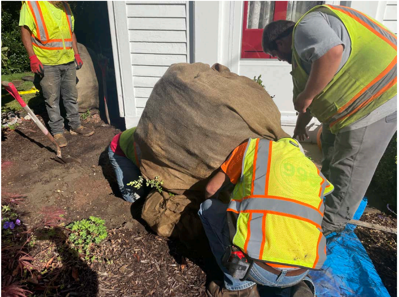
Picture 2: Ludlow wrapping burlap around a shrub they removed from the southwest corner of the 24 Maiden Lane, Durham, residence as they prepare to excavate to address a leak in the home's foundation. View to the northwest.
