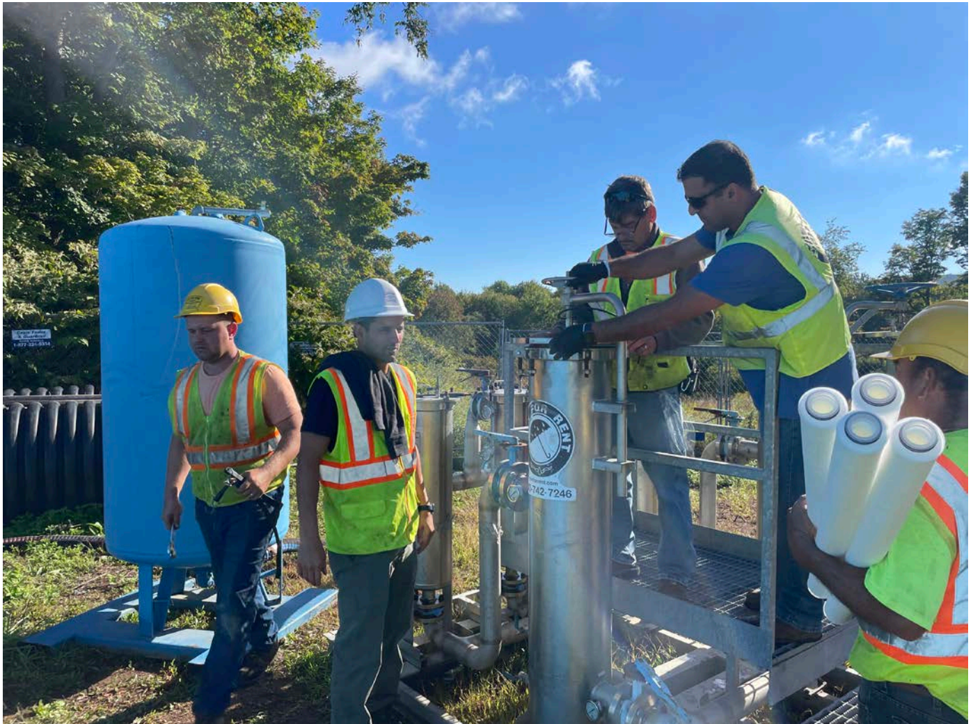
Picture 2: Rain for Rent assisting Ludlow in setting up the treatment system that will be used to treat water in the frak tank located at the 281 Main Street, Durham, work yard. View to the northeast.
