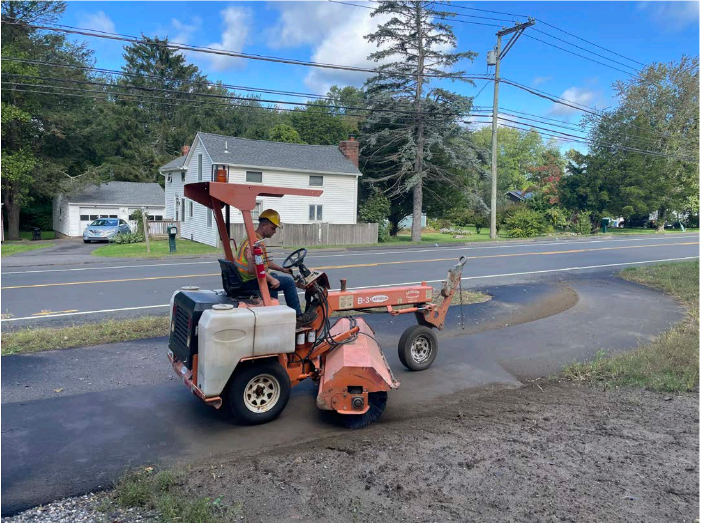
Picture 4: Ludlow using a Broce Broom to clean the driveway of the Water Meter Building located on S. Main Street in Middletown. View to the northwest.
