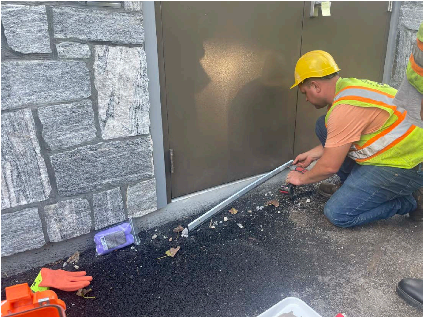
Picture 7: Ludlow attaching a sweep to the bottom of one of the doors to the Water Meter Building located on S. Main Street in Middletown. View to the southeast.
