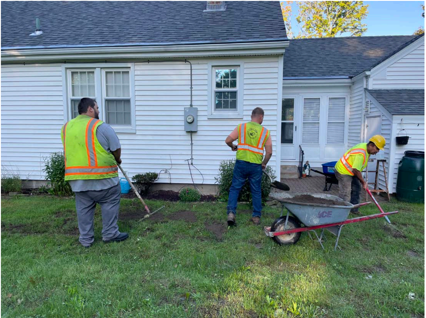
Picture 1: Ludlow placing and grading loam on the east side of the 261 Main Street, Durham, residence. View to the northwest.
