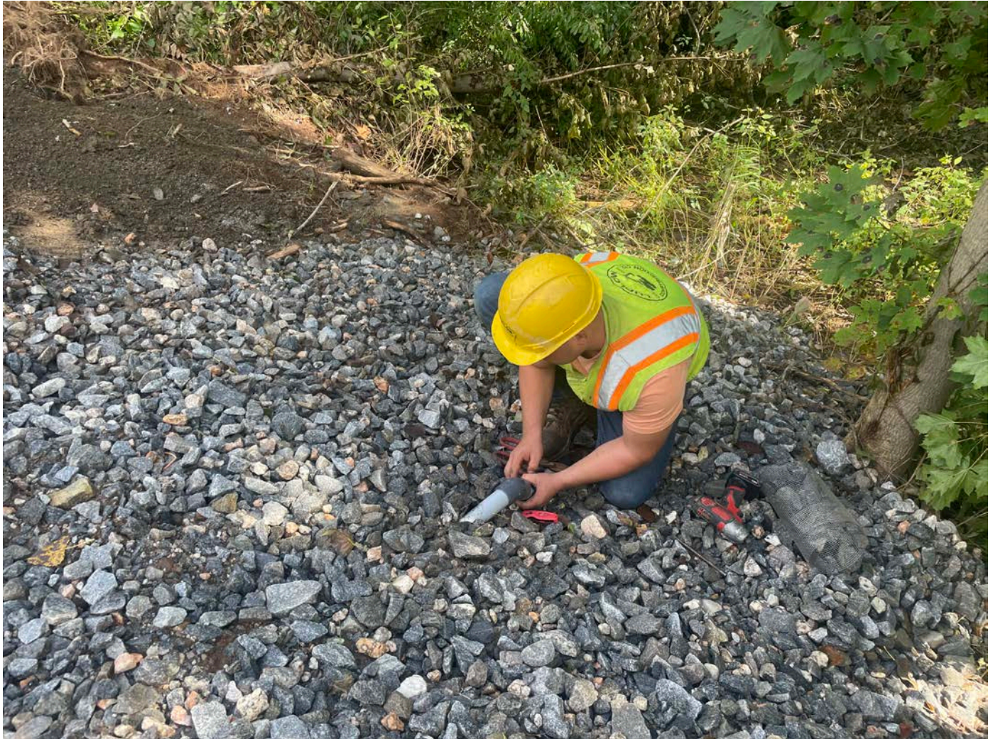
Picture 6: Ludlow attaching a section of screen to the sump pump discharge point located on the east side of the Water Meter Building located on S. Main Street in Middletown. View to the northeast.
