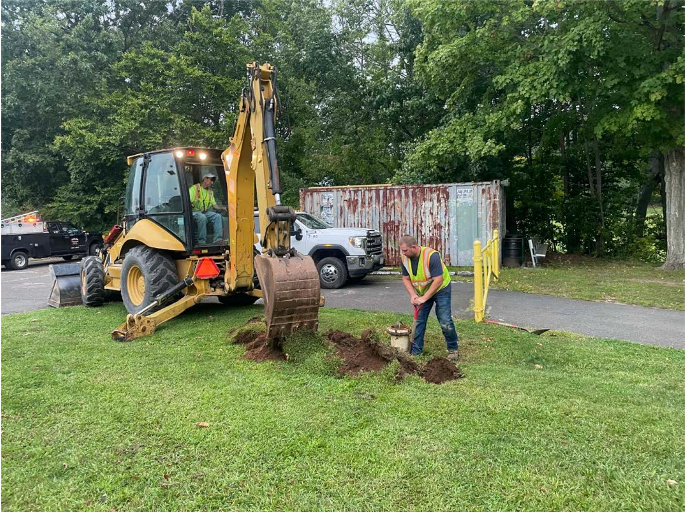
**Picture 1: Ludlow excavating around the well located on the north side of the CRHS as part of well decommissioning activities. View to the northwest.**
