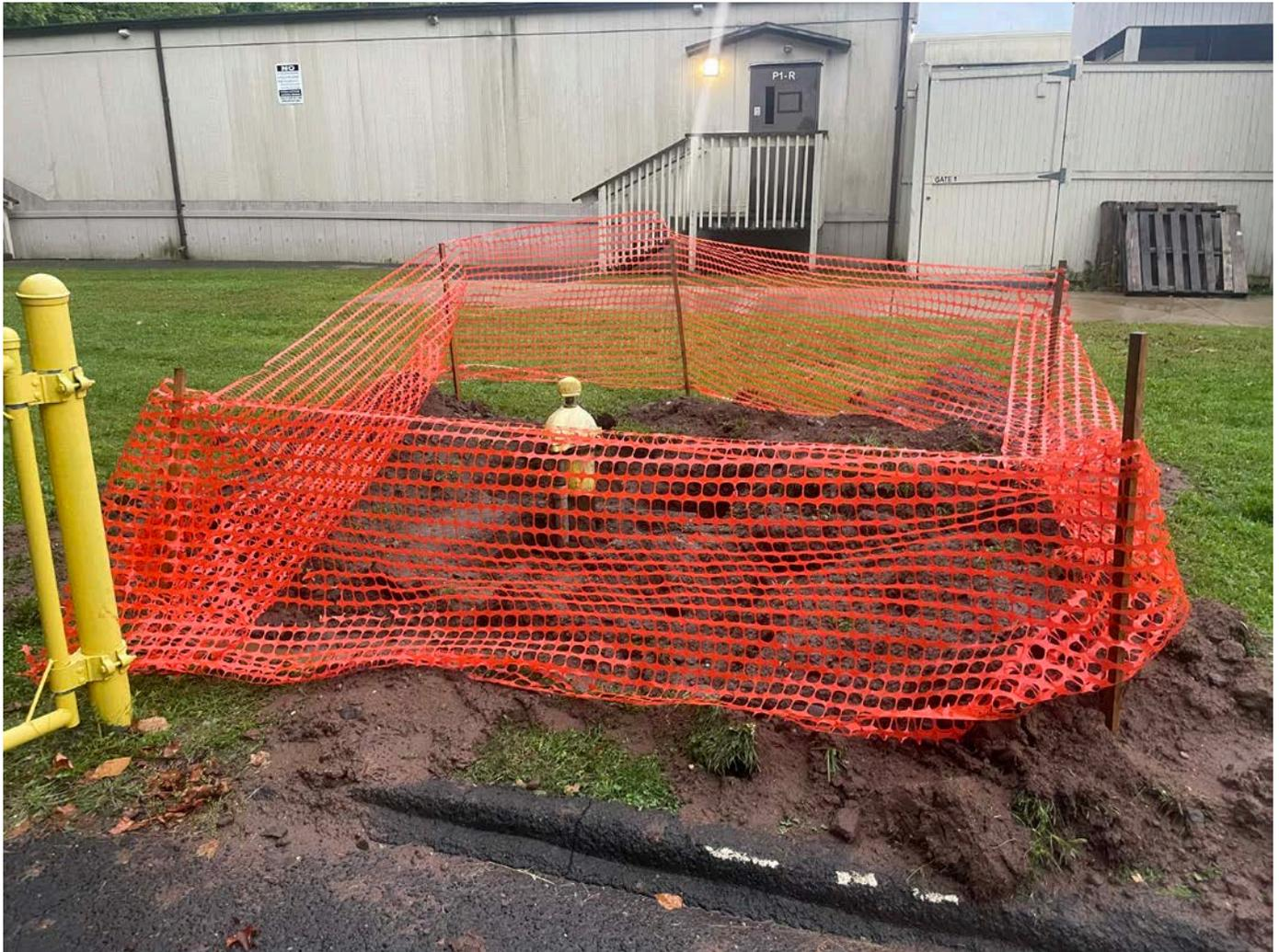
Picture 2: The excavation that Ludlow made and then secured with snow fencing on the north side of the CRHS as part of well decommissioning activities. View to the south.
