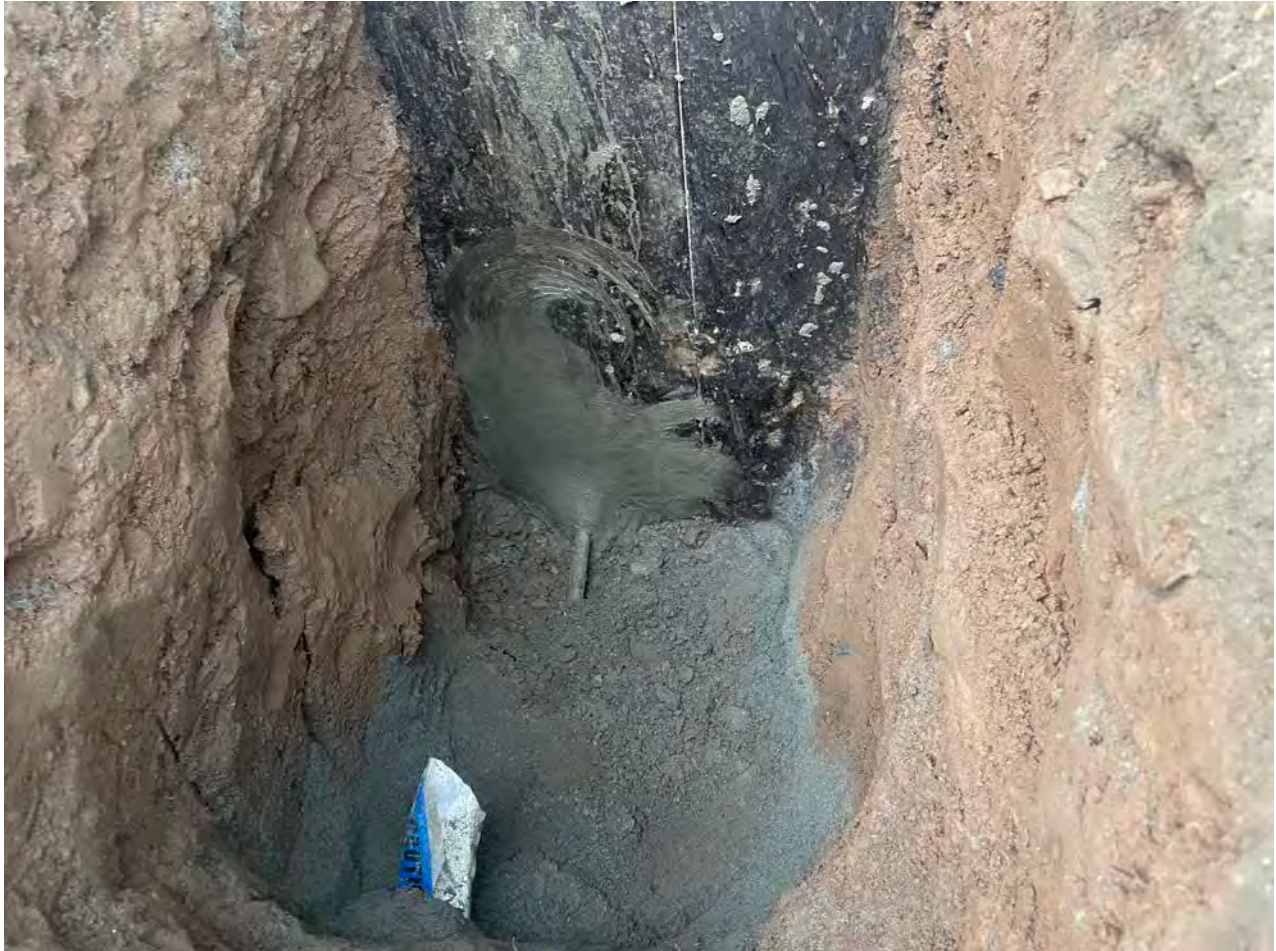
Picture 3: The east side of the 166 Maple Avenue residence where Ludlow has daylighted the 1” copper water service line that penetrates the home’s foundation. Ludlow has placed a patch of hydraulic cement around the area where the copper line penetrates the foundation. View to the west.
