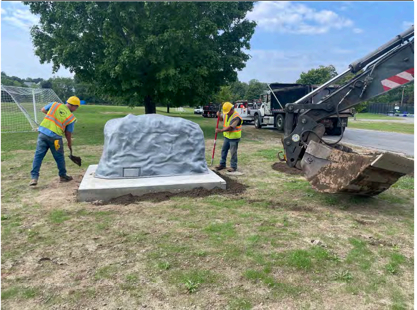
Picture 8: Ludlow placing loam around the backflow preventer located on the south side of Pickett Lane, Durham, near Station 517+73. View to the west.
