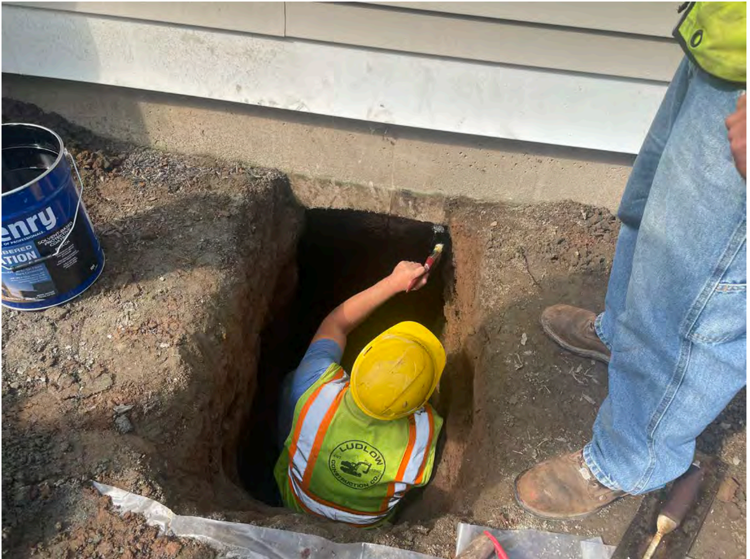
Picture 5: Ludlow applying foundation coating to the area they placed a cement patch at the 166 Maple Avenue residence where the 1" copper water service line penetrates the foundation. View to the west.
