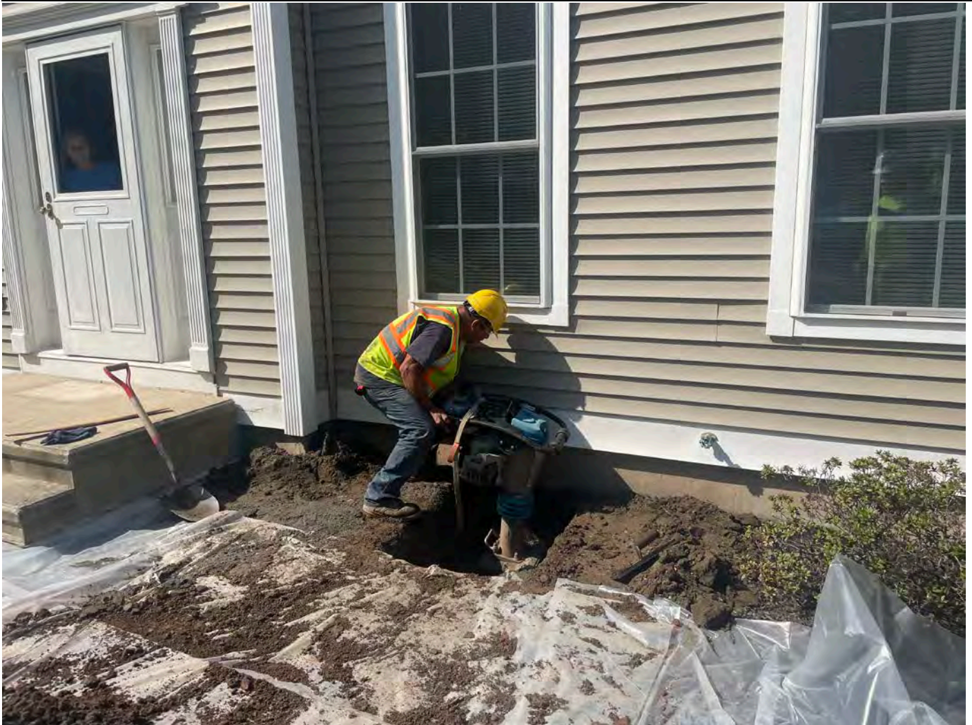
Picture 6: Ludlow compacting backfill on the east side of the 166 Maple Avenue residence after they repaired a small leak where the 1" copper water service line penetrates the east side of the home's foundation. View to the southwest.
