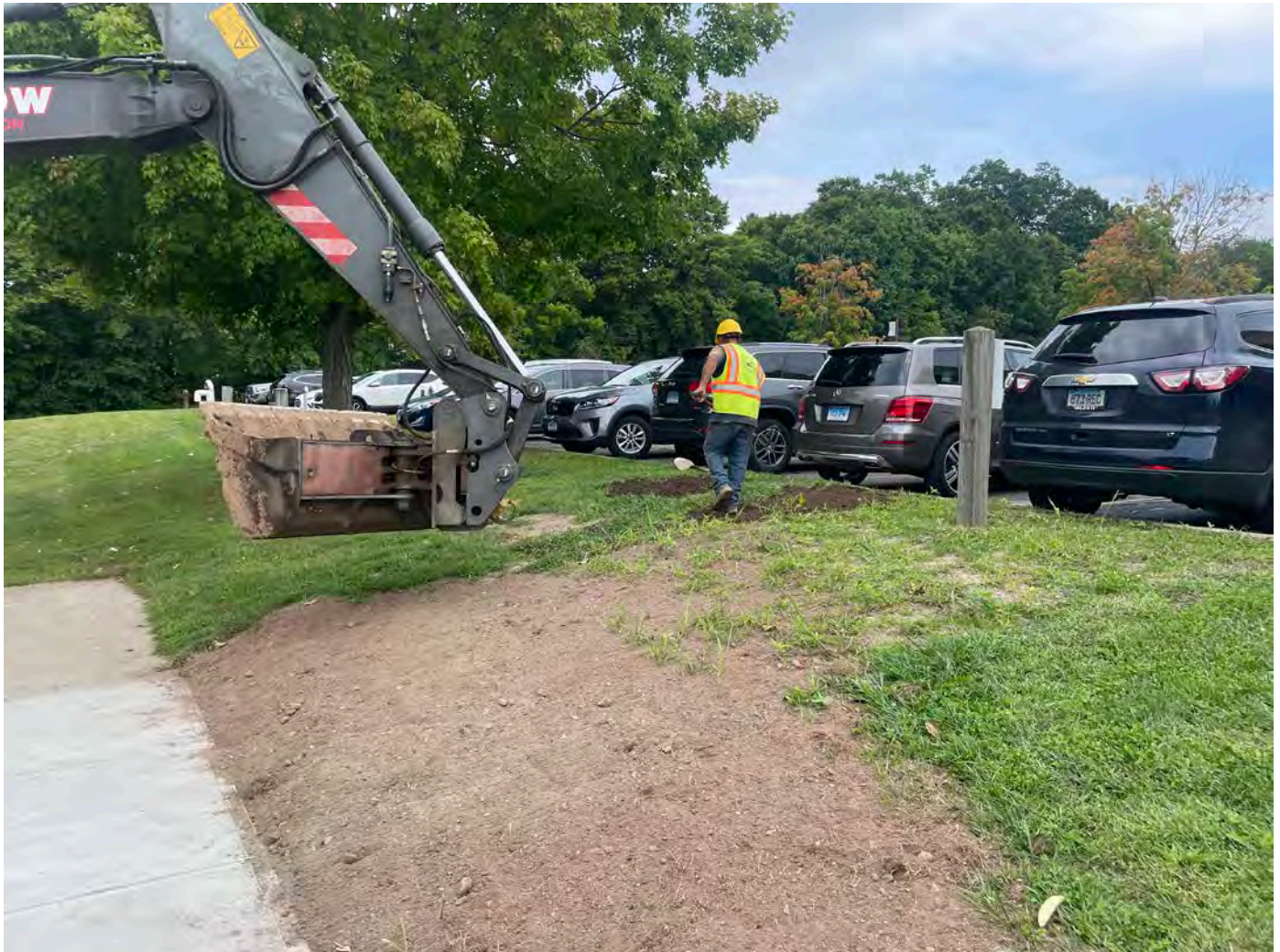
Picture 7: Ludlow placing loam on the portions of the lawn that were disturbed during the installation of a water service line at the CRHS. View to the northeast.
