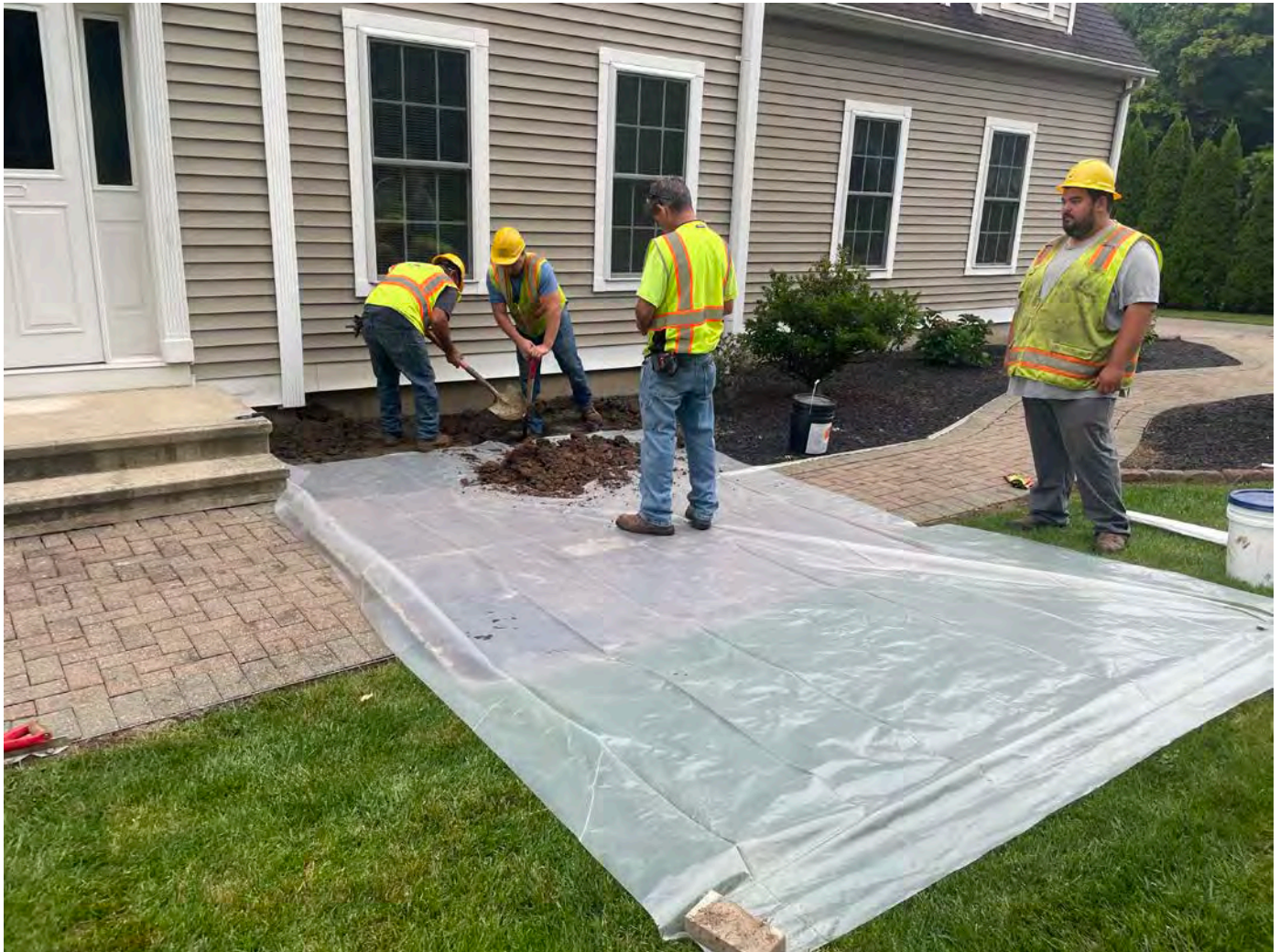
Picture 2: Ludlow hand-excavating on the east side of the 166 Maple Avenue residence to daylight where the 1" copper water service line penetrates the foundation in order to address a minor leak in the basement of the house. View to the northwest.
