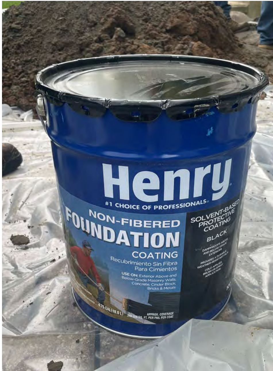
Picture 4: The foundation coating that Ludlow applied to the area they placed a cement patch at the 166 Maple Avenue residence where the 1" copper water service line penetrates the foundation.
